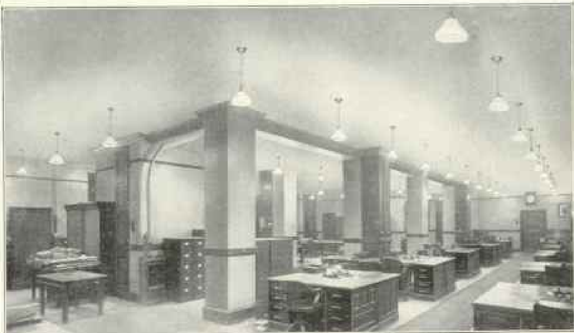
Alba Lighting Equipment, Carnegie Steel Co., Pittsburgh. Desk lamps in this room were removed after installing Alba.
