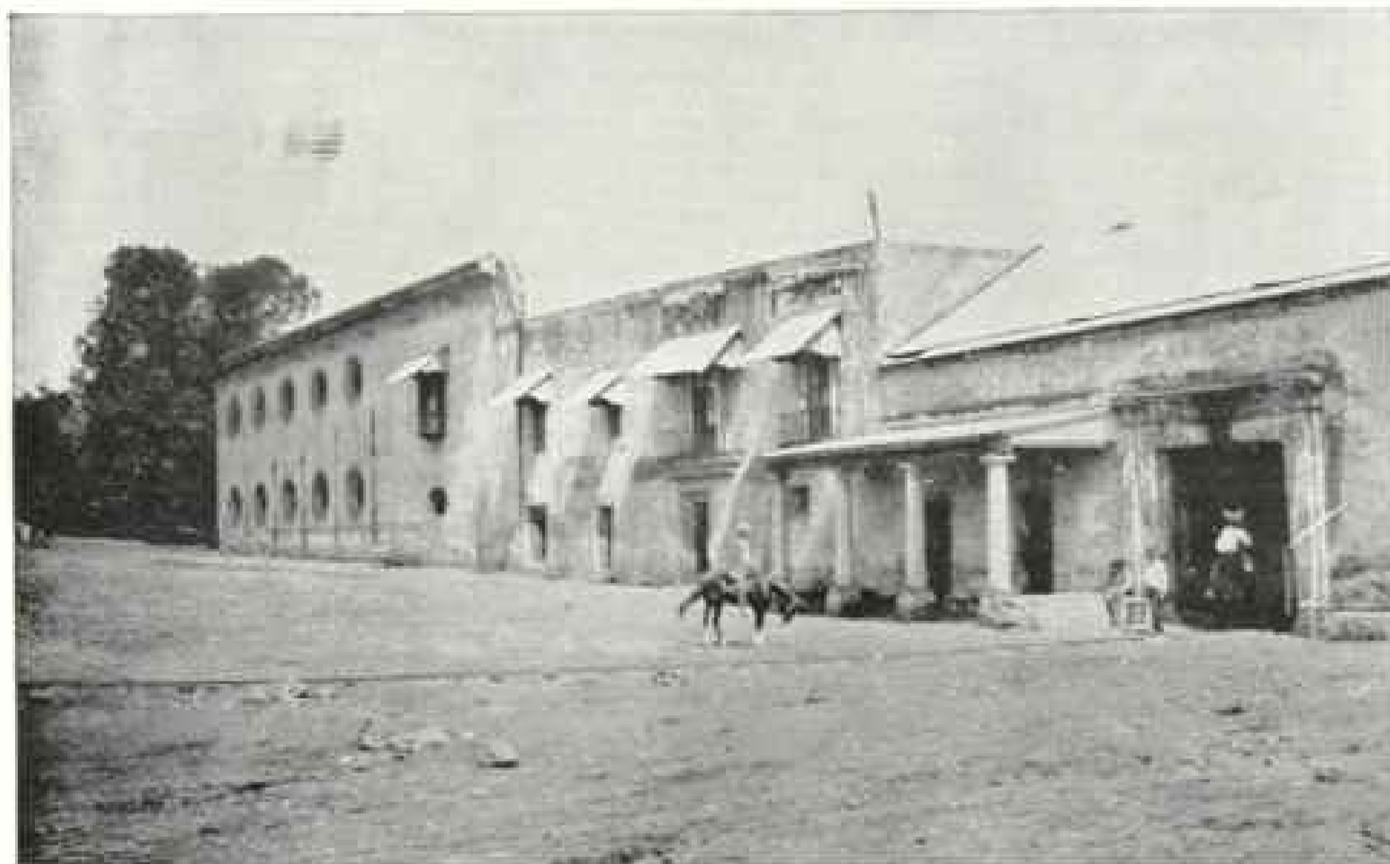
BUILDINGS OF HACIENDA ATLAOMULCO, CUERNAVACA, MEXICO, BUILT BY CORTÉS AND STILL OWNED BY CORTÉS' ESTATE
