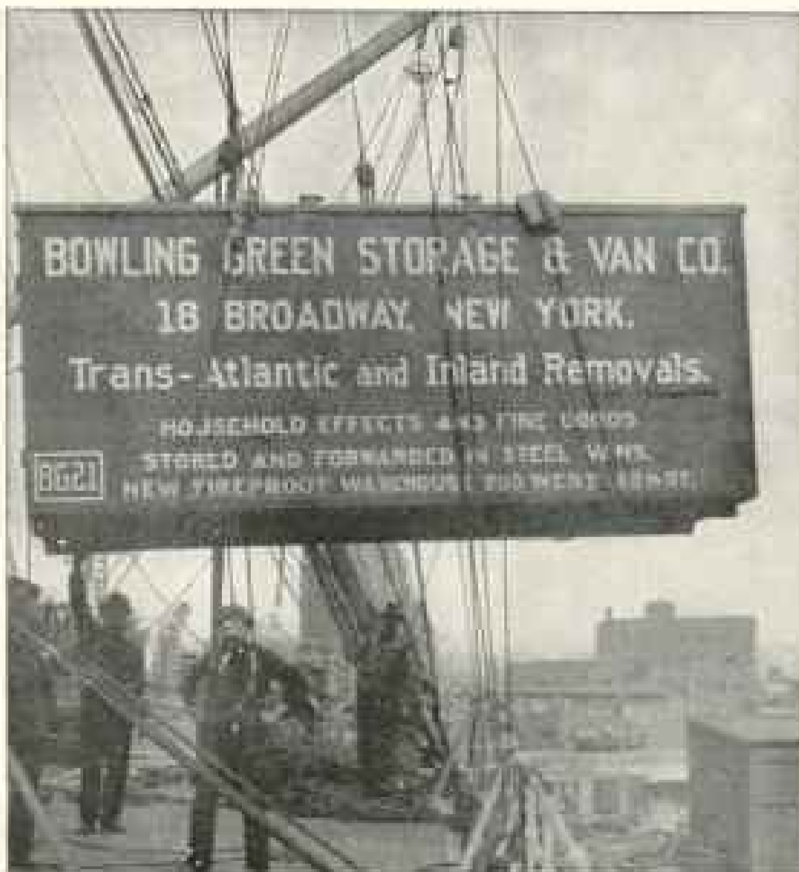
HOISTING LIFT-VAN ON BOARD STEAMSHIP
