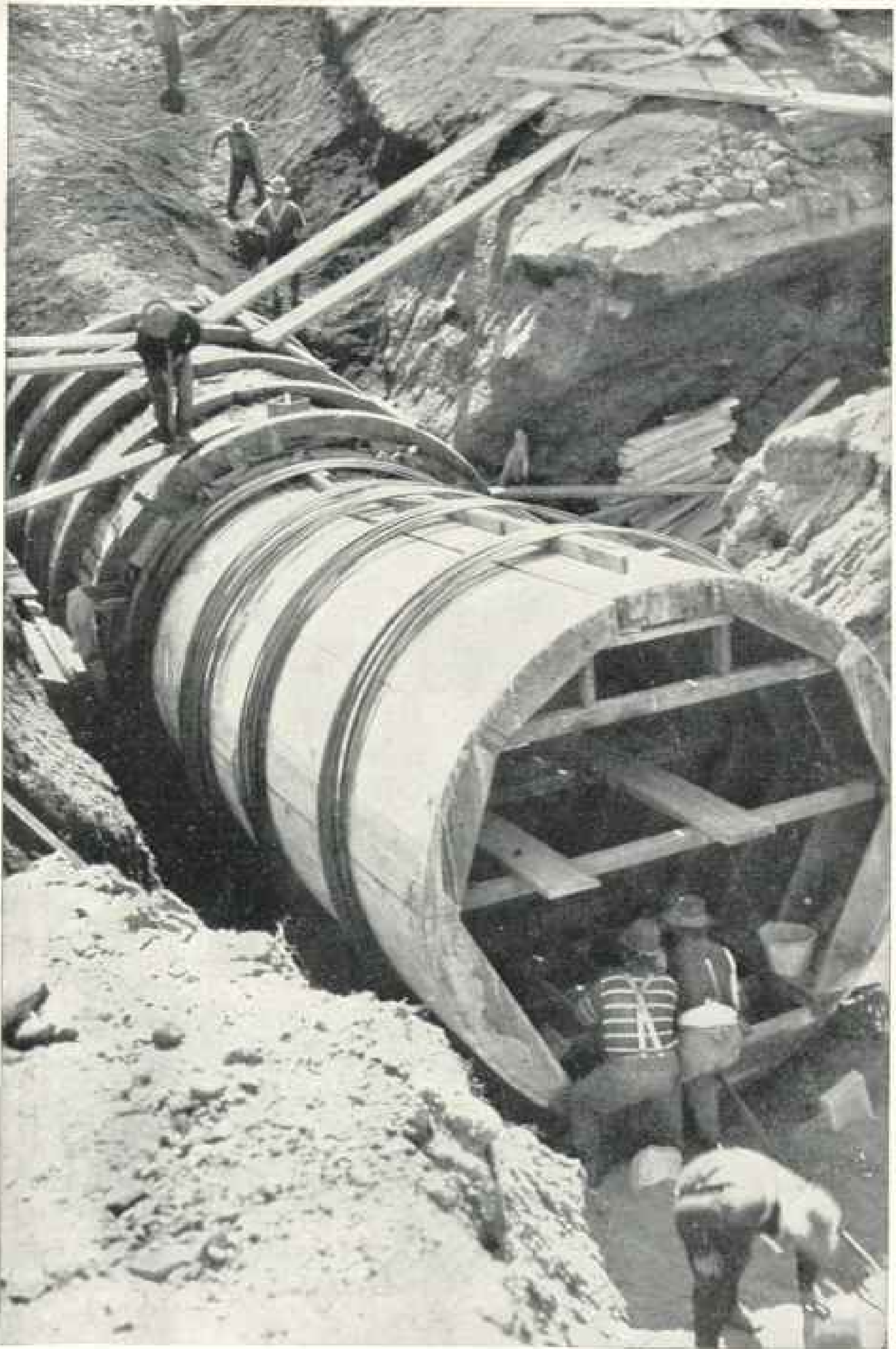
ANOTHER VIEW OF AN INVERTED SIPHON: IT IS BUILT OF CONCRETE, HEAVILY REINFORCED WITH STEEL. (SEE PAGE 576)
