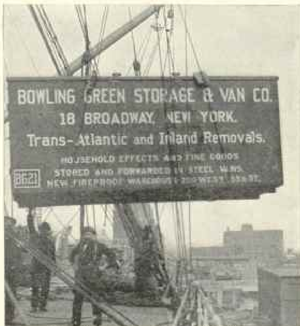
HOISTING LIFT-VAN ON BOARD STEAMSHIP
