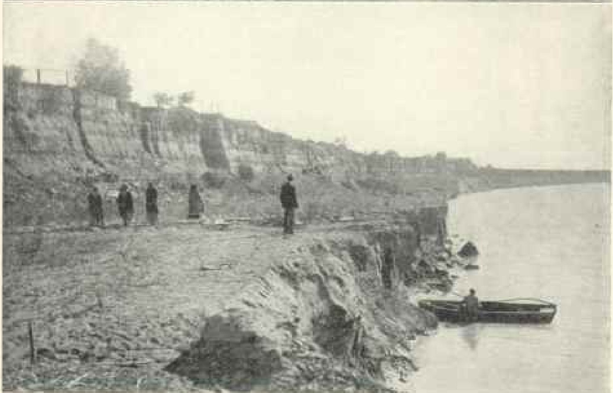
END OF THE PROTECTIVE LEVEE AT THE INTAKE OF THE IMPERIAL CANAL SYSTEM BELOW YUMA. CUT THROUGH AND DESTROYED BY THE COLO- RADO RIVER IN DECEMBER, 1906
