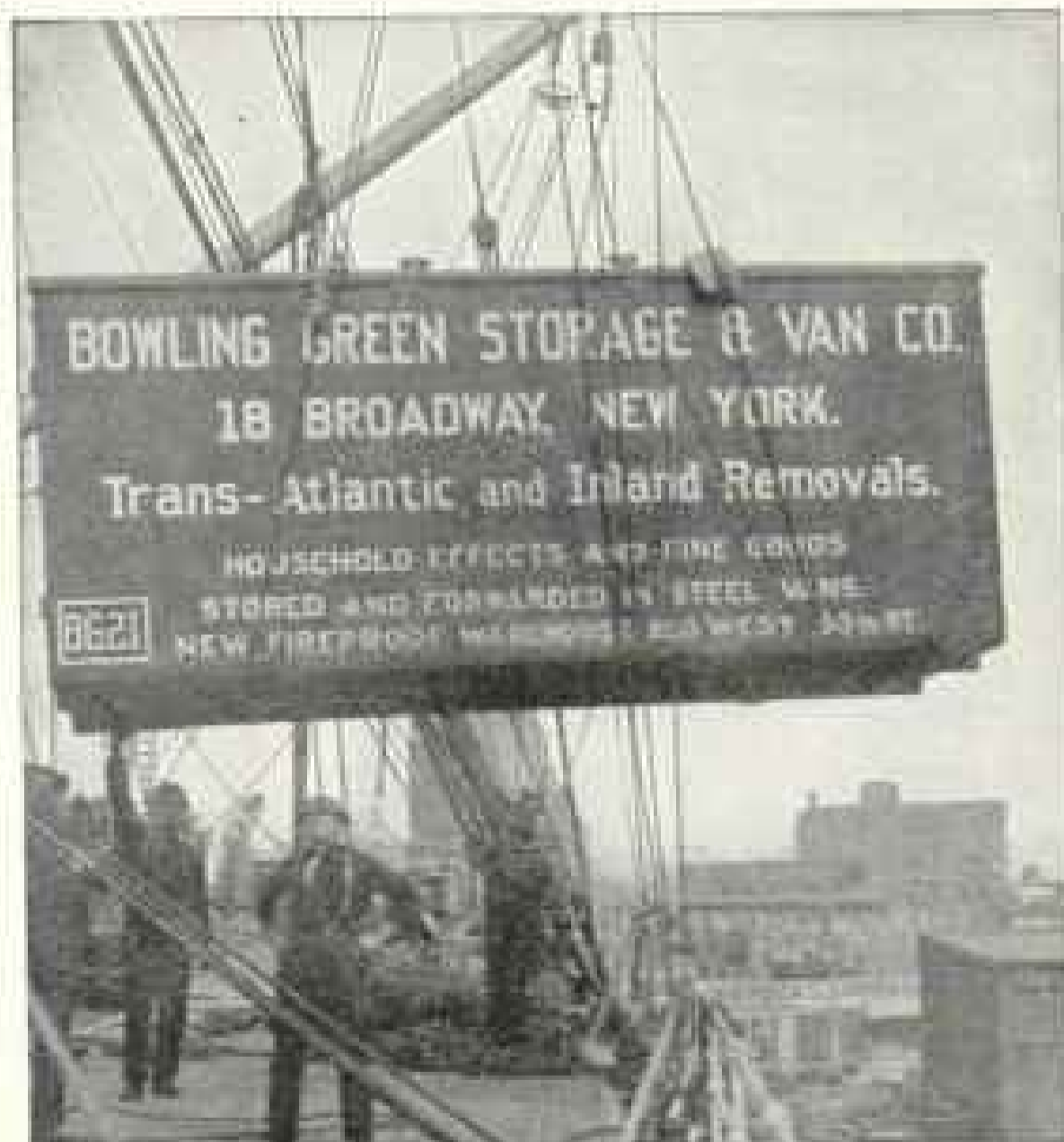
HOISTING LIFT-VAN ON BOARD STEAMSHIP
