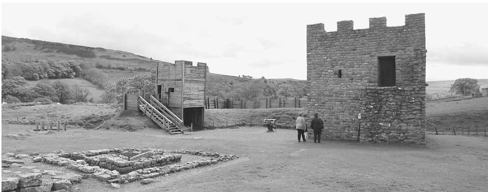
Roman towers at Vindolanda. (Chris McKenna)
