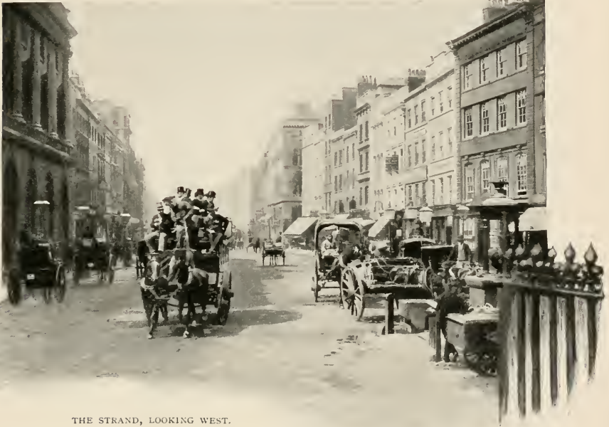
THE STRAND, LOOKING WEST.
