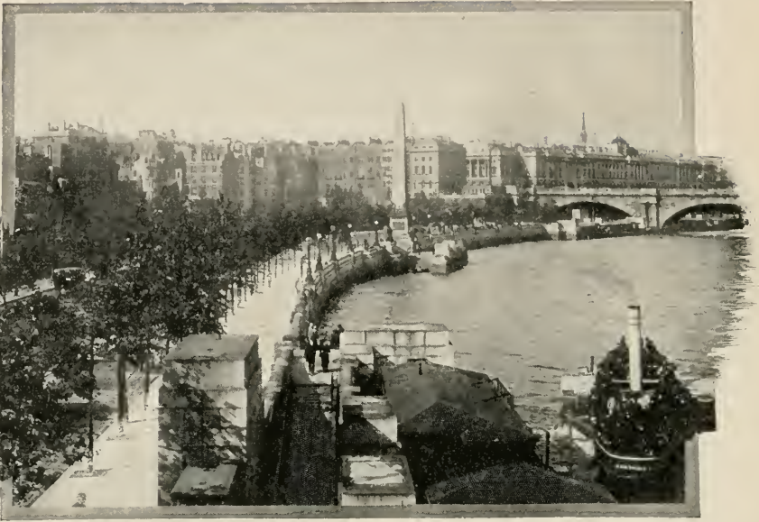
THE VICTORIA EMBANKMENT.
