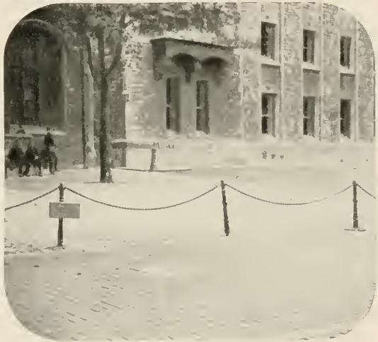
THE SITE OF THE SCAFFOLD.
