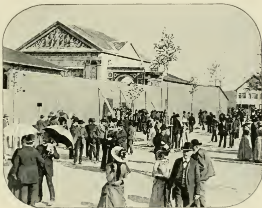
OUTSIDE THE ENCLOSURE.
