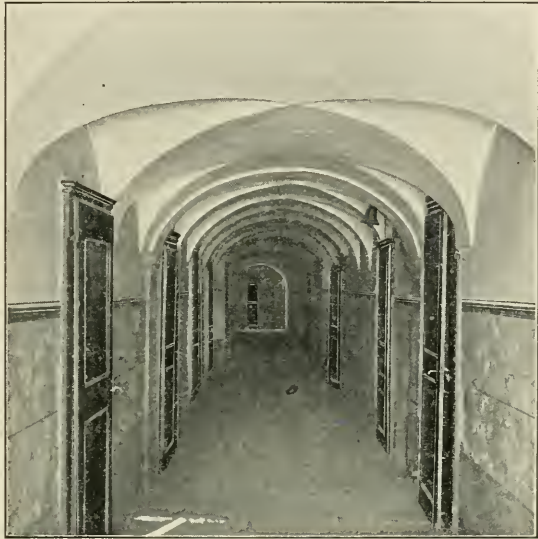
A CORRIDOR IN THE HOSPICE.
