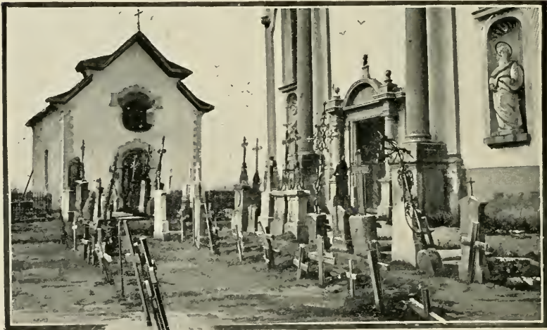
WHERE SEVERAL ALPINE CLIMBERS REST.
