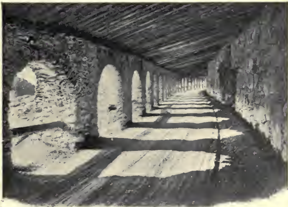
AVALANCHE GALLERIES ON THE BERNINA PASS.
