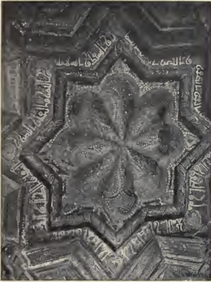
A SECTION OF THE CEILING.
