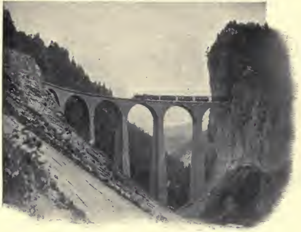
A VIADUCT ON THE NEW RAILWAY.
