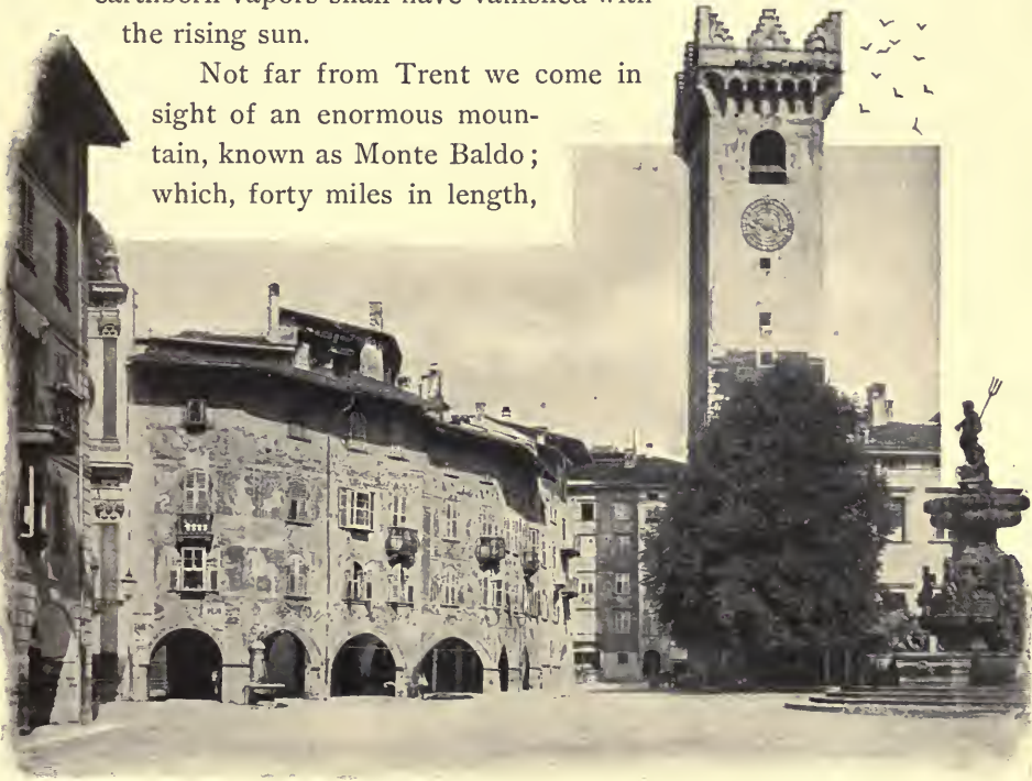
OLD BUILDINGS, TRENT.
