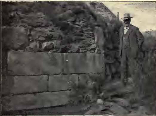
FOUNDATION OF THE OLD ROMAN BRIDGE.
