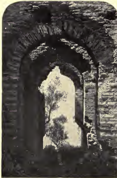
A CORRIDOR OF THE PAST.
