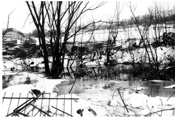
Fig. 6.16. River Chura in Moscow. We see large-scale construction works in progress, with excavators on the left. A motorway is being built here; the entire territory shall soon look differently. The river will either disappear, or have to run through pipes. We have managed to photograph the river in the last months of its existence. Photograph taken in January 2001.
