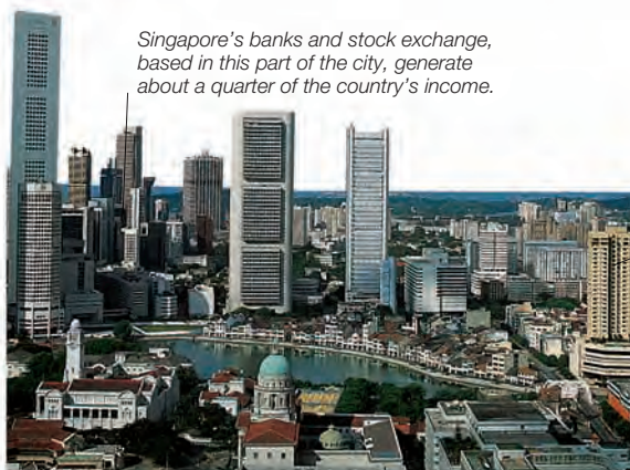
Singapore’s skyline is dominated by modern high-rise buildings, built because land is in such short supply.
