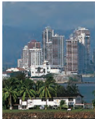
Banks and business centers line the canal approach to Panama City.
