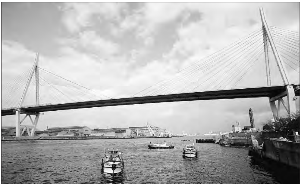
Tenpozan Watasi bridge in Osaka, Japan. (PhotoDisc)
