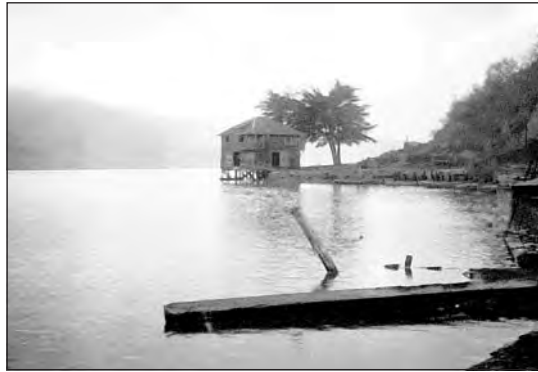
High tide at Bolinas Lagoon in California's Marin County in 1906. (U.S. Geological Survey)
