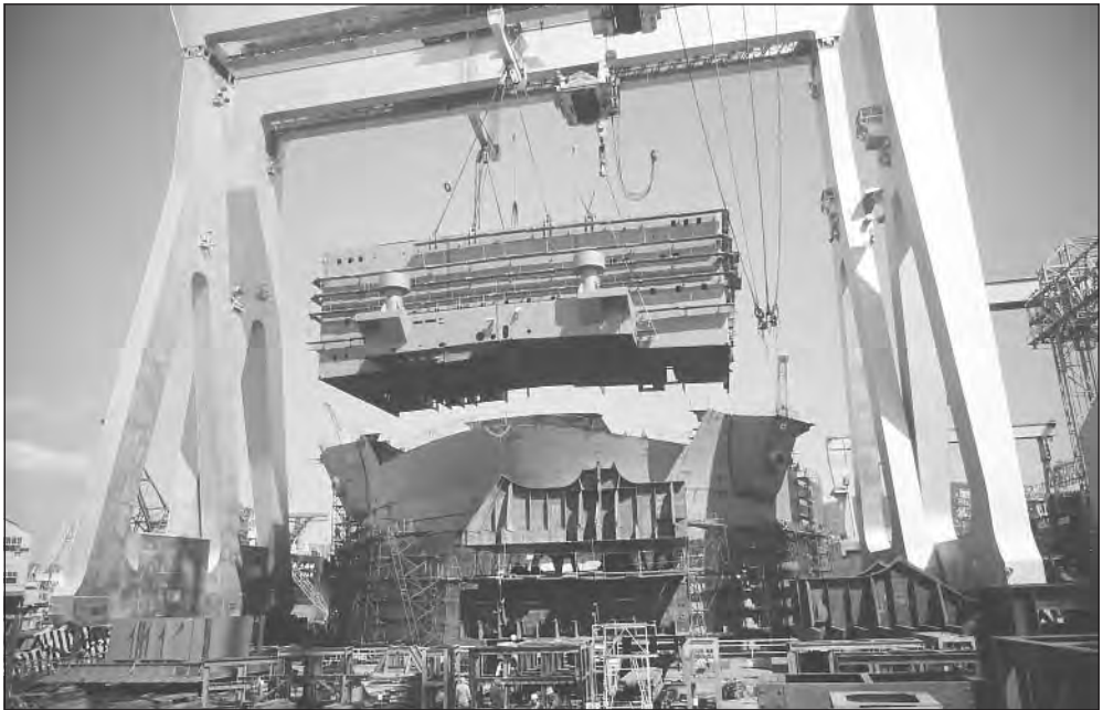
Crane lifting cargo containers at an Asian shipyard. (PhotoDisc)
