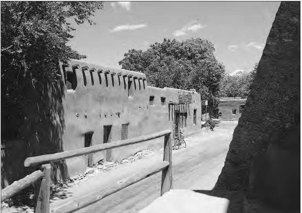
For thousands of years the people of the American Southwest have used the red clay soil to make adobe bricks—a building material with excellent insulating properties that is ideal for the region. (PhotoDisc)
