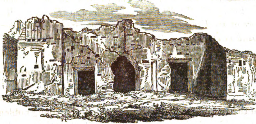
Excavations in the Rock at Athens, commonly called the Prison of Socrates.
