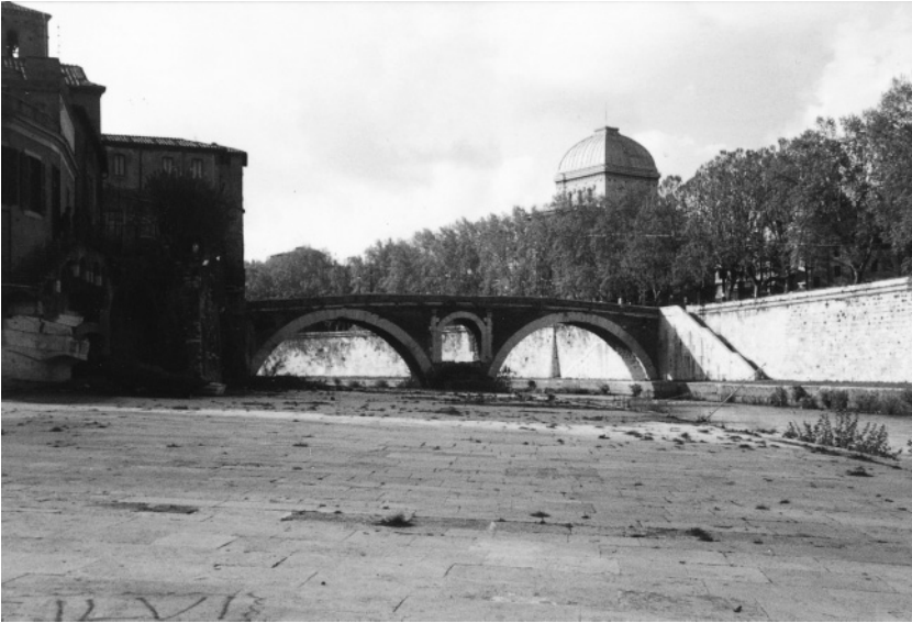
Figure 8 The bridge (seen from the south) originally constructed by Lucius Fabricius, a curator of roads, in 62 BC which connected the Tiber island and its healing sanctuary of Aesculapius with the Campus Martius.
