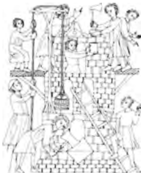
Pulley and wooden ladder (from Bible dating from the beginning of the 13th century) Wooden ladders have been used from time immemorial to carry building materials up onto a higher level. Pulleys were used to pull up mortar in tubs and buckets and small stones. In the picture above (behind the pulley) we can see a plumb level being used to monitor the upper edge of the wall.
