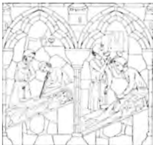
Stonemason's yard (c. 1220/30) Stonemasons were not only in charge of manufacturing ashlar; they were also responsible for making columns, capitals, and reliefs. Our picture gives the reader a view of a stonemason's yard and shows two stages in the manufacture of a stone sculpture. The stonemason's tools - wooden mallet and chisel - can be clearly seen on the right.
