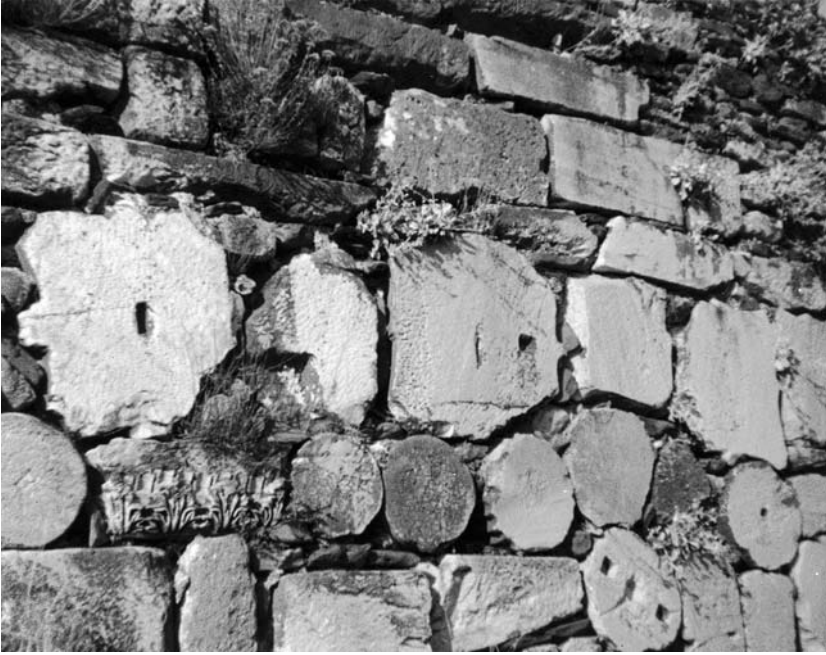
Figure 31b Marble column drums, probably from the Temple of Artemis, reused for the walls of the Byzantine hilltop fortress at Sardis
