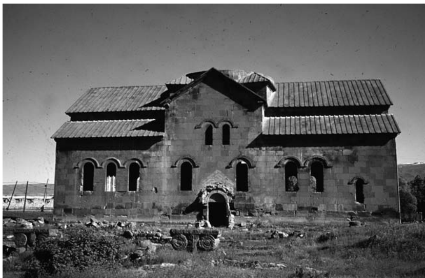
Figure 22 The southern façade of the palatine church of Aruch, built by Mu‘awiya’s principal Armenian client, Gregory Mamikonean, and his wife Heline in 670. A columned palace has been excavated immediately to the south of the church, attested by the capital in the foreground
