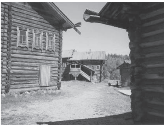
FIGURE 3.7. Typical houses in Malye Karely, Arkhangelsk Oblast, showing northern Russian architecture. Note the covered section that is lower than the rest of one house; this serves as a winter shelter for animals. Photo: A. Shanin.
