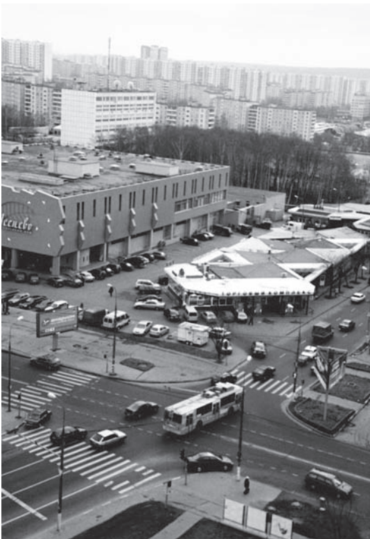
FIGURE 11.9. Yasenevo, a typical late Soviet microrayon, built in the 1980s on the periphery of Moscow. It has multistory apartment buildings, playgrounds, day care centers, schools, clinics, and shops along the periphery. The retail kiosks date from the 1990s. Photo: I. Blinnikova.
