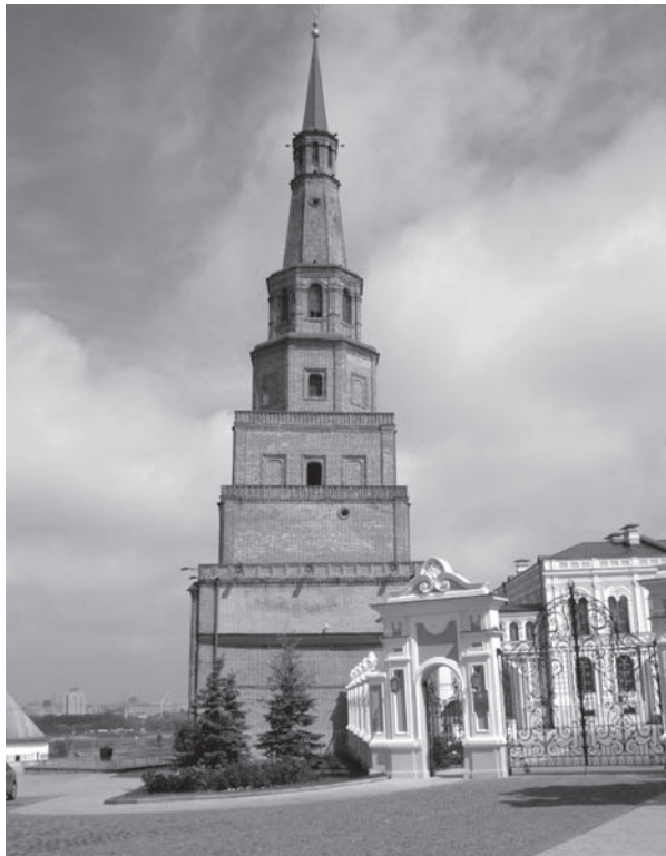
FIGURE 2. Suyumbike was built in the late 17th century in Kazan, probably as a guard tower. Its tilt from the vertical is 1.8 m near the top. Photo: S. Blinnikov.
