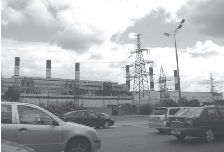
FIGURE 5.2. The smokestacks of the Yuzhnaya power station in Moscow, as seen from the beltway. Twenty such plants surround the city and provide both electricity and hot water to millions of customers. Increasing car traffic more than offsets any gains produced by cleaner central power production, however. Photo: Author.
