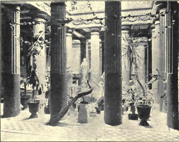
PERISTYLE OF THE POMPEIIAN HOUSE AT SARATOGA SPRINGS, N. Y. Franklin W. Smith, architect.
