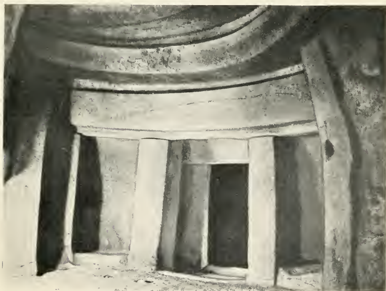
FIG. 14. HAL SAFLIENI. KERNEL OF STRUCTURE, SHOWING CORBELLED ROOF. (Photo, T. M. Salmond, Esq.)
