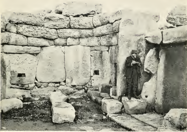
FIG. 12. MNAIDRA. CORBELLING, COURSES, AND WINDOW-OPENINGS.
