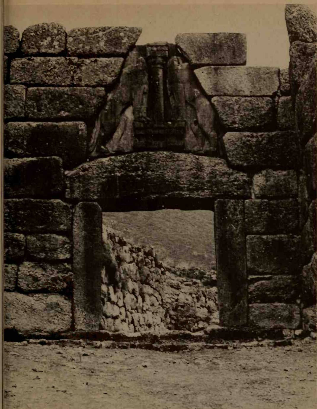
8 The Lion Gate at Mycenae. Two lions, their heads missing, stand heraldically at either side of an altar supporting a column. The triangular gap, filled by the slab, helps to relieve the weight of masonry on the great lintel. Thirteenth century B.C.
