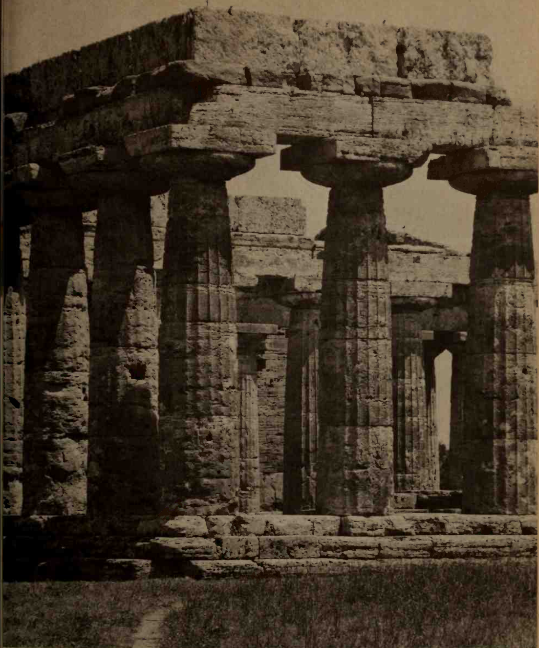
56 The Doric Temple of Hera (the so-called 'Basilica') at Paestum. A good example of the early cigar-shaped columns with bulging capitals. Mid sixth century B C
