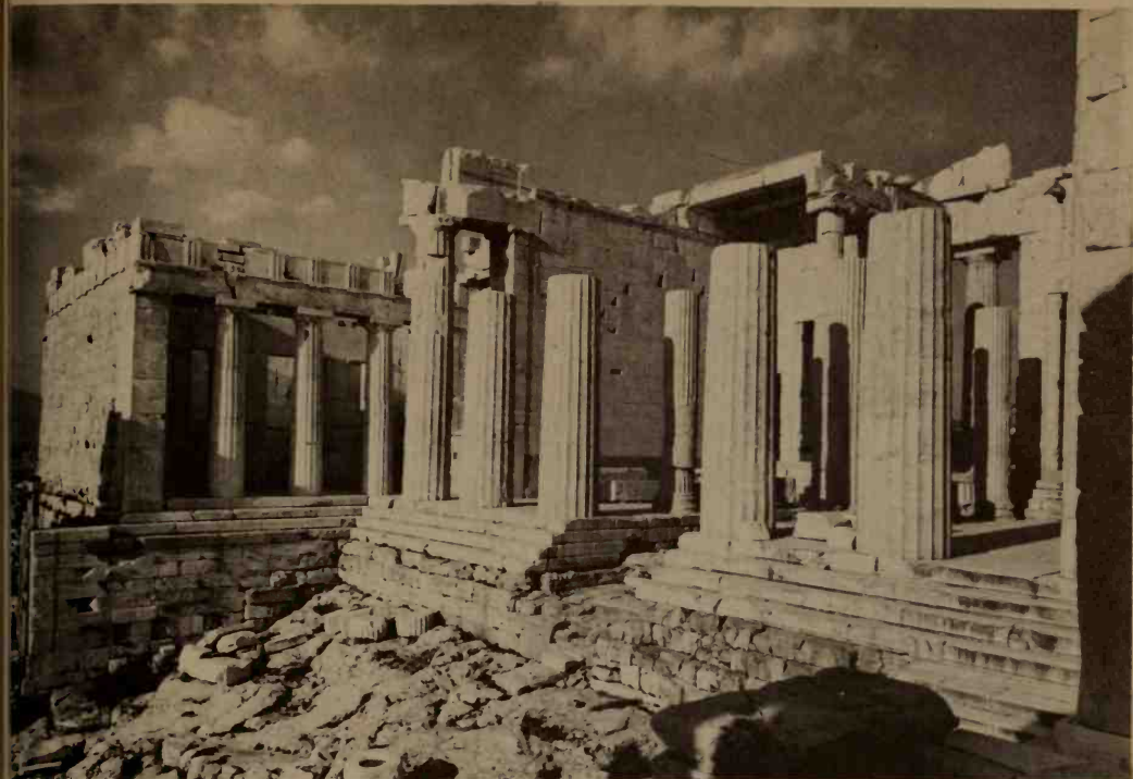
121 The Propylaea to the Acropolis at Athens, from the south-west. An Ionic column from the centre passageway can be seen centre right. Built 437-432 B.C., to plans of Mnesicles. Width of entrance front 18.5 m
