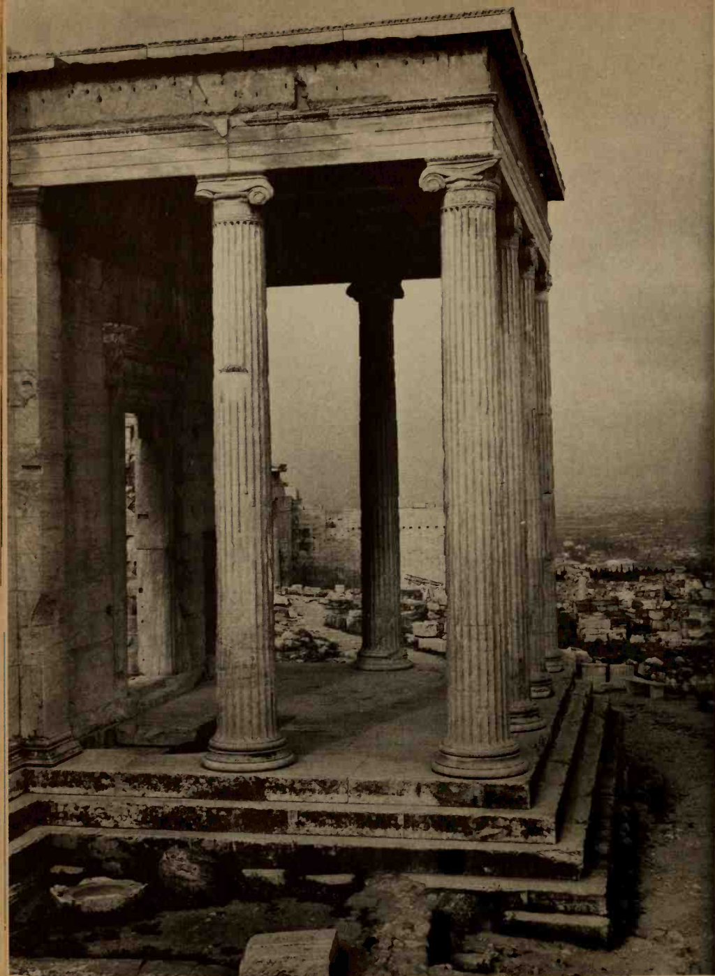
124 The Ionic north porch of the Erechtheion, on the Acropolis at Athens, from the east. The holes which fastened the frieze figures to the darker backing marble can be seen just below the roof. Built intermittently between 421 and 405 B C
