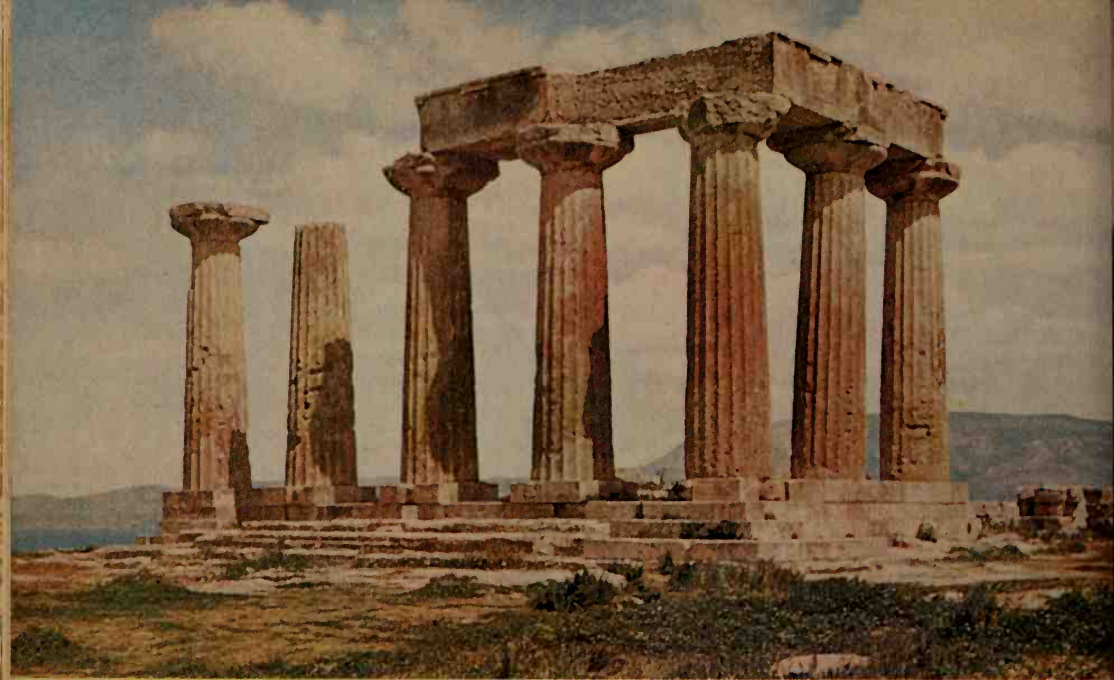
55 The Temple of Apollo at Corinth; the earliest Doric temple in Greece with some of its monolithic columns still standing. Mid sixth century B C
