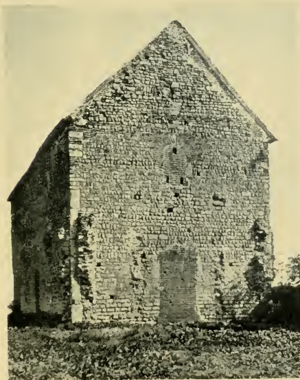
West-end of St. Peter-on-the-Walls.
