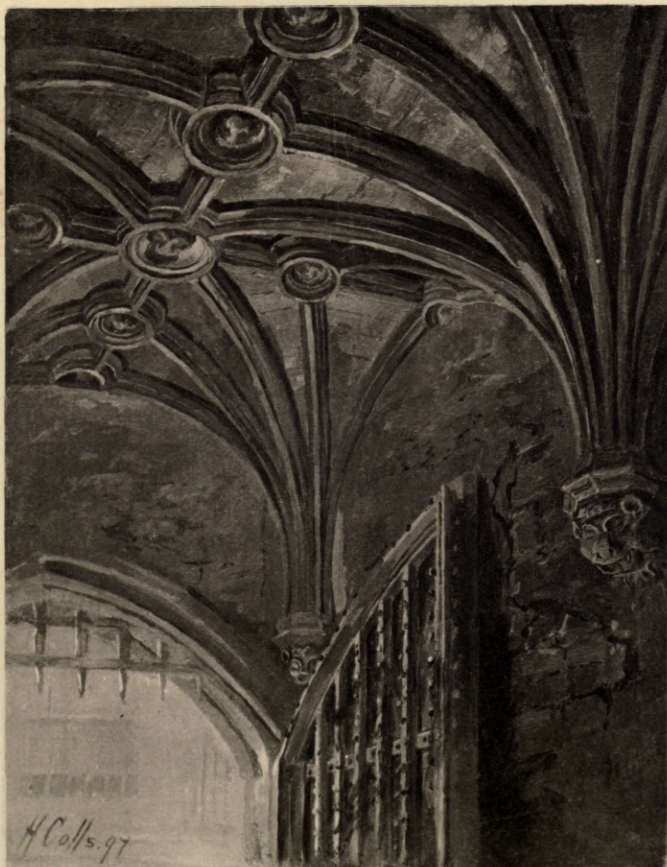
Groining in Ceiling of the Bloody Tower.
