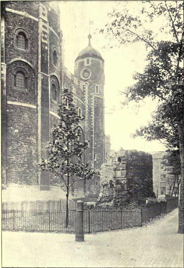
The White Tower, showing the Exterior of St. John's Chapel and remains of the Roman Wall
