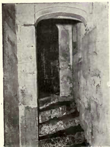
STAIRCASE IN BLOODY TOWER LEADING TO VAULT IN THE WAKEFIELD TOWER.
