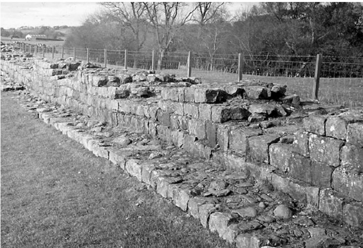
Plate 3.2 Willowford (Northumberland): 'Narrow' gauge wall built on the north front of the already-constructed broad foundation.
