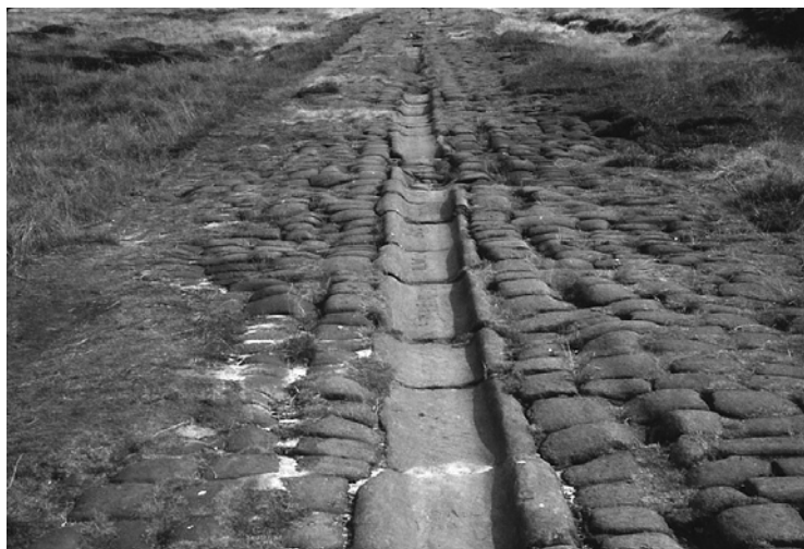
Plate 4.1 Blackstone Edge (Greater Manchester): Section of paved Roman road between Manchester and York; the gradient is in places 1 in 4.
