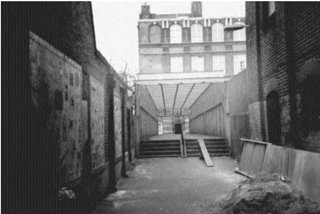
Wood's Buildings, looking from Whitechapel Road toward what was Winthrop Street and the school. If Jack was disturbed by the approach of Charles Cross, he may well have escaped by dashing around the school and running down this alleyway toward the point from which the photograph was taken. (Yvonne Berger)
