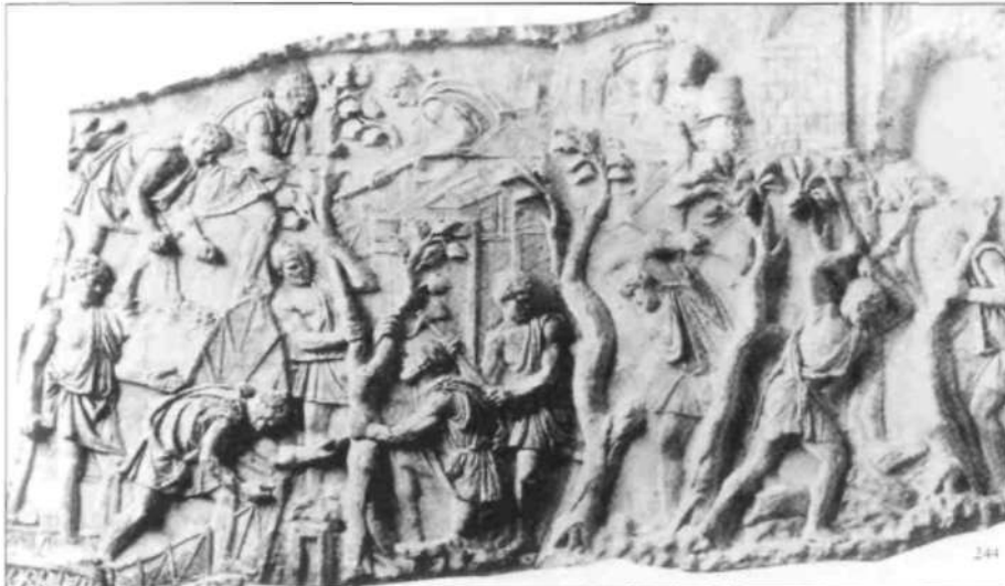
A scene from Trajan's Column (Scene XCII) depicting legionaries, working without body armour, constructing a road through a forest. Those hewing wood are using the dolabra , a tool commonly associated with digging. (Reproduced from Lepper, F. and Frere, S. S., Trajan's Column: A New Edition of the Chicorius Plates , Sutton, Stroud, 1988)
