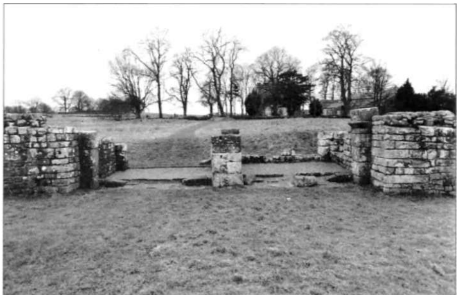
The east gateway at Birdoswald fort ( Banna ), as seen from outside the fort, the best-preserved example on the Wall. Of particular interest are the double-portals and one of the springers (the part of an arch where the curve begins) for an arch over the northern passage. (Author's Collection)
