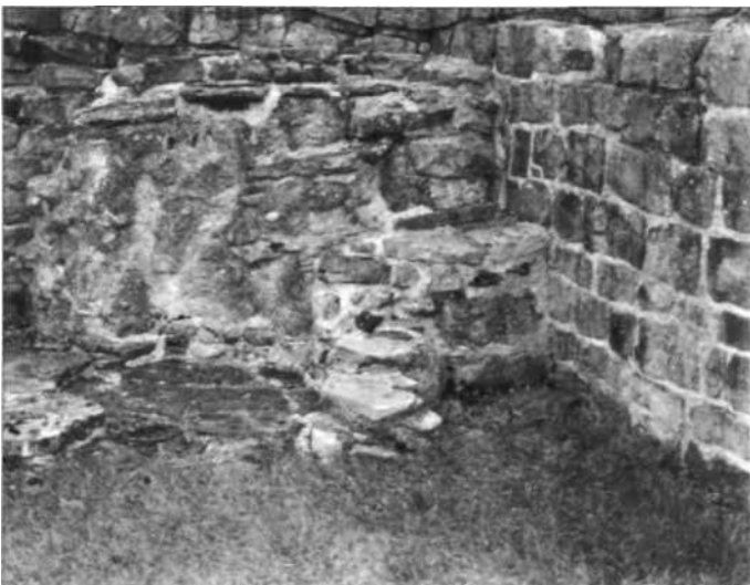
The remains of the bread-oven situated in the north-west angle of the rampart of milecastle 48 (Poltross Burn). Bread-ovens were always positioned in the ramparts so as to reduce the risk of fire. (Author's Collection)
