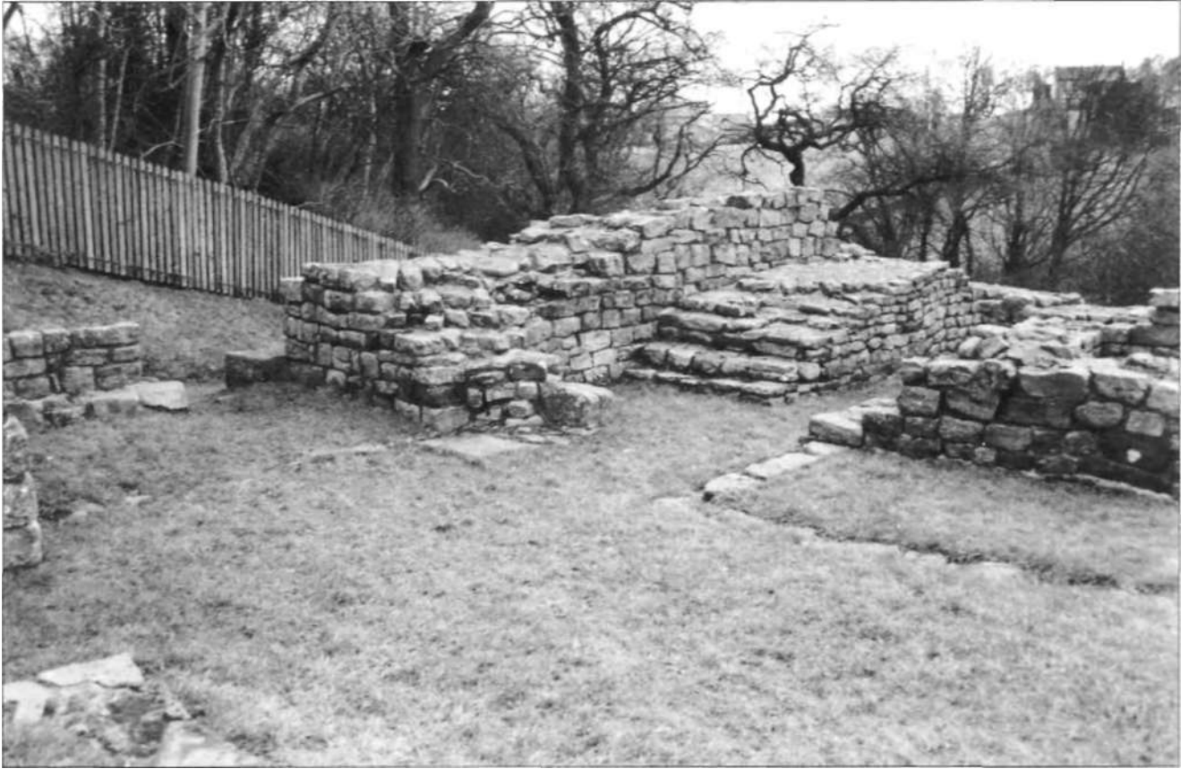
The conspicuous remains of the internal stairway at milecastle 48 (Poltross Burn), which gave access to the rampart-walkway and the tower above the north gateway. This stairway is exceptional and has not been found in other milecastles. (Author's Collection)
