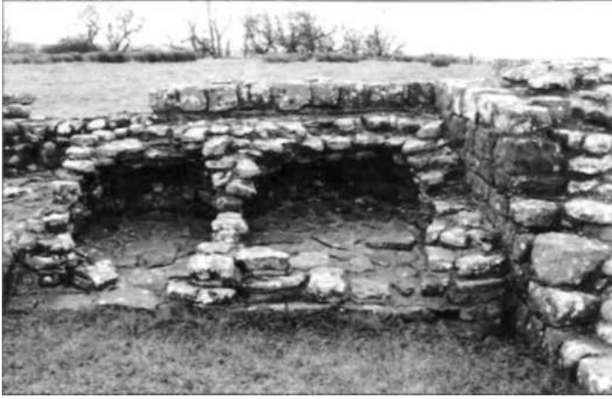
A group of bread-ovens cut into the back of the earth rampart by the south gateway at Birdoswald fort ( Hanna ). The surviving structures consist of a raised stone flagged floor and low stone walls upon which rubble and clay domes would have rested. (Author's Collection)
