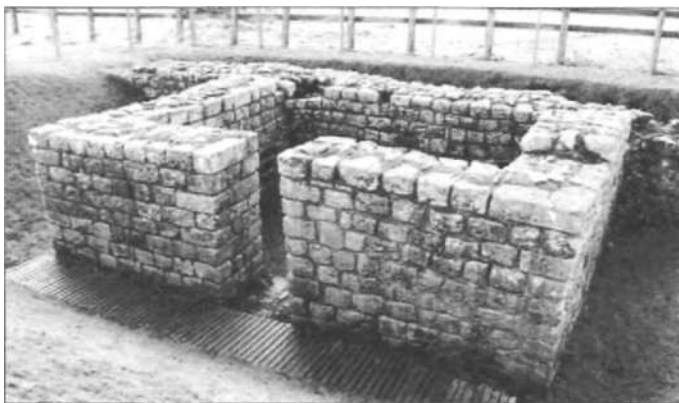
The interval tower between the south-east angle-tower and south gateway at Chesters fort (Cilurnum). The tower is built projecting inwards from the curtain-wall, a common feature of first- and second-century AD Roman fortifications. (Author's Collection)
