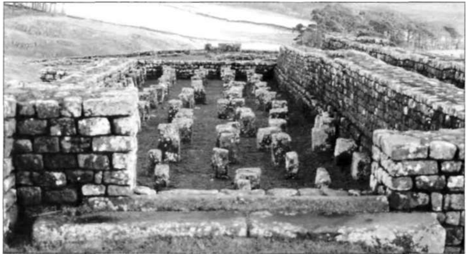
The pillared floor-supports and loading platform of the north granary at Housesteads fort ( Vercovicium ).The pillars once supported a flagged floor to be seen at Corbridge and Birdoswald. (Author's Collection)
