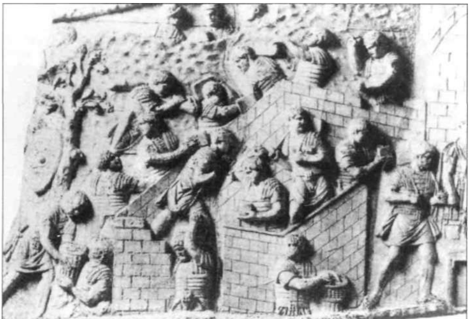
A scene from Trajan's Column (Scene LX) in which legionaries, working in body armour but bare-headed, dig ditches and cut and handle turf-blocks - note the rope sling to carry turf-blocks on their backs and the use of baskets to move soil. (Reproduced from Lepper, F. and Frere, S. S., Trajan's Column: A New Edition of the Chichorius Plates . Sutton, Stroud, 1988)
