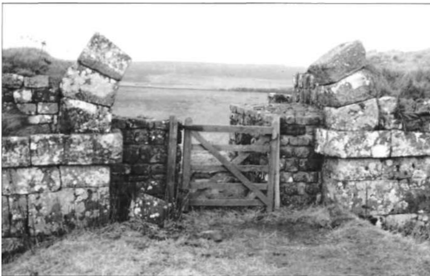
The north gateway of milecastle 37 (Housesteads) as seen from inside the milecastle. The arch stones have been partially restored. (Author's Collection)
