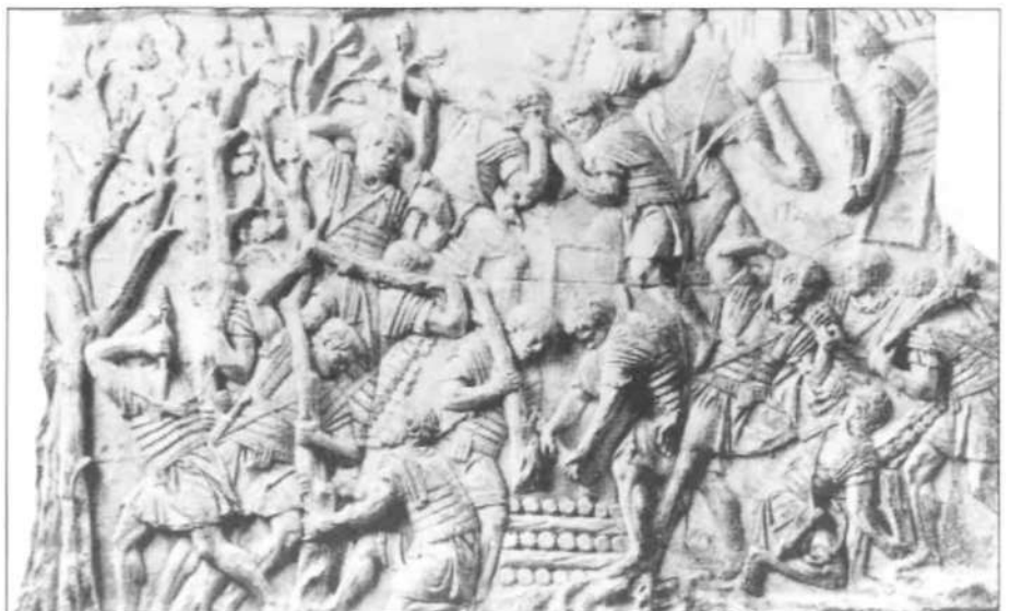
RIGHT A scene from Trajan's Column (Scene CXVII) in which a legionary work-party cuts and gathers timber. The cut timber is being stacked neatly ready for transportation. (Reproduced from Lepper, F. and Frere, S. S., Trajan's Column: A New Edition of the Chieorius Plates , Sutton, Stroud, 1988)
