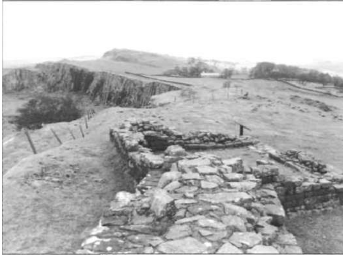
Turret 45a (Walltown) clearly recessed into the Wall, looking north-east. This turret is especially remarkable, for it was built as a free-standing look-out tower before the Wall was brought up to its east and west sides. (Author's Collection)
