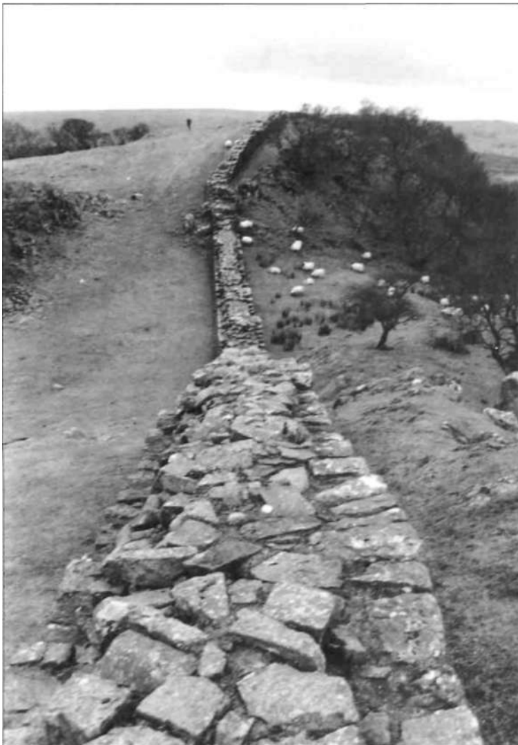
The Wall at Walltown Crag, looking south-west from turret 45a (Walltown), showing the facing-stones and rubble-core used in its construction. This is a section of the Narrow Wall. (Author's Collection)
