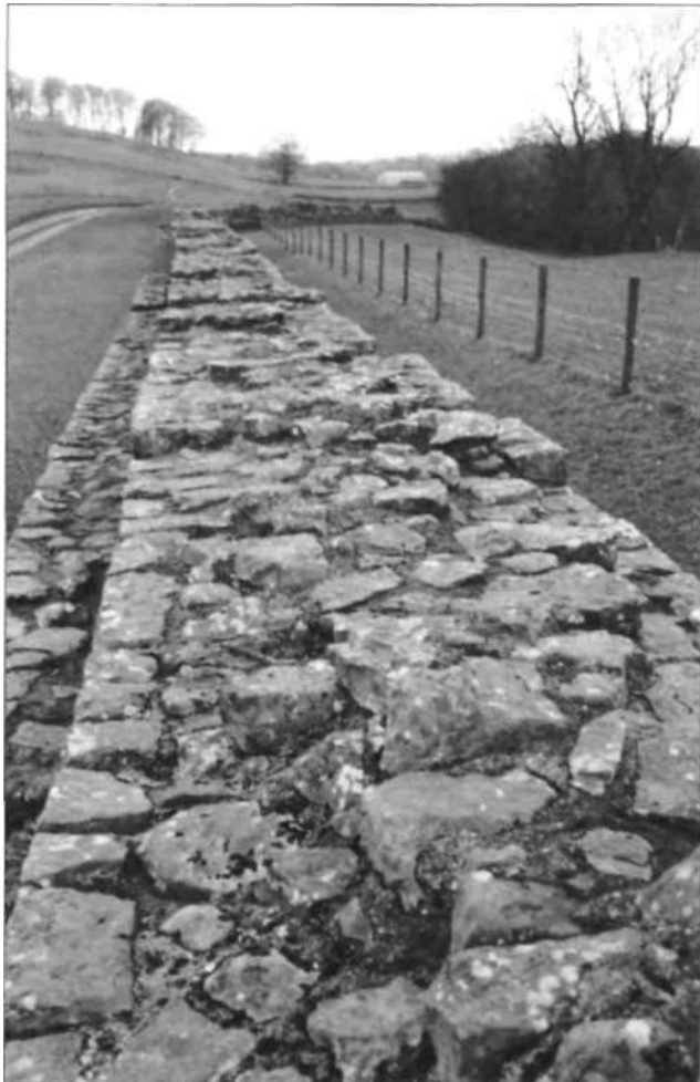
The Wall east of turret 48a (Willowford East) showing the horizontal offset where the Narrow Wall has been built on a Broad Wall foundation. (Author's Collection)
