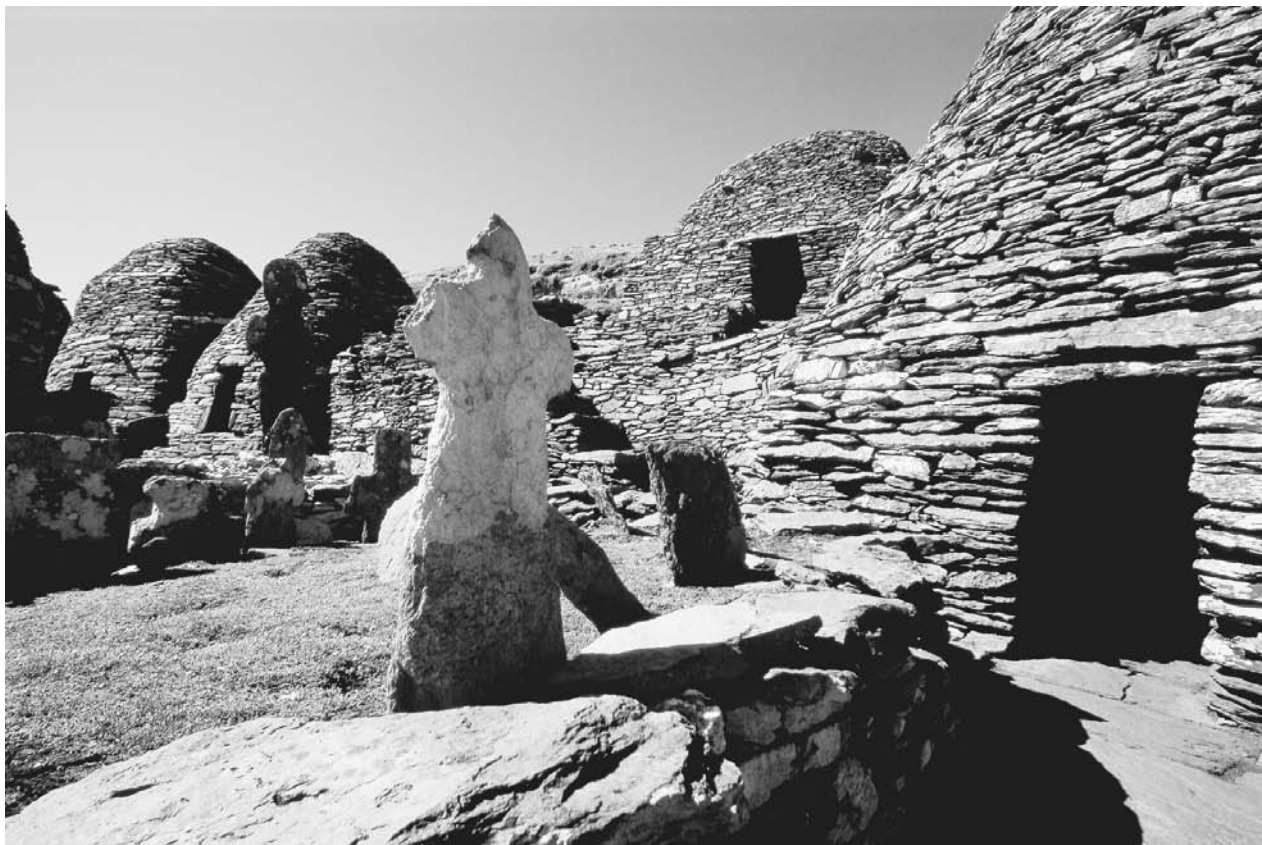
Beehive stone huts on Skellig Michael, Co. Kerry, dating to the seventh to eighth century. These huts are round outside and square inside, some with wall cupboards (for books and vessels). © MICHAEL ST. MAUR SHEIL/CORBIS. REPRODUCED BY PERMISSION.
