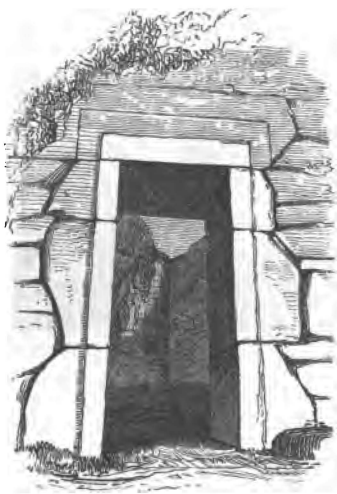
Doorway of Lady's Church.
