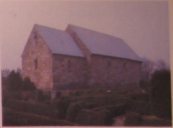
Fig. 9. Sædding church, W. Jutland, Denmark, is a typical Jutland rural parish church, built of squared granite blocks, in the 12th cent
