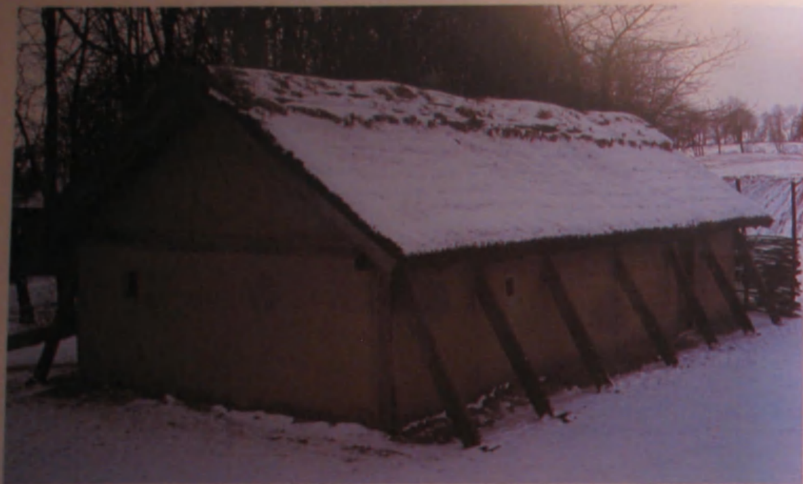
Fig. 1 Full-scale reconstruction of a house from Hedeby, the greatest trading centre in Viking Age Scandinavia. The house was built in 870 and measured 5 × 12m. The walls were of wattle-and-daub in a timber
