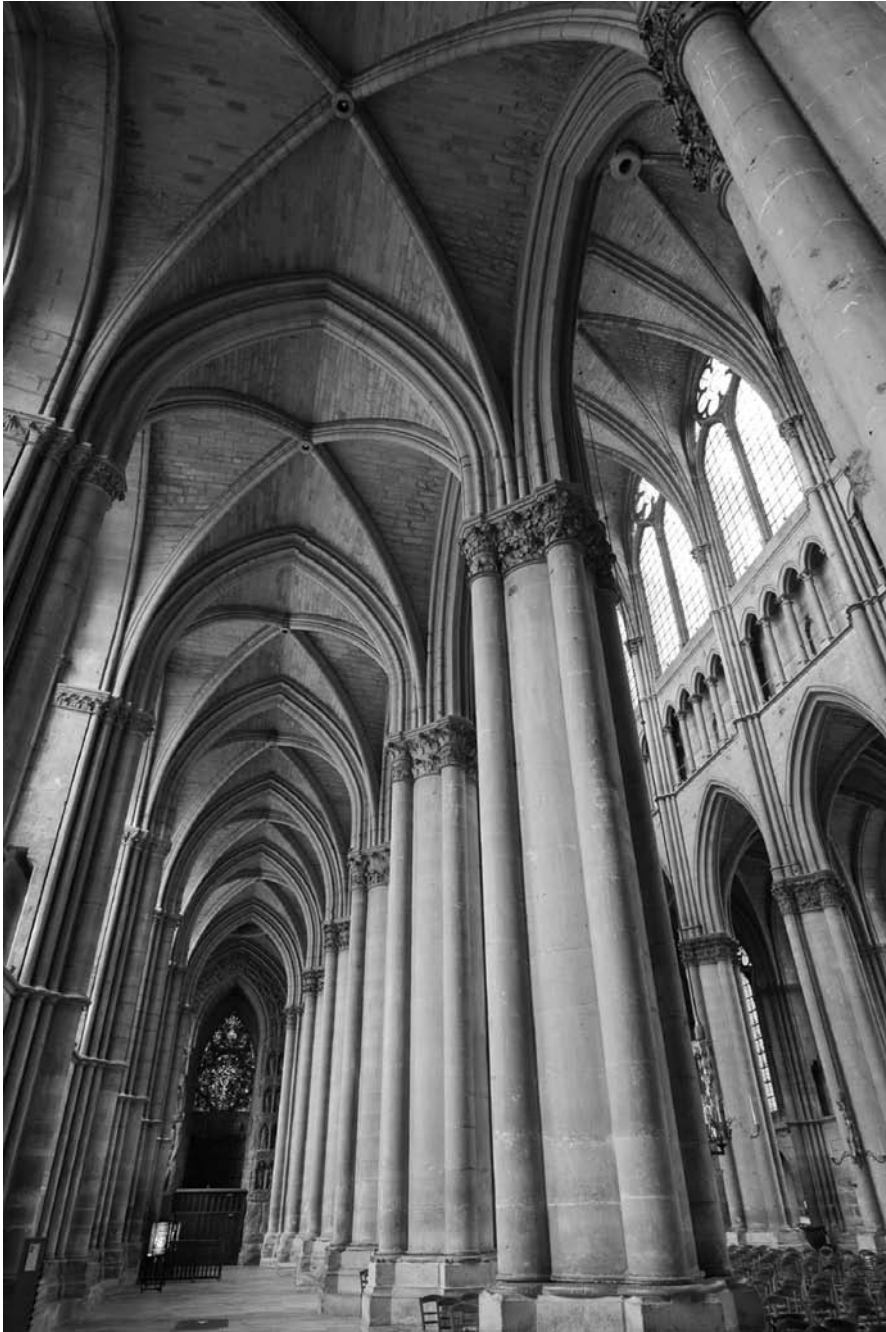
Ribbed vaults in Reims Cathedral hold up the vaulted ceiling with far less stone than in previous construction methods. Three arches (transverse, lateral, and diagonal) rest on each cluster of columns. The thin stone ribs lean on a round boss, visible at the point of the X. The delicacy of the weight-bearing skeleton allows maximum space for windows. (Claudio Giovanni Colombo/iStockphoto)
