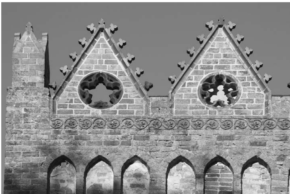
Medieval bricks could be thicker or thinner than modern standard bricks, and different clays varied their color. This Cistercian abbey in Germany added decorative bricks. (Andreas Bauer)
