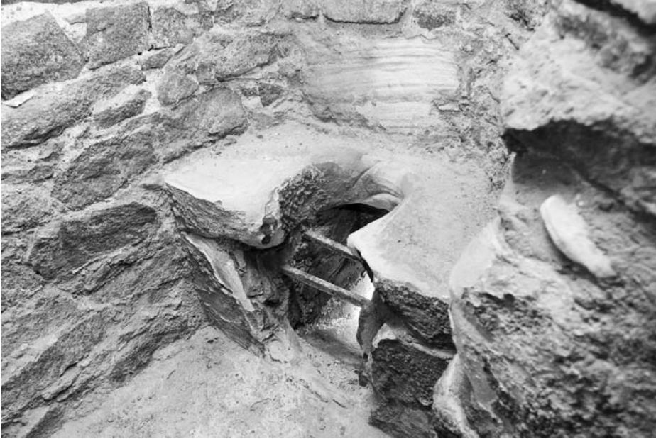
This castle garderobe has survived better than many since not only the closet and chute but also the seat were made of stone. Daylight shines up through the hole, which leads straight to the sea. (iStockphoto)
