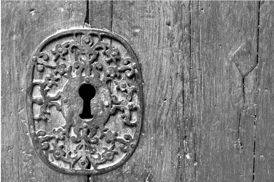
The face plate of a door lock protected and hid the mechanism behind. It was easier to make an elaborate plate than to design a lock that could not be picked. By the late Middle Ages, locks had become reasonably sophisticated. (Dreamstime.com)
