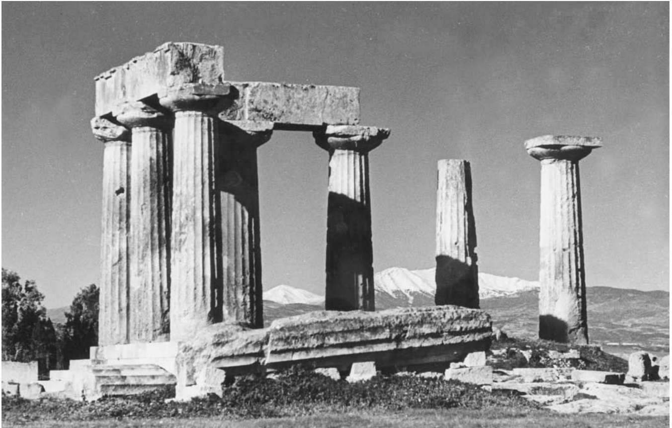
The Temple of Apollo at Corinth shows the fluted columns topped by rounded capitals of the Doric order in closer detail. ( Alison Frantz Photographic Collection, American School of Classical Studies at Athens )
