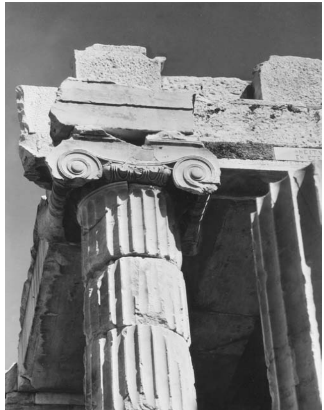
The Ionic order was used specifically in the construction of temples of the gods. The top or capital of each column was decorated with this scroll-like pattern. (Alison Frantz Photographic Collection, American School of Classical Studies at Athens)
