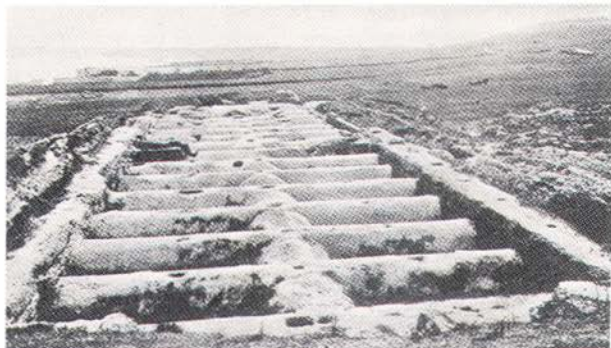
Carthage was razed to the ground in 146 B.C. and very little of the great city is now visible. Perhaps the most striking relics are these cisterns, part of the city's original reservoirs, consisting of 17 great barrel vaults. (Author's collection)
