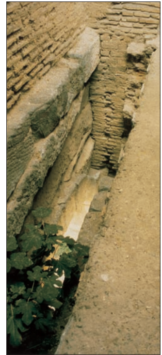
The interior of the Istanbul Gate of Iznik. (Frederick Nicolle photograph)
