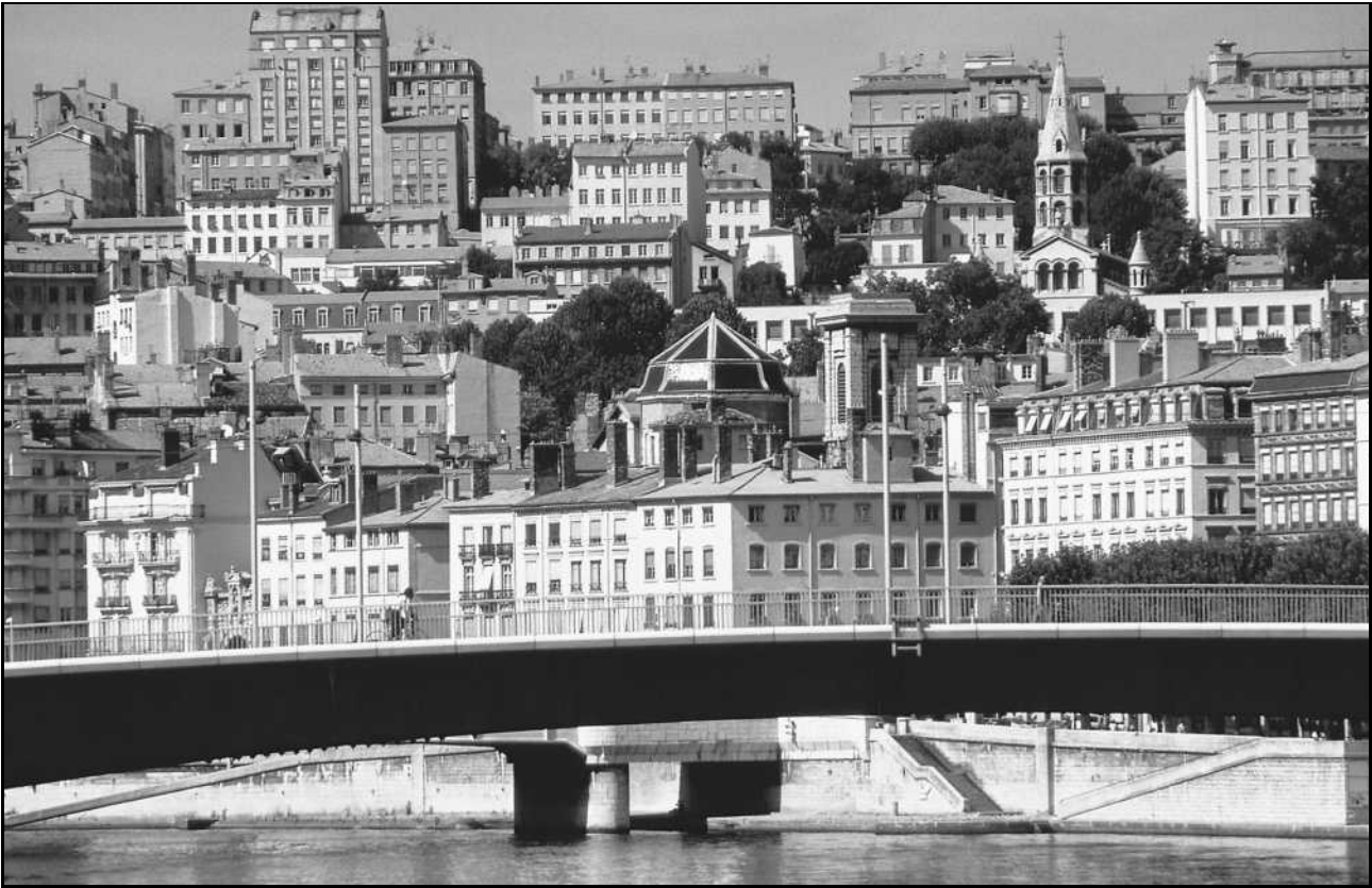
Bridge over Rhone River in Lyons, France
