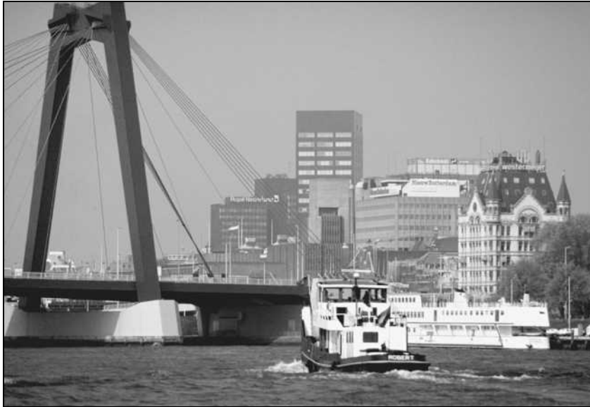
Bridge over Hollandse IJssel River in Rotterdam
