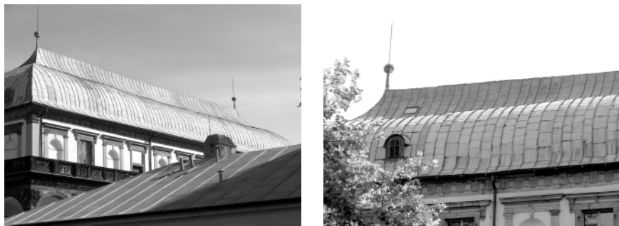
15.3 New patina layer after four years' exposure (a) eastern and (b) western sides).
