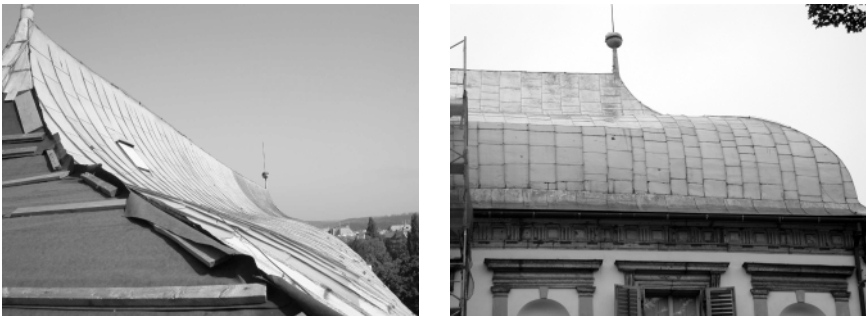
15.2 Reconstruction of the copper roof.
