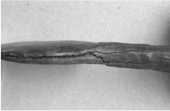
11.9 Flaking along the lines of cracks with powdery orange corrosion products.
