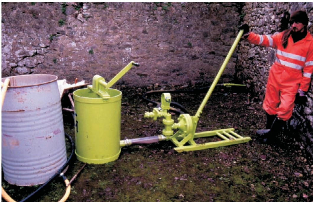
Figure 4.48 The simple diaphragm pump which has largely replaced gravity grouting of masonry walls.
