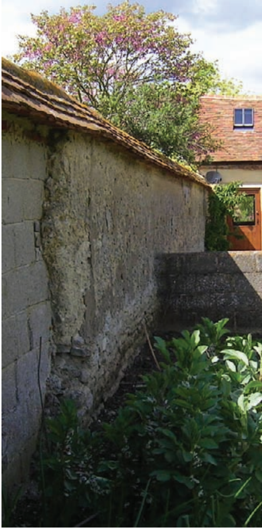
Figure 2.30 Wichert wall at Haddenham, Buckinghamshire.
