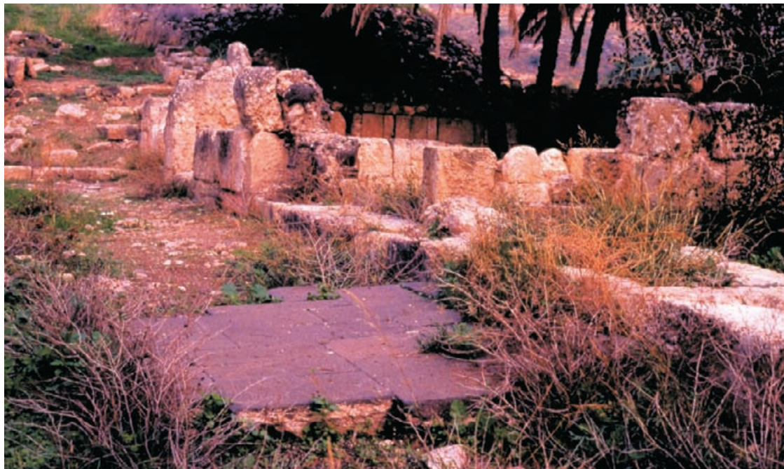
Figure 5.19 Section of mosaic pavement at Horvat Minim in Israel covered with geotextile, pozzolanic pellets and sand, which were found to be ineffective in protecting surfaces from vegetation (photograph: G. Abrey).
