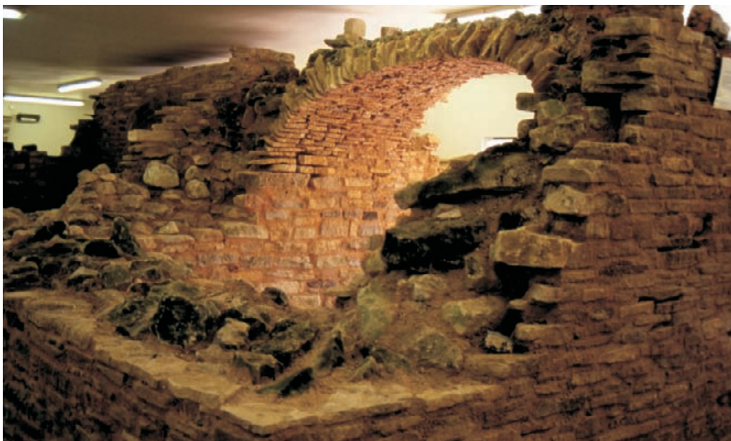
Figure 8.3 'Ruinette' at West Dean College, Sussex, England, designed by John Ashurst and Colin Burns and built by Gerry Williams and his team. The ruinette incorporates many of the conditions found in the field, such as unstable and voided core work, detaching faces, cracked vaults and overhangs. Practitioners can gain experience in consolidation work without risk to historic fabric.
