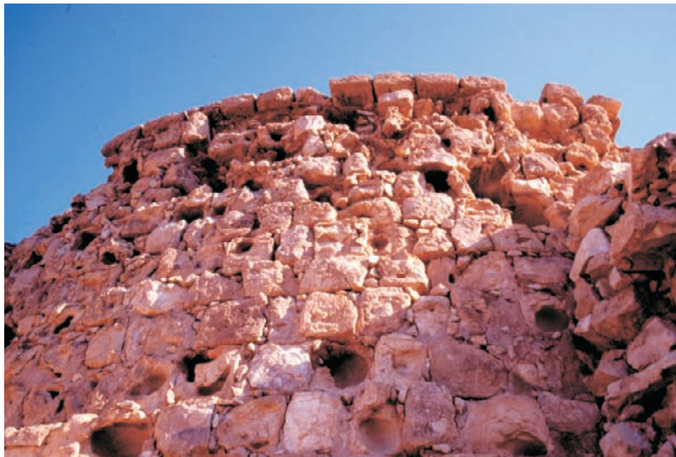
Figure 10.20 Early prototype of stone tile in lime mortar with a close texture to match stones in better condition. Thin mud washes are already blending the repair into the background.
