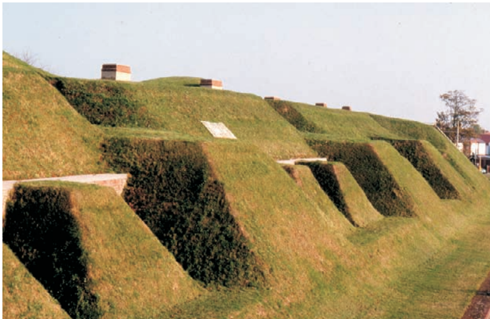
Figure 4.68 The use of earth and turf on the late nineteenth century Fort Brockhurst, part of the Palmerston Defences of the Naval dockyards of Portsmouth. The meticulously trimmed profiles quickly become wilder in appearance as grass gains height and wild flowers become established. Repairs are made in block bonded grass sods.
