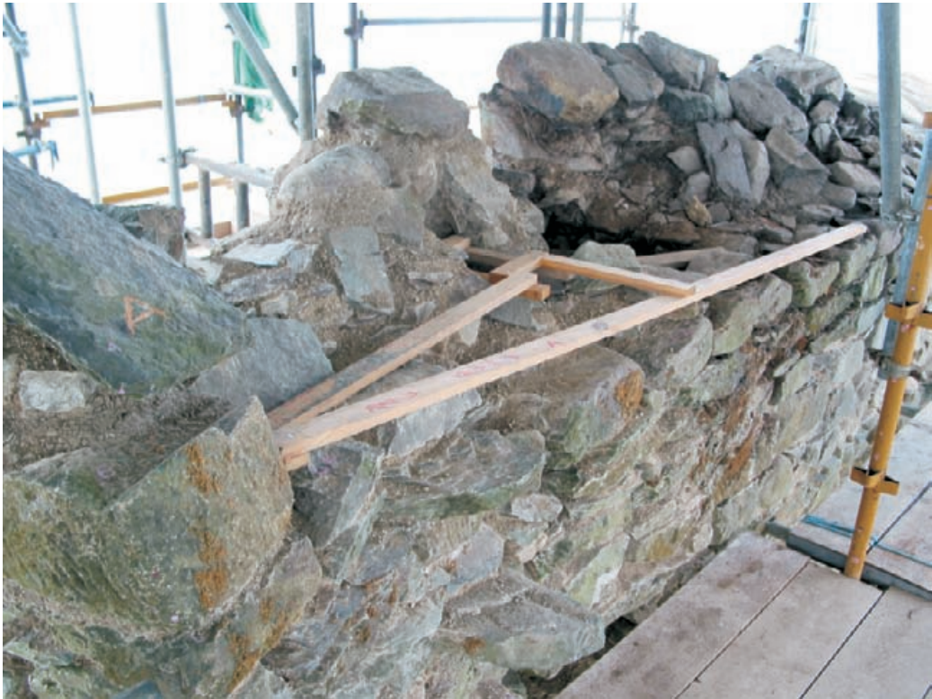
Training. Training exercises with John Ludlow's conservation technician team in County Cork, Ireland show, top, the use of the planning frame in marking out stone sizes and positions before taking down and rebuilding and, bottom, the use of profile frames in recording twists and distortions in the wall to enable the consolidated work to be built back in exactly the same positions.
