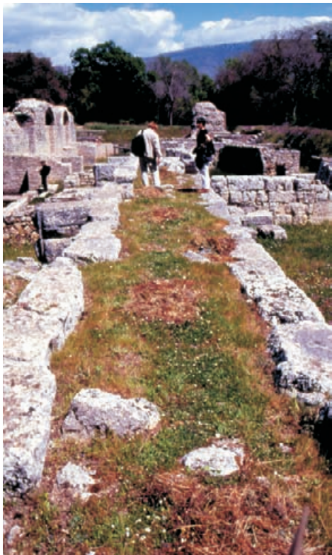
Figure 4.26 Perfect protection for this roofless ruin is provided by a mature mat of turf and wild flowers. This natural covering can hardly be improved on, and if the masonry below is stable, should be left alone.
