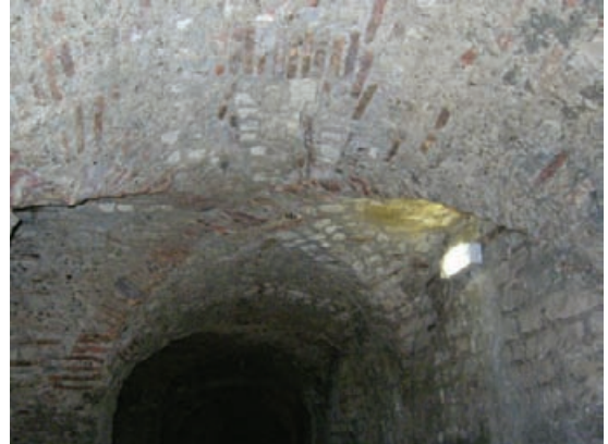
Figure 2.44 Diagonal brick ribs in Roman vault.
