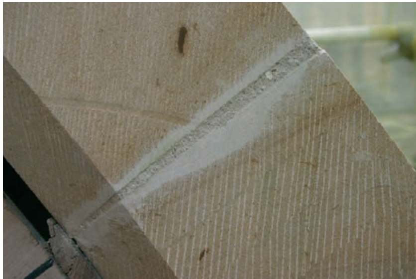
Figure 8.7 New stones are simply square blocks sawn six sides with a straight chamfer cut on two faces. Because there is no masonry involved the blocks still exhibit lash marks from the saw and a parody of tooling has been applied to the faces, even though there is no evidence of tooling on the original stones; the blocks form wedge-shaped joints and the blocks do not even line up. Some joints are imperfectly filled, and lime stains the surface of the stones.
