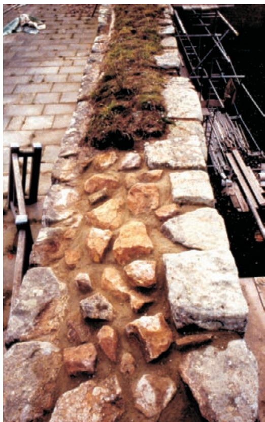
Figure 4.28 Walls built in clay mortar should not have cement or even lime-based mortar introduced as part of a consolidation process. Biodegradable net is used here to secure the loose wall heads after excavation, pegged with long plastic anchors deep into the core. In this wet area, grass and plants native to the site soon take over the wall tops again.
