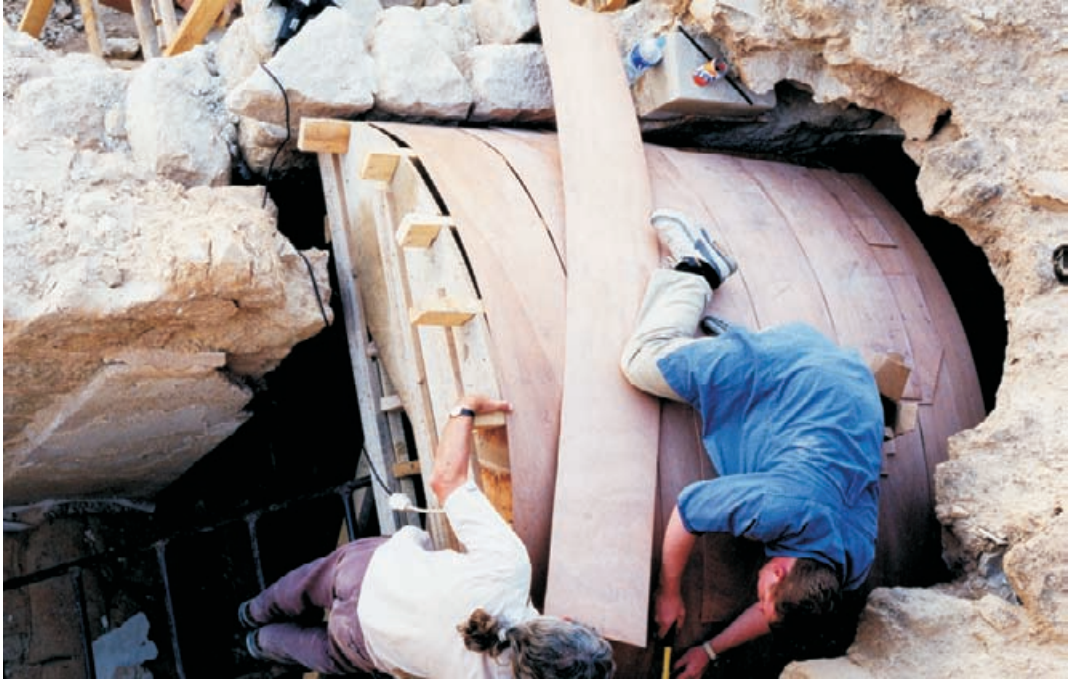
Figure 10.32 Fixing the plywood sheathing to the vault former.
