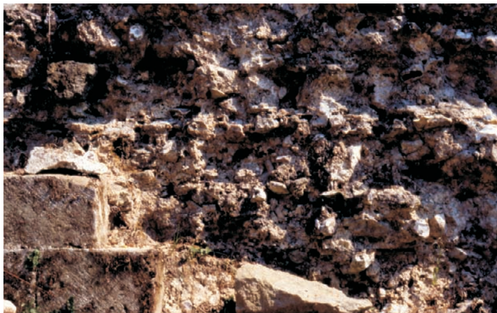
Figure 4.35 Detail of core showing the tail impressions of missing stones, with a few surviving ashlars bottom left. This evidence needs careful 'as found' consolidation to avoid losing or distorting the record. Clarendon Palace.
