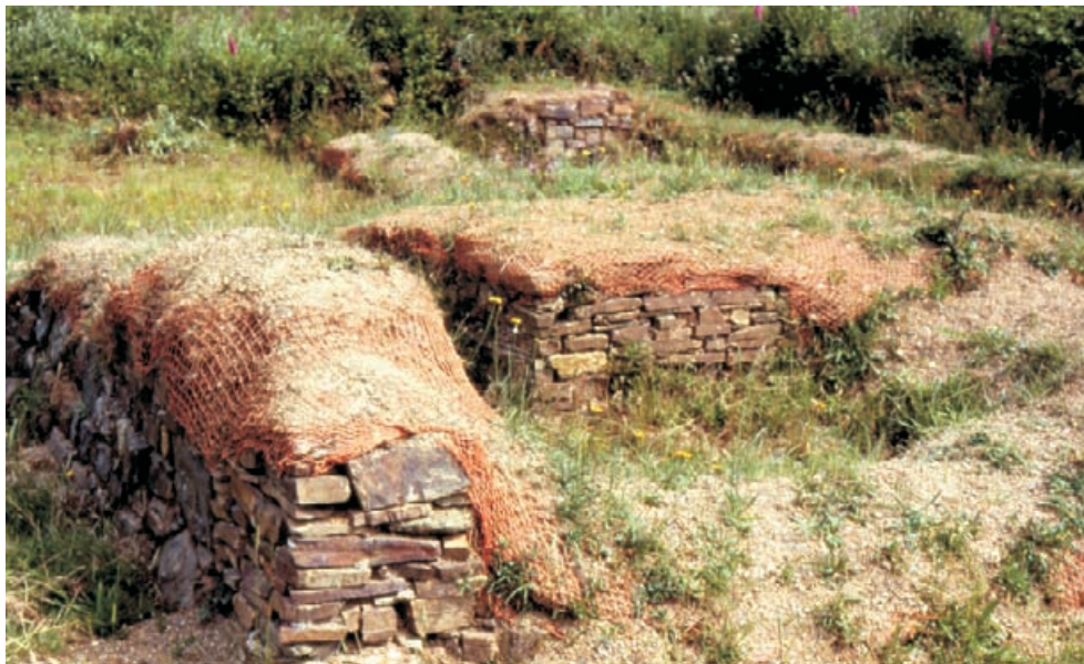
Figure 4.28 Walls built in clay mortar should not have cement or even lime-based mortar introduced as part of a consolidation process. Biodegradable net is used here to secure the loose wall heads after excavation, pegged with long plastic anchors deep into the core. In this wet area, grass and plants native to the site soon take over the wall tops again.
