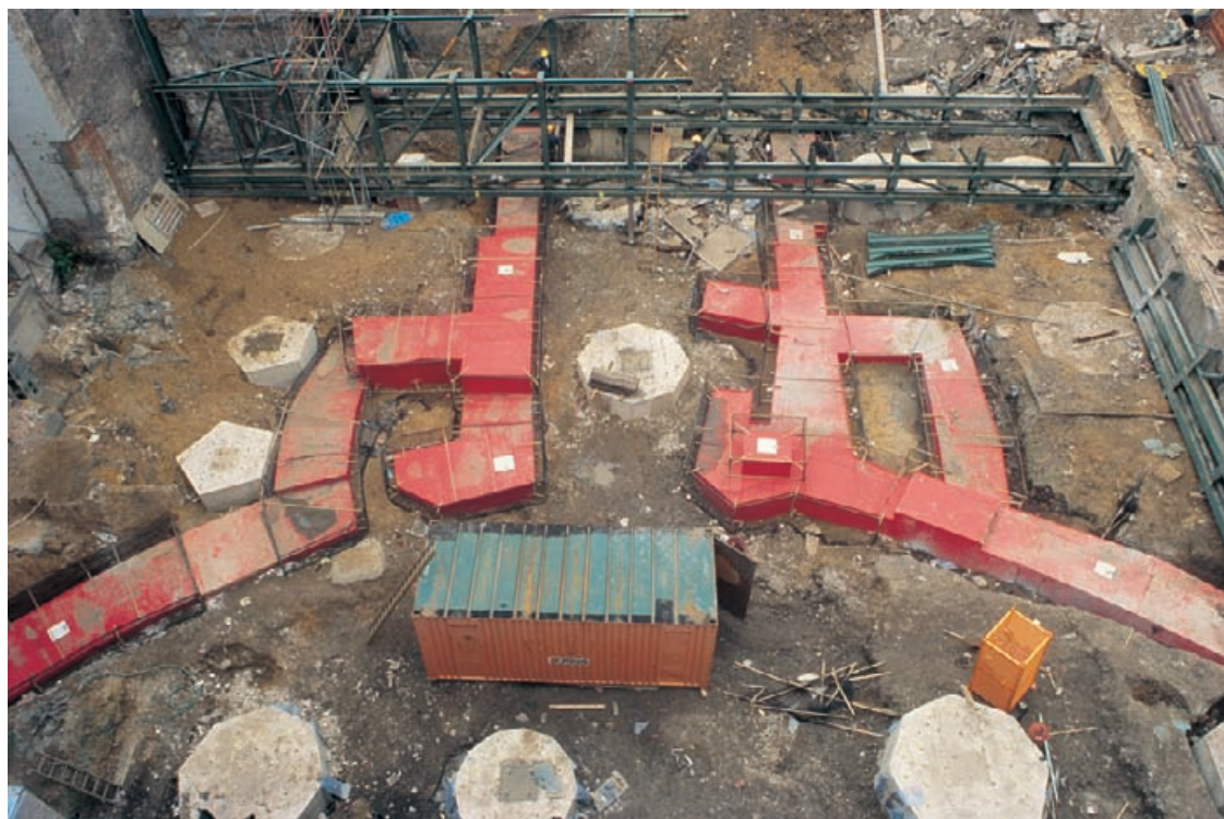
Figure 5.14 View of protected remains of the Roman amphitheatre in the course of redevelopment at the Guildhall, London (photograph courtesy of Museum of London Archaeology Service).
