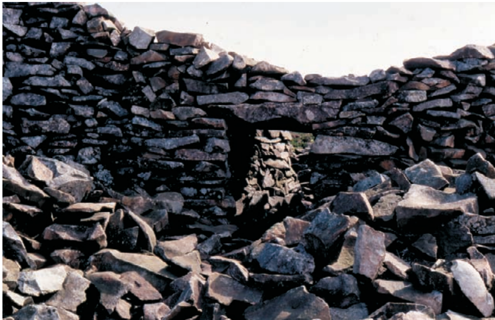
Figure 4.64 Trei'r Ceiri. Unmortared, roughly split slate walls of iron age date in Wales. The sophistication of this masonry lies not in the dressing of the stones but in the way in which they are assembled, each stone acting as a structural component and sitting comfortably within the wall. Such walls could be packed with earth and turf to make them water and wind proof, but should never be mortared in any consolidation work.
