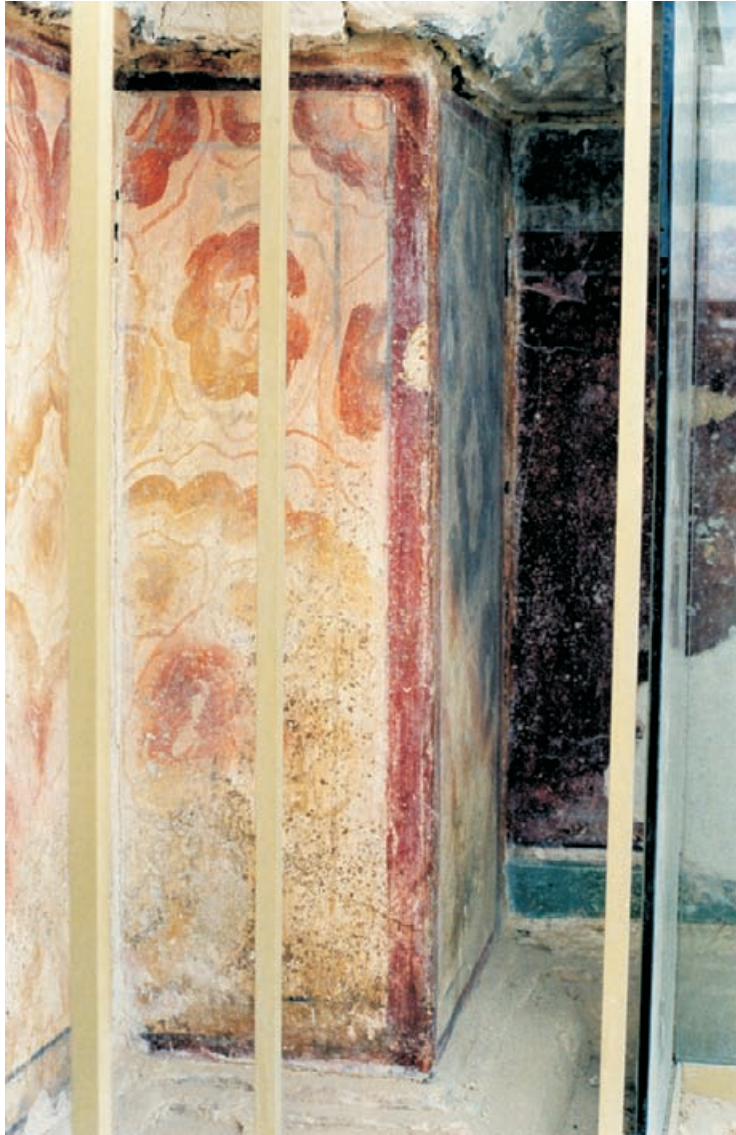
Figure 5.13 Detail of wall painting on the lower terrace at the Northern Palace, Masada in Israel, with pitting to the lower section from soluble salts (photograph: C. Woolfitt).
