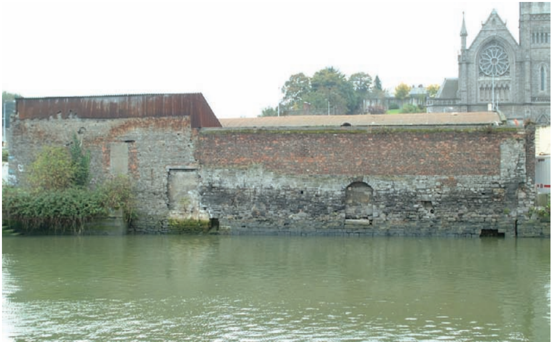
Figure 7.12 Medieval waterfront merchant's house at Drogheda on the east coast of Ireland, showing a range of conservation issues, including modern overburden, later repairs, missing and dislodged masonry, and difficulties in interpreting the character of the archaeological monument.
