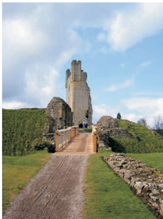
Figure 9.6 One of two sympathetic, though distinctly modern, oak bridges constructed at Helmsley Castle in Yorkshire. With much timber fabric having long since perished, the use of oak goes some way to redress the masonry: timber balance.
