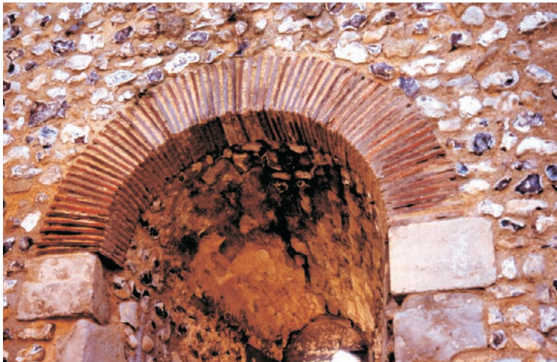
Figure 4.58 Philosophy in place at Wolvesey Castle in Winchester. Missing stones of the arch have been replaced with clay tile rings; although an effective piece of consolidation the completeness of the tile ring could be misleading, suggesting that this might originally have been a tile arch.
