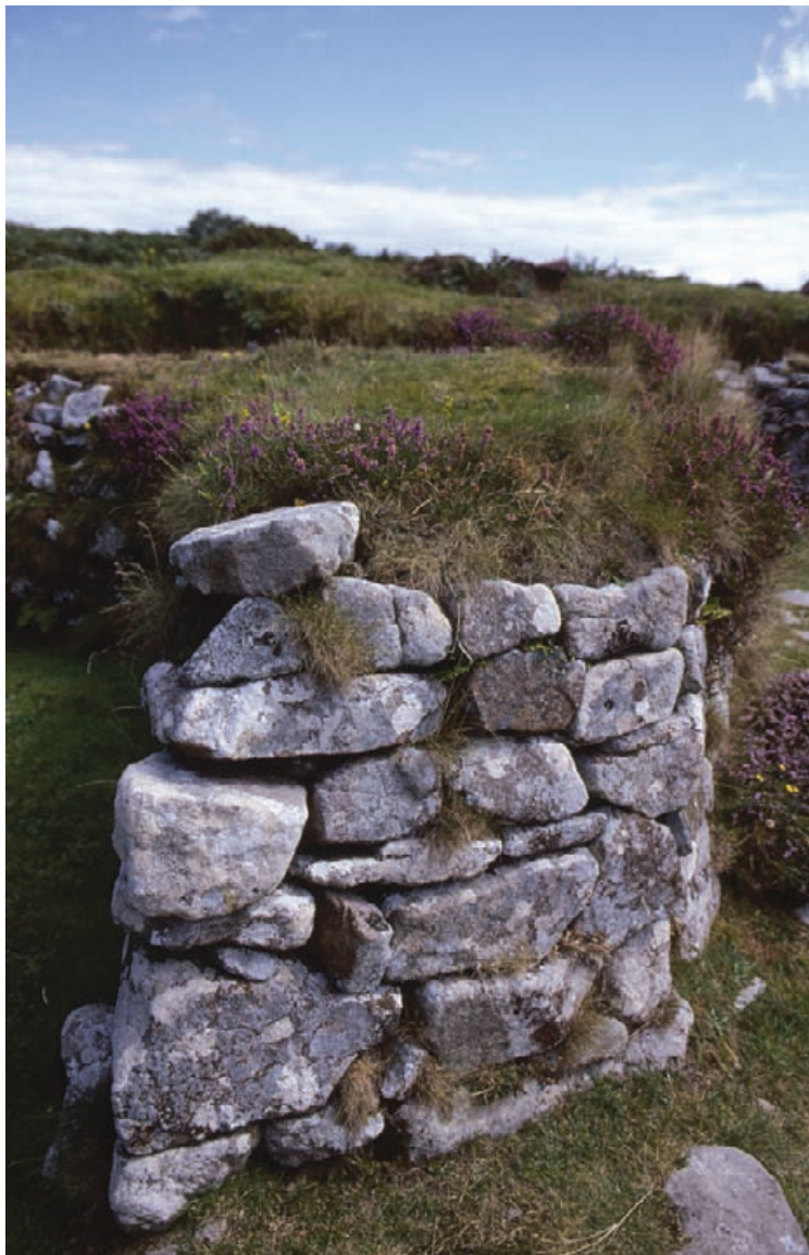
Figure 3.3 Soft wall capping has been found to be beneficial for the protection of standing wall remains, enhancing site ecology and providing a long-term, low-maintenance conservation solution.
