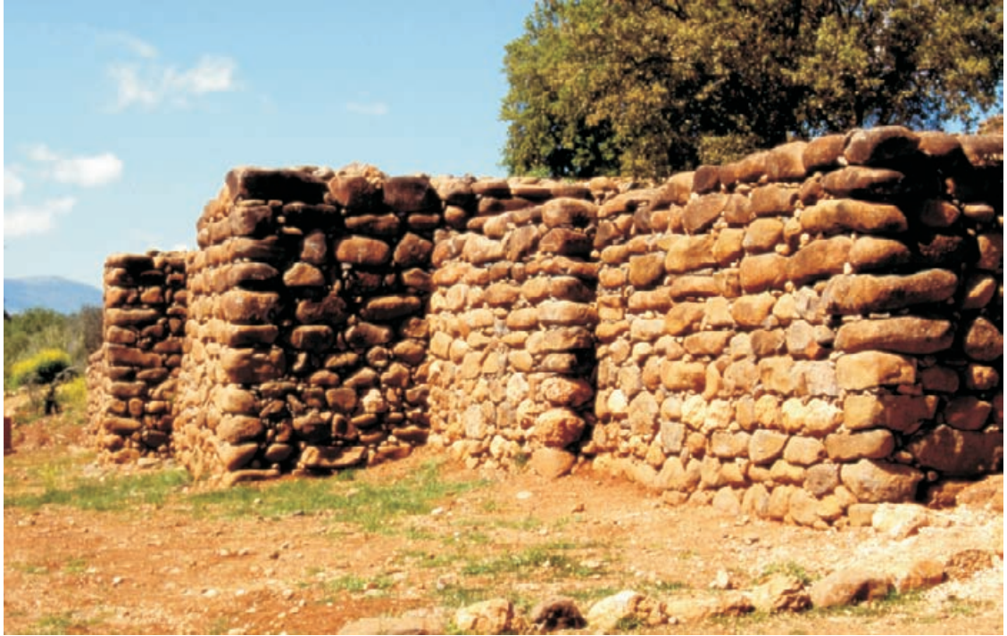
Figure 4.66 Masonry of water-washed boulders at Tel Dan, Northern Israel. Upper courses rebuilt.
