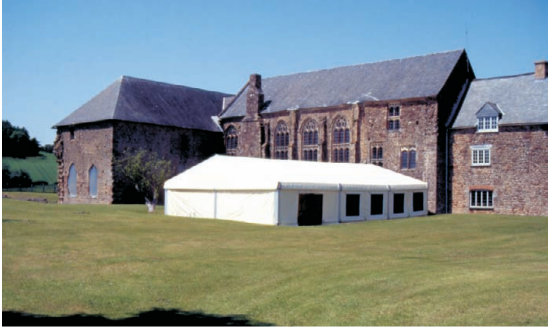
Figure 5.29 View of the tent-like shelter structure over tile pavement at Cleeve Abbey (photograph: J. Ashurst).
