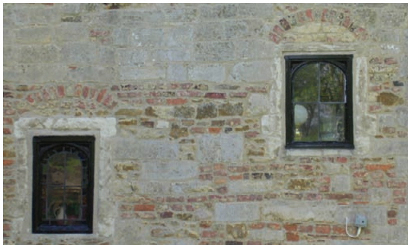
Figure 2.40 Brick relieving arches in stone masonry.
