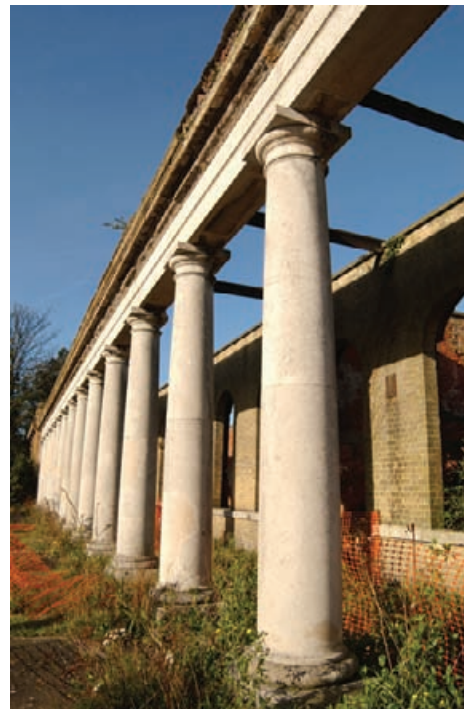
Figure 10.40 The tuscan order was used by Sir William Tite for the entrance colonnade, worked in portland stone, with scholarly detailing.
