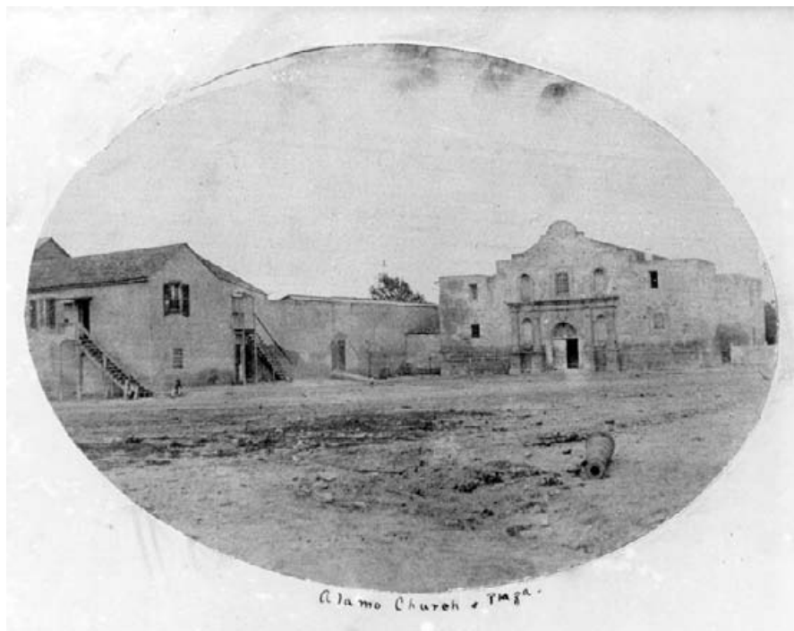
Figure A4.4 The 'Alamo Church and Plaza'. Post 1860 rebuild of the west façade of the Church building and of its roof (DRT) (Reproduced by kind permission of the Daughters of the Republic of Texas).
