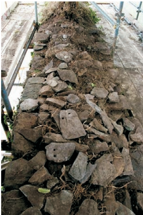
Figure 4.18 First stage clearance of ruinous wall head showing removal of vegetation and the stratification layers which confront a conservation technician.
