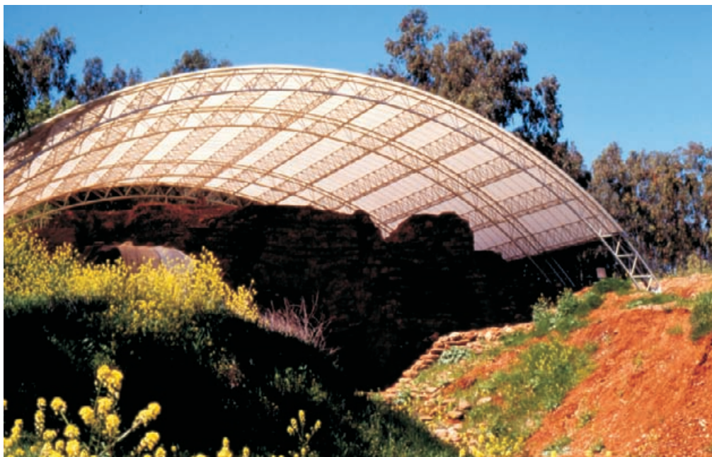
Figure 5.26 Protective shelter at Tel Dan in Israel (photograph: J. Ashurst).
