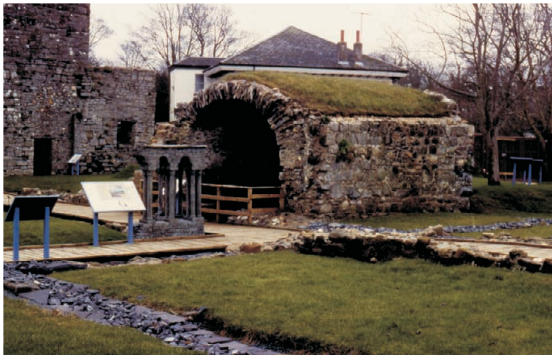
Figure 4.32 The Chapter House vault covered with humus and turf taken from the site.
