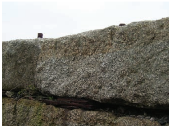
Figure 2.47 Jacking effect of thin steel packer.
