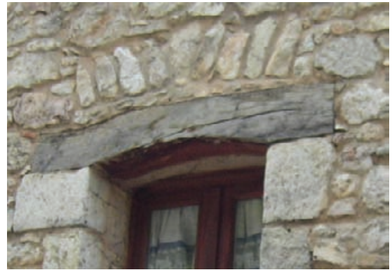
Figure 2.41 Typical relieving arch above timber lintel.
