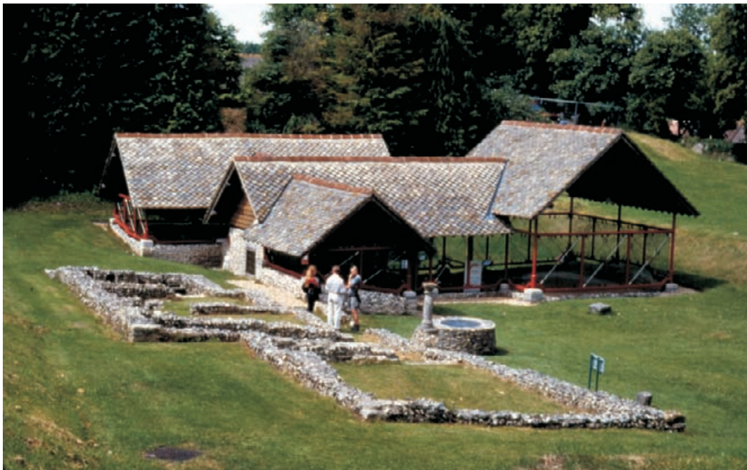
Figure 5.31 The recent protective building over the west range of the Roman Town House in Dorchester (photograph: C. Woolfitt).
