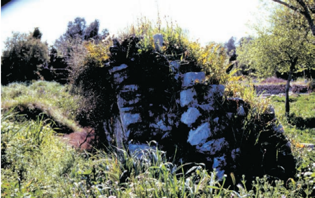
Figure 6.5 Plants thriving on the lime core and sloping surfaces of collapsed walls at Butrint, Albania. On such an extensive site, zones such as these may be left in their 'natural' condition without loss or detriment to the monument.
