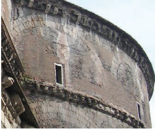
Figure 2.42 Blind arches in the walls of the Pantheon.
