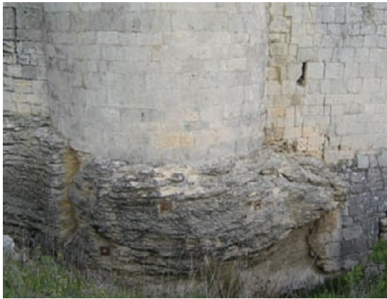
Figure 2.60 Rock bolting at Chateau de Lacoste.
