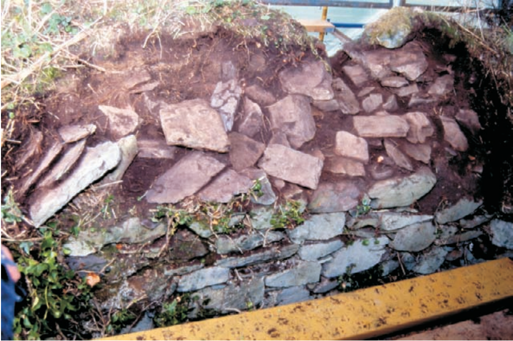
Figure 4.18 First stage clearance of ruinous wall head showing removal of vegetation and the stratification layers which confront a conservation technician.
