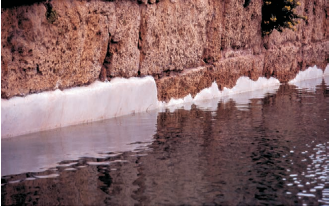
Figure 10.27 Detail of new water-holding plaster applied by Kimi Maman to the restored Herodian dam above Caesarea. The plaster copies that of the Roman period.
