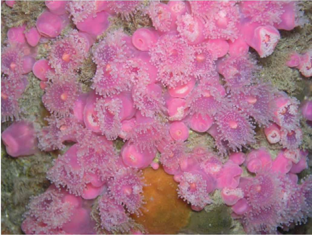
Figure 7.7 Submerged masonry surfaces can be obscured by extensive marine growth (e.g. the jewel anemone ( Corynactis viridis ) which may have other heritage values. Courtesy of Rebecca Morris.
