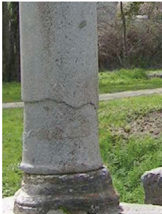
Figure 2.15 Granite column showing temperature-related ‘onion-peeling’.
