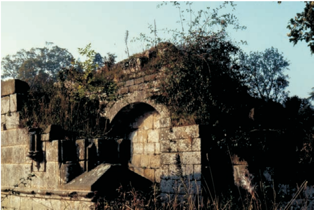
Figure 6.6 Wall cover at Jervaulx Abbey, UK, including wild roses, is an undeniable asset to the site, but needs to be controlled to allow adequate stabilisation and masonry maintenance to be carried out.
