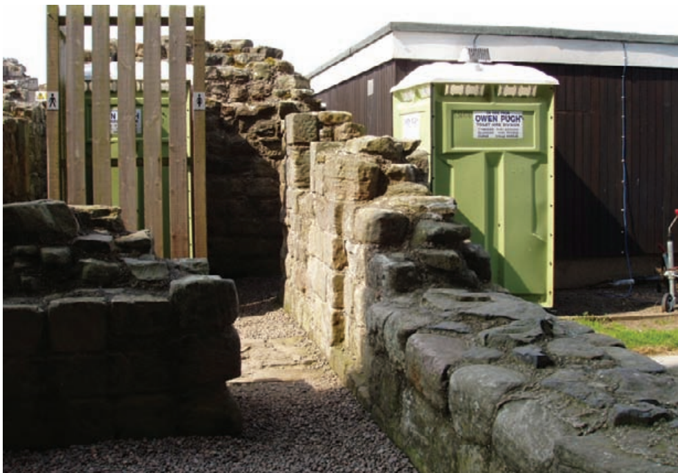
Figure 9.8 The proximity of services, such as portable toilets, to historic fabric can have a seriously adverse effect on enjoyment of a site.
