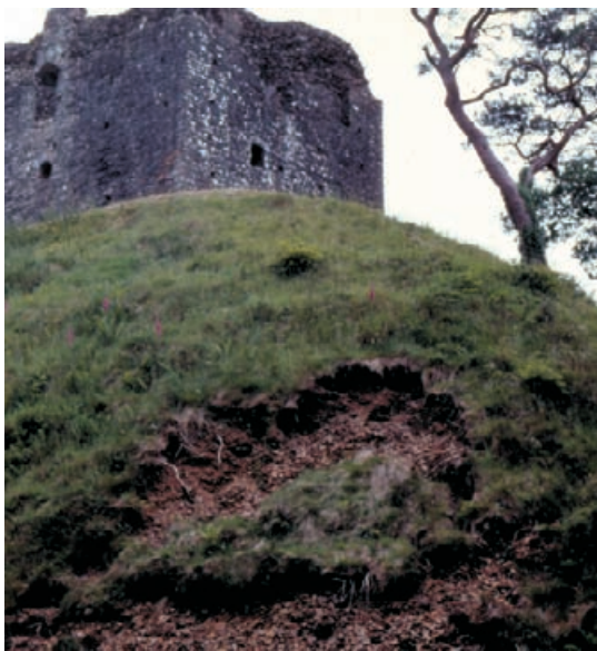
Figure 4.67 The Medieval earth motte of Okehampton Castle, UK, showing earth slippage after heavy rain, exacerbated by burrowing rabbits. Turf repairs are appropriate, cutting into the mound and laying turfs as bonded blocks with staggered joints. Synthetic rope land mesh can be pegged across the repair until the grass is established.
