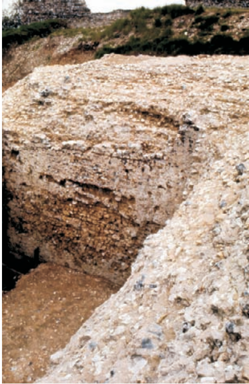
Figure 4.16 Core facework, especially that exposed at wall heads, and even buried core are particularly susceptible to binder dissolution and migration in very wet conditions, especially at low temperatures (see Appendix). The design of replacement mortar for these conditions is clearly important. Non-hydraulic or weakly hydraulic mortars are too vulnerable and may never carbonate satisfactorily in persistently wet conditions. Moderately or even eminently hydraulic lime may be needed. But if the original material is too weak for such binders a weak mortar with soil and turf capping should be used. Face core work at Castle Acre Castle.
