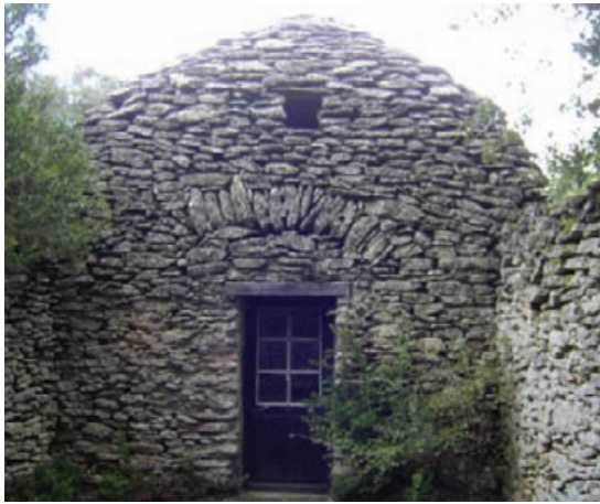
Figure 2.39 Relieving arch in dry-stone borie.
