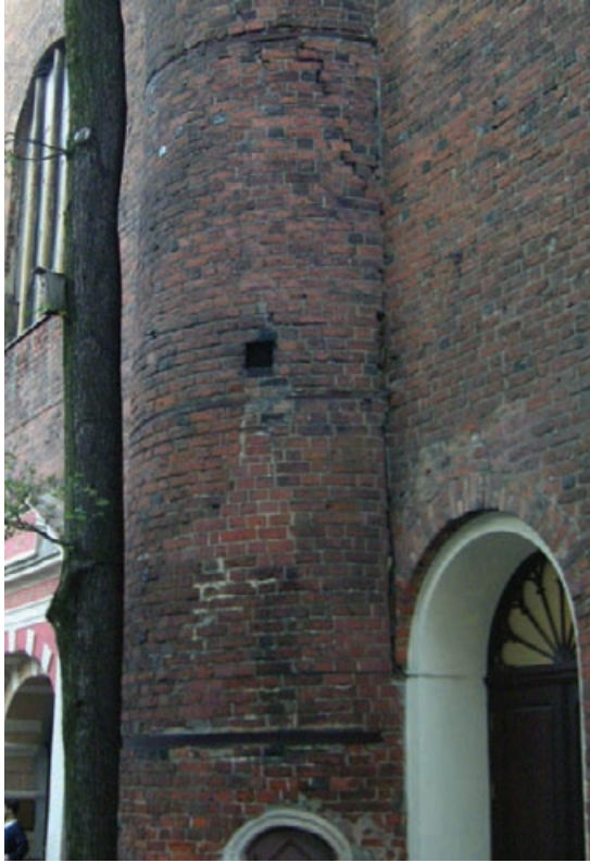
Figure 2.62 Steel tie bands, Riga Old Town.
