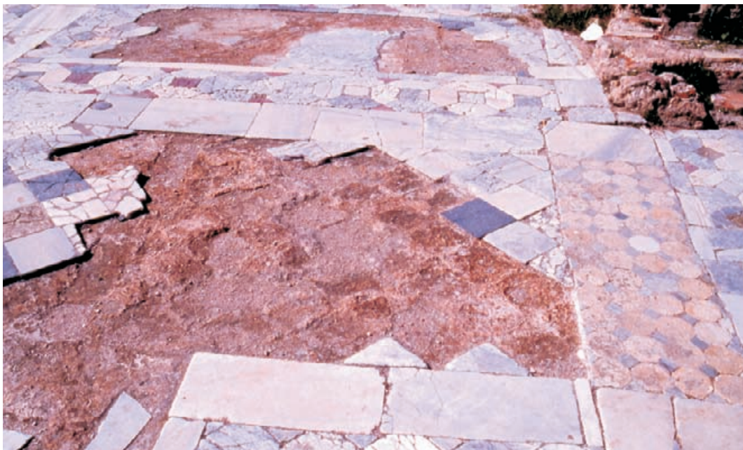
Figure 5.9 Section of ancient opus sectile pavement suffering gradual loss from visitor traffic and exposure; imprints of missing stones are visible (photograph: C. Woolfitt).
