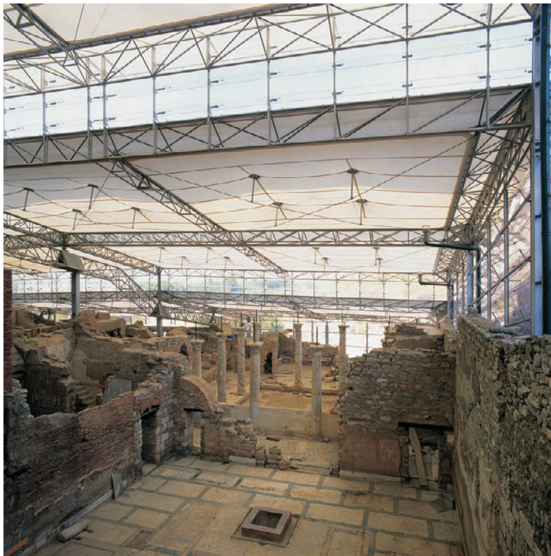
Figure 5.28 Interior of the new enclosure at Ephesus, with translucent roof and wall cover (photograph courtesy of the Austrian Archaeological Institute).
