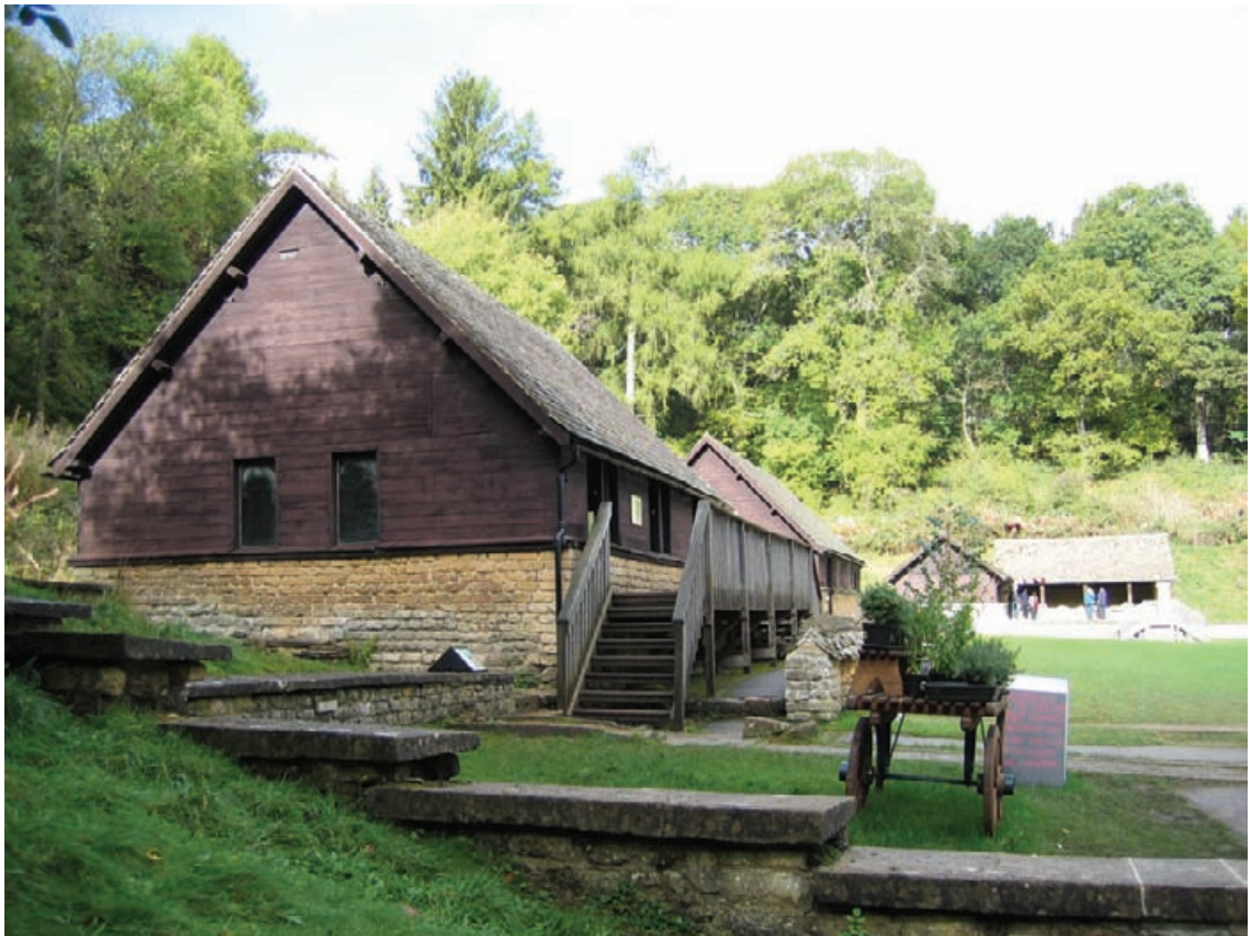
Figure 5.21 View of nineteenth century enclosure buildings over the remains of a wing of the Roman villa at Chedworth (photograph: C. Woolfitt).
