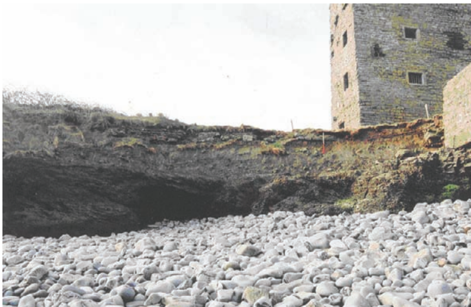
Figure 7.10 The inter-tidal area below Carrigaholt Castle, Clare on the west coast of Ireland showing a highly mobile erasive cobble beach. The sub-surface remains of a now-lost gabled house can be seen in the cliff edge, now within 3 metres of the tower.
