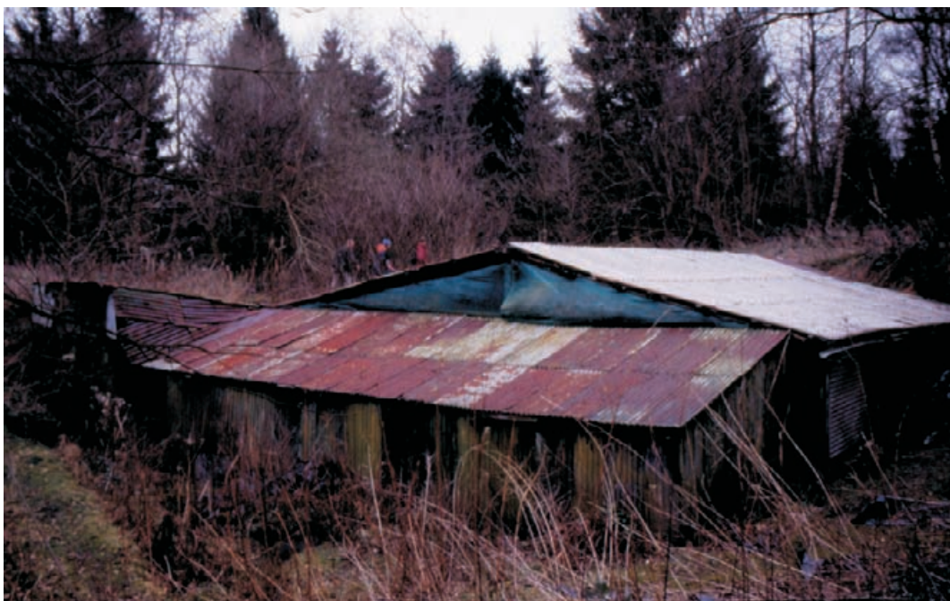
Figure 5.32 Temporary shelter over Roman remains situated in a natural depression in the landscape (photograph: C. Woolfitt).
