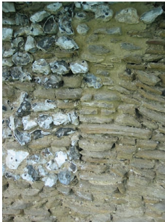
Figure 10.9 Detail of line of crenellated parapet on south elevation, with Bargate rubble construction of merlon on the right and infill of embrasure in flint on the left.
