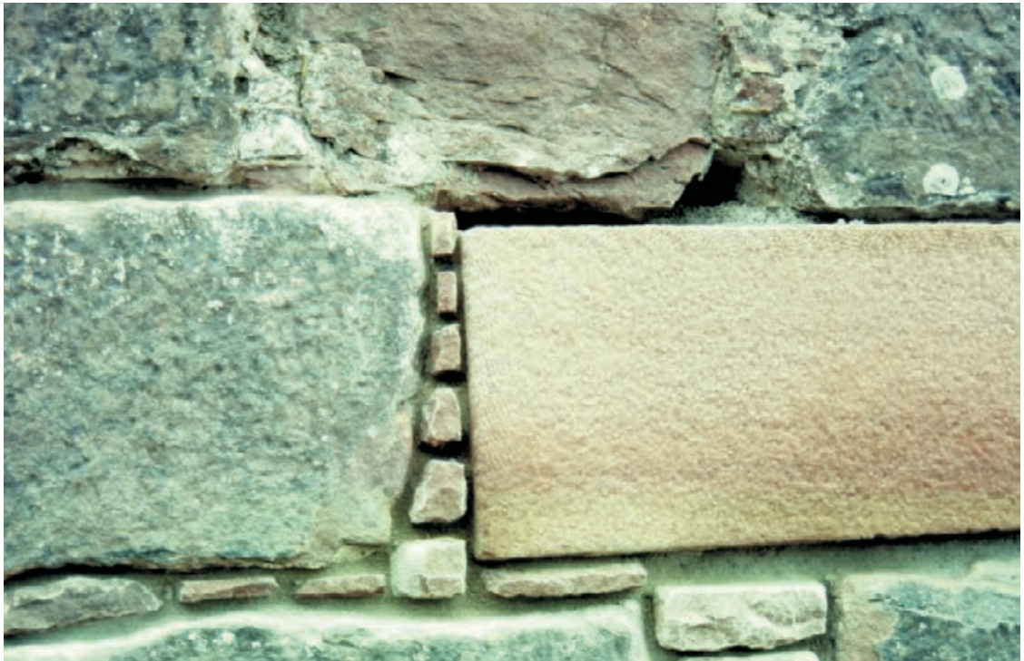
Figure 4.51 Uncomfortable machine cut replacement stone in an eighteenth century context of quarry-dressed stones.
