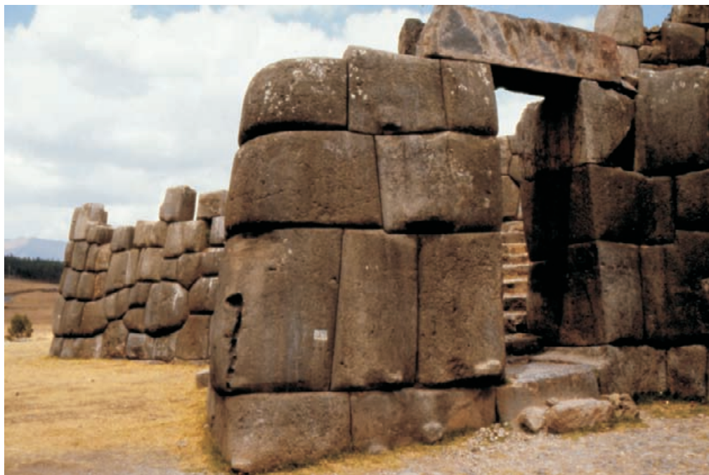
Figure 4.65 Massive, un-mortared stones as Cuzco illustrate some of the most accurately worked masonry seen anywhere, and virtually indestructible except through severe seismic activity, deliberate demolition or artillery fire.
