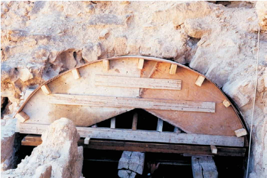
Figure 10.33 Completed formwork raised up into position under the old work.
