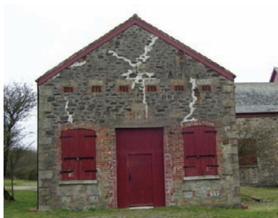
Figure 2.48 Cracking due to corrosion of a steel gantry beam.
