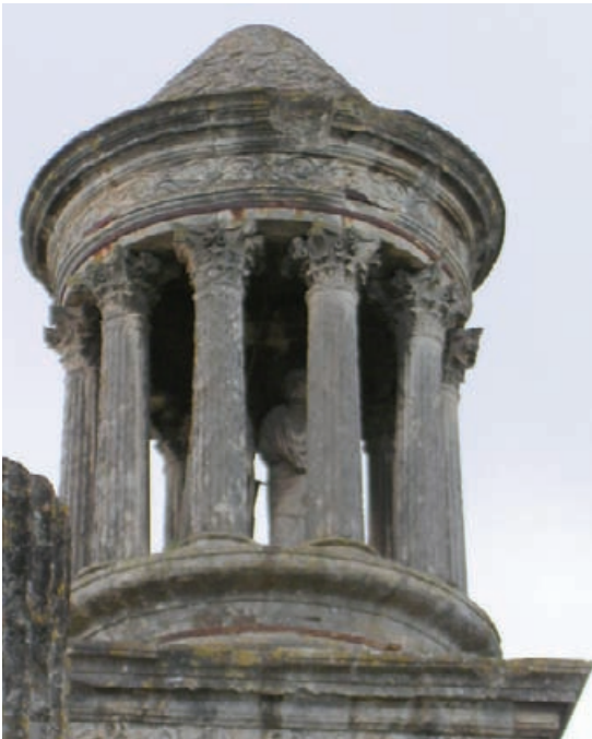
Figure 2.57 Iron girding bands, St Remy.
