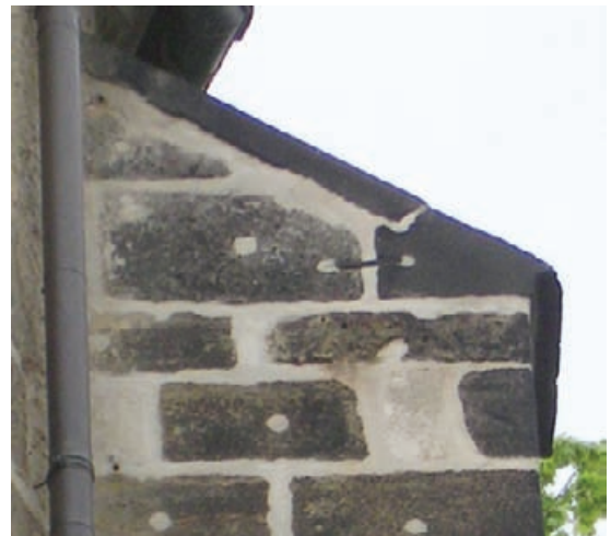
Figure 2.55 Cramps left in place post-grouting, Saxony.
