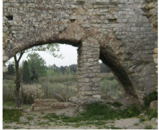
Figure 2.61 'Temporary' masonry support.
