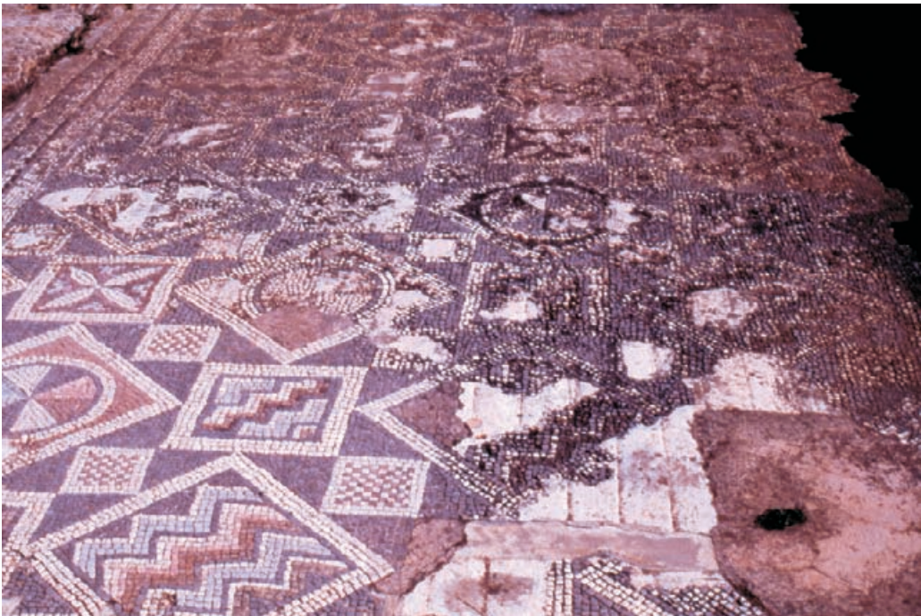
Figure 5.12 Exposed Byzantine mosaic pavement, with the pattern of water ponding and saturation reflected in the organic growth (photograph: C. Woolfitt).
