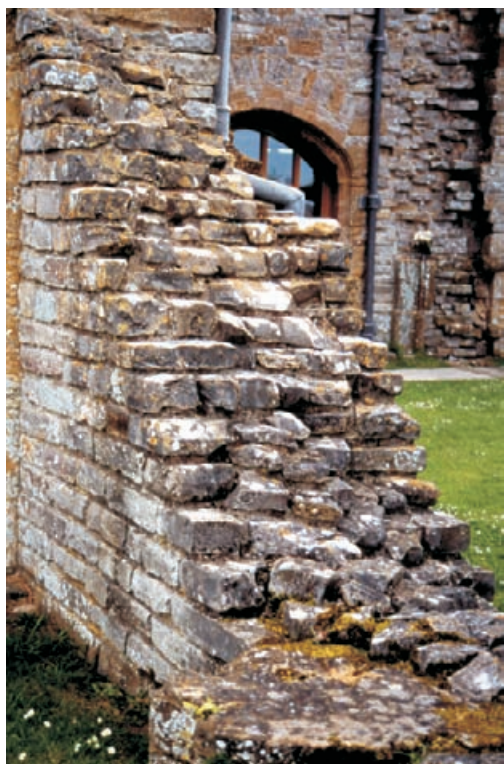
Figure 9.3 (a) An example of 'rough racking', a favoured treatment by the Ministry of Works (UK) in the first half of the twentieth century for broken wall ends and heads, used selectively at Muchelney Abbey to denote post twelfth century work.
