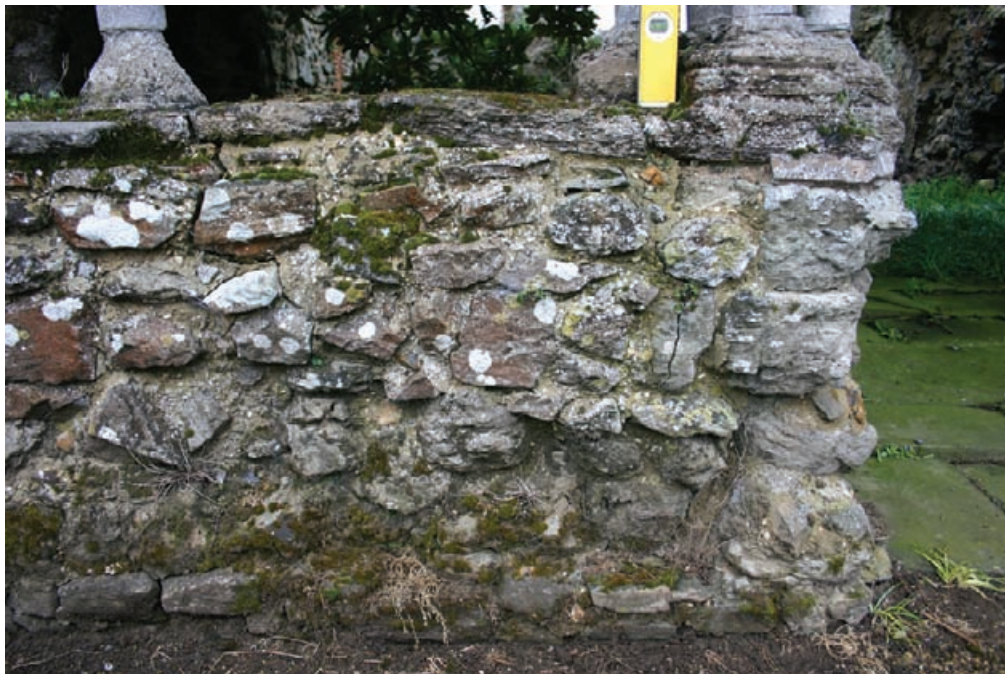
Figure 4.45 Detail of base of column cluster seen in Figure 4.44 showing the distorted and fractured support wall. Temporary supports of the arcade are required to enable the wall to be recorded, taken down and rebuilt in hydraulic lime mortar. Stitching of such poor construction is inadvisable because of lack of adequate anchorage.
