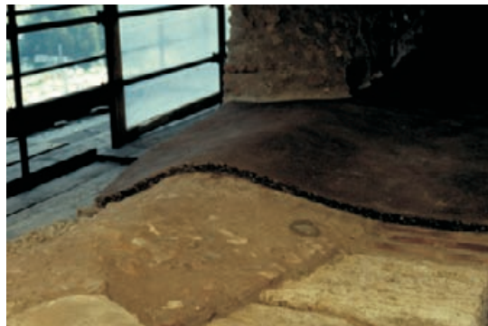
Figure 4.76 An unusual reversible wall capping system seen on the so-called 'Temple of Saturn' in the Forum of Rome, which is designed to protect the archaeology of the wall head. This is a multi-layer lime-pozzolana plaster which is designed to provide a weathering surface but which can easily be broken off in the future without damage to the original substrate.
