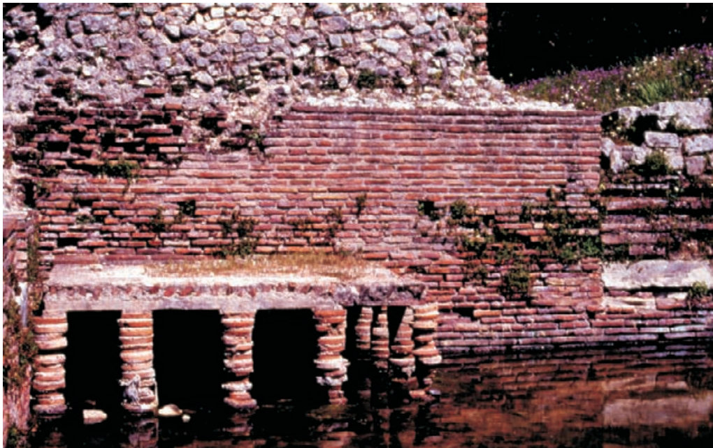
Figure 6.8 Flooded area of hypocaust, Butrint, now home to terrapins, requires draining if soluble salt damage to pilae is to be addressed. Alternative flooded zones with less sensitive fabric can be used for relocation.
