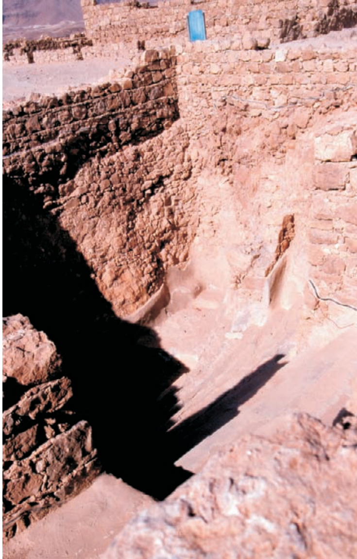
Figure 5.8 At Masada in Israel a black line through masonry joints is used to delineate rebuilt masonry from the original (photograph: J. Ashurst).
