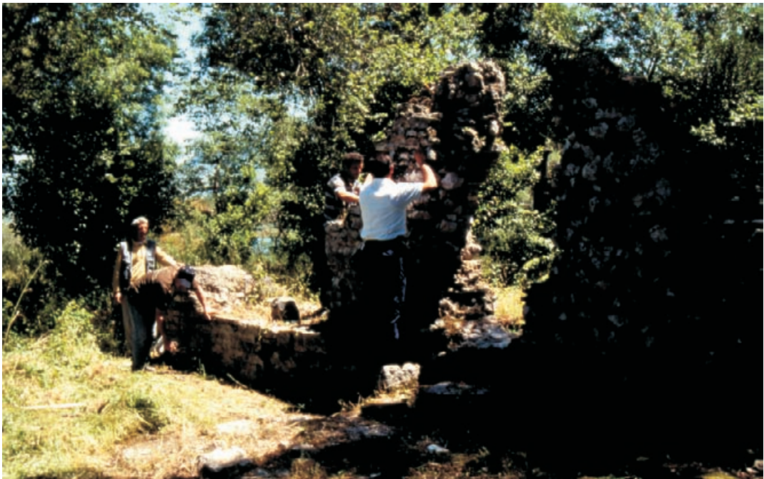
Figure 8.5 Site training on the 'Venetian' House, Butrint, Albania. First-stage site recording and assessment.
