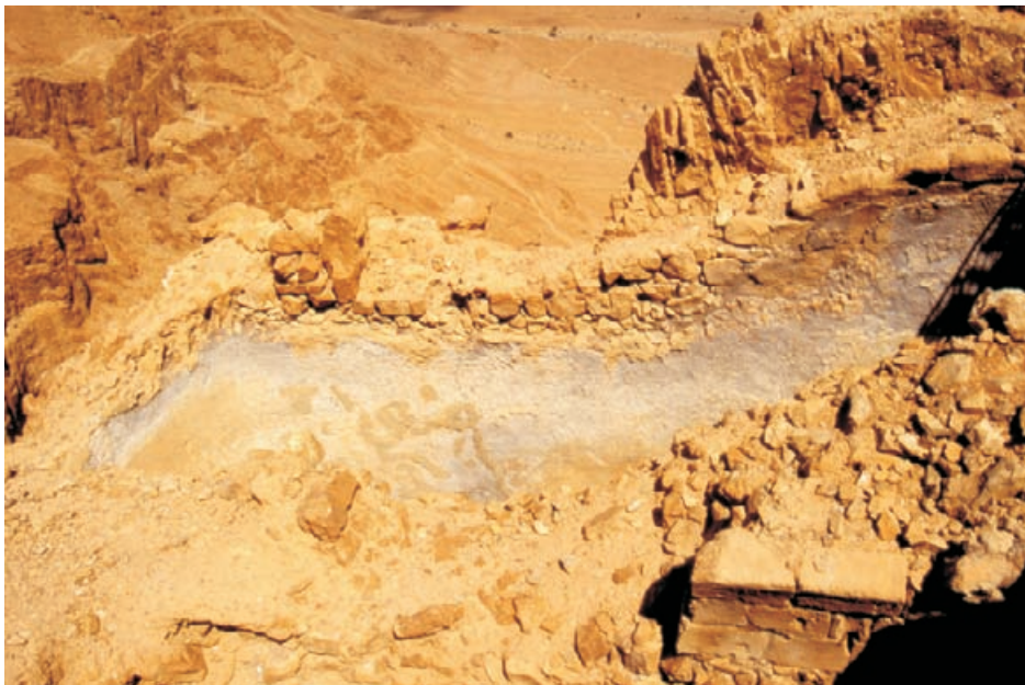
Figure 10.25 Herodian plaster lining to the artificial gutters running around the mountain to collect water and deliver it into rock-cut cisterns.
