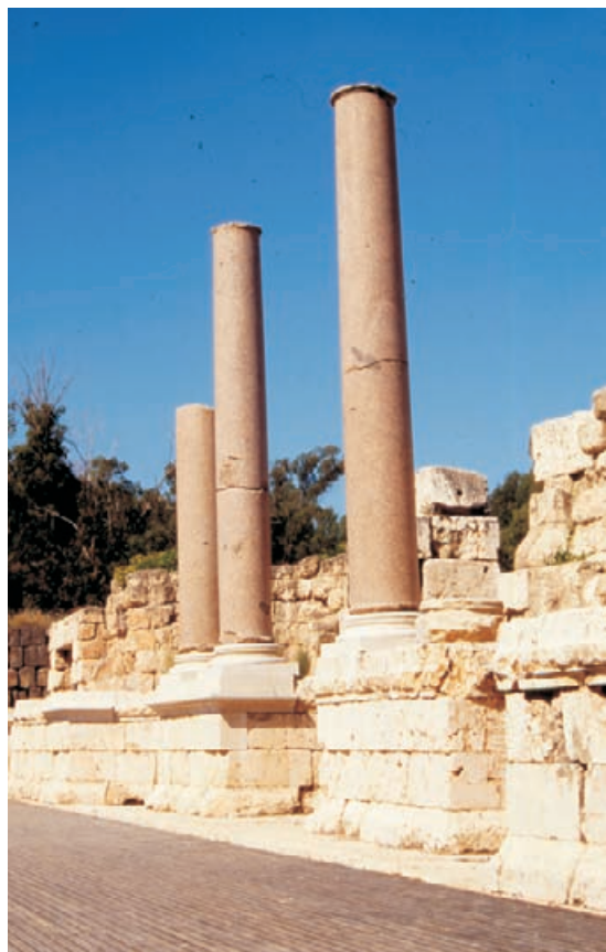
Figure 9.5 Anastylosis at Beth Shean, with re-erected columns recovered from their fallen positions in the street below (but see comments in Chapter 1, page 23, on Tall elements repaired with reinforcing rods set in resin).
