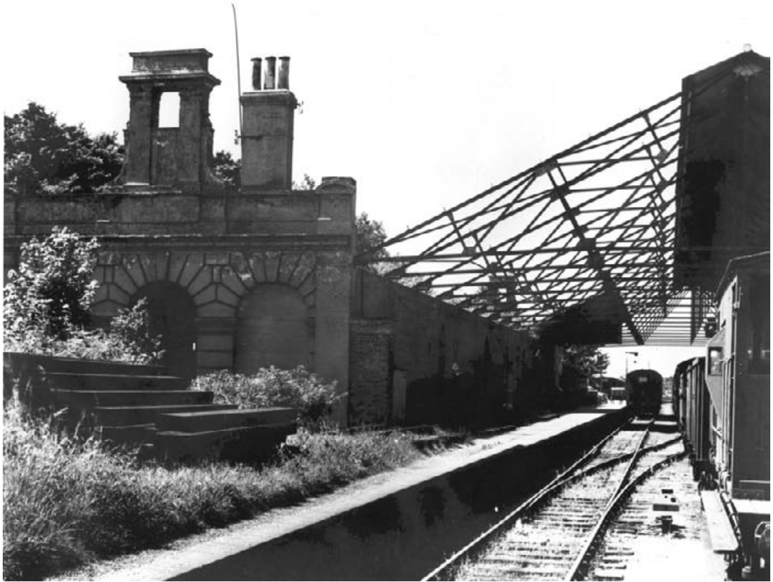
Figure 10.36 Hillspan roof installed after the original timber roof was destroyed by enemy action in 1941.
