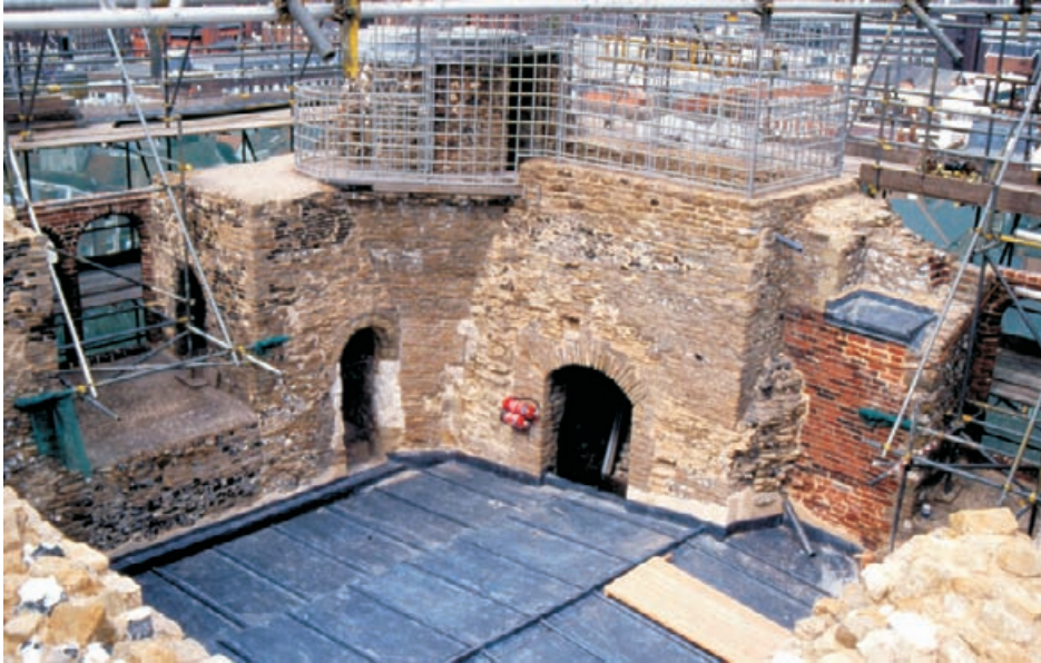
Figure 10.12 View of new lead covered roof, looking north-west.
