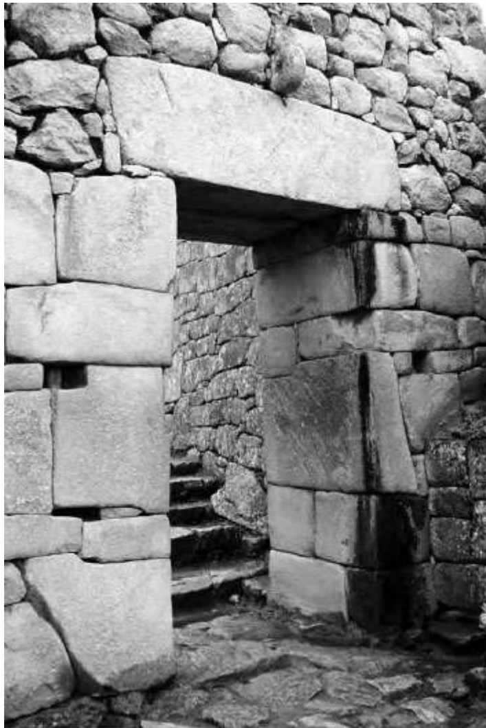
A megalithic door at Machu Picchu with small reconstructed stones above it.
