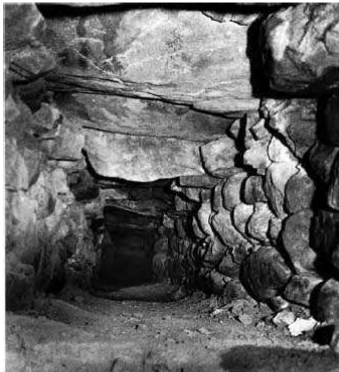
Megalithic drainage tunnel at Chavin, part of the washing of ores?
