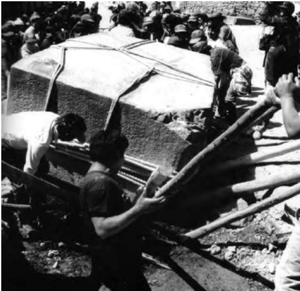
A photo of the 2004 effort to move a large stone at Ollantaytambo with ropes and levers.
