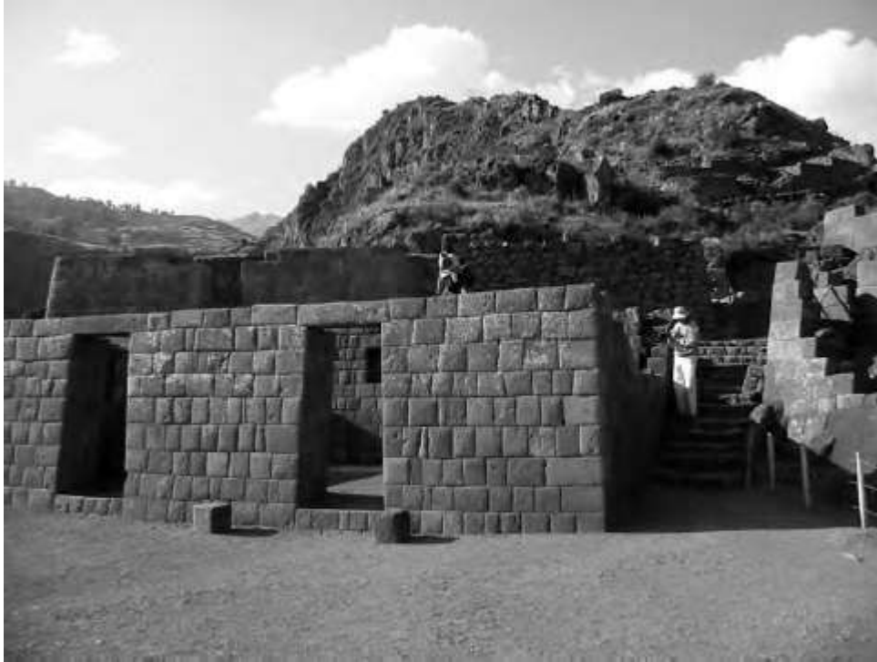
The smaller but finely fitted so-called “Royal Inca” construction, seen here at Pisac.
