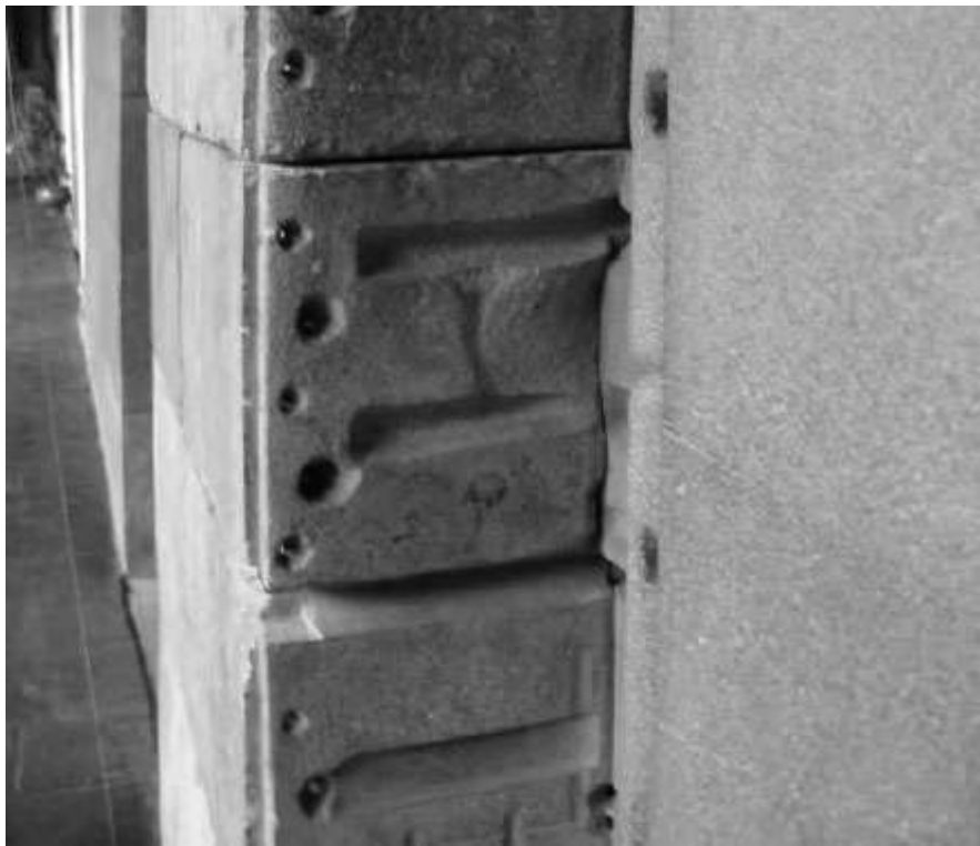
Two close-up photos of the drill holes in the articulated doorway at the Qoricancha.
