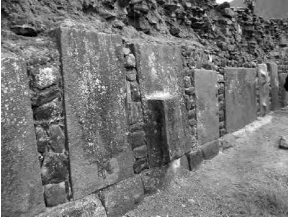
Massive blocks on the megalithic side of Ouantaytambo used in later construction with crude stones used as fill.
