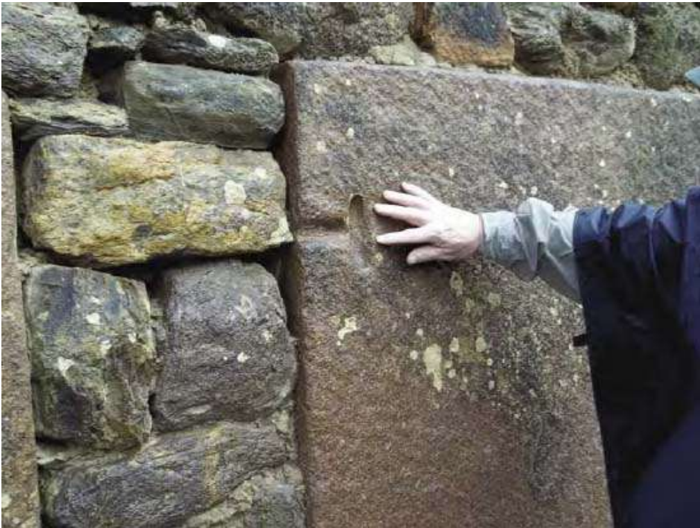
A large block on the west side of the Sun Temple of Ollantaytambo with a vertical keystone cut.
