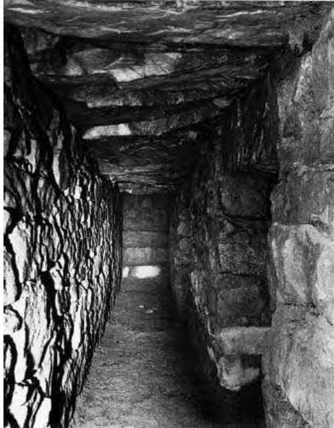
Gallery tunnel under the New Temple at Chavin, part of an extensive network of channels.
