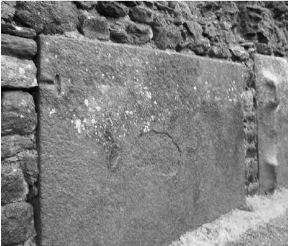
A portion of the wall at Ollantaytambo with a keystone cut in a vertical position.
