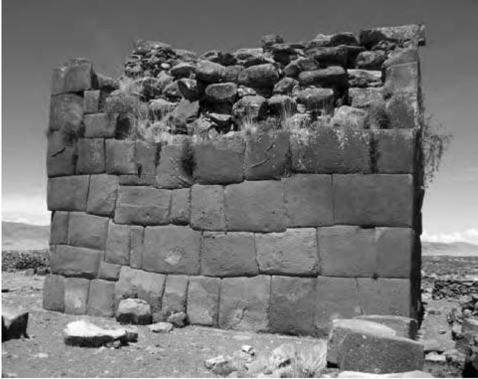
The square tower with a snake cut into the corner at Cutimbo.
