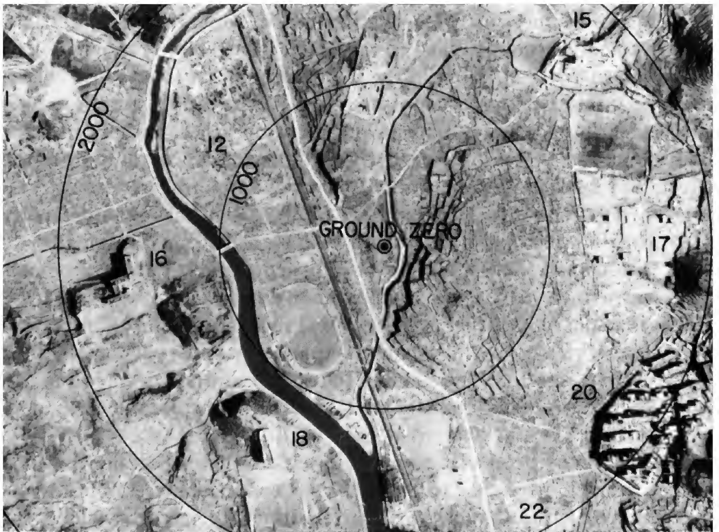
Area around ground zero at Nagasaki before and after explosion (1,000-foot radius circles are shown).
