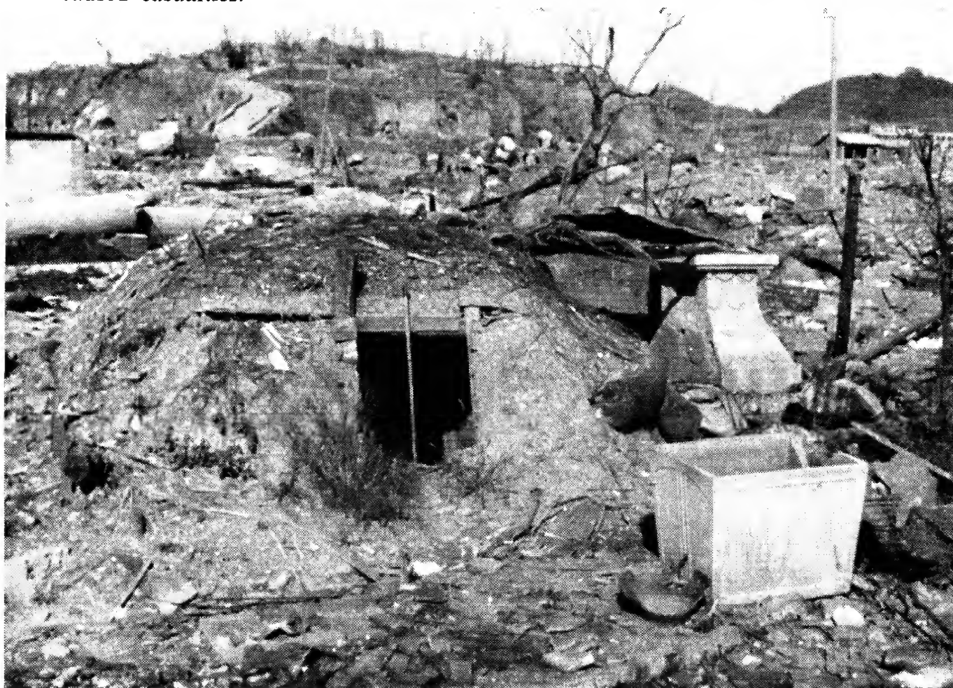
Photo No. 18. NAGASAKI. Typical small earth-covered back yard shelter with crude wooden frame, less than 100 yds. from the centre of damage, which is to the right. There was a large number of such shelters, but whereas nearly all those as close as this one had their roofs forced in, only half were damaged at 300 yds., and practically none at half a mile from the centre of damage.
