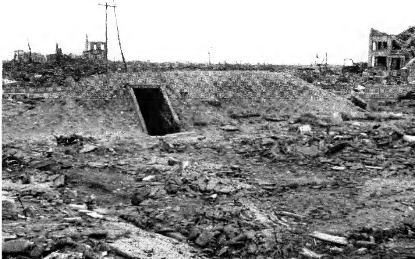
Photo No. 17. HIROSHIMA. Typical, part below ground, earth-covered, timber framed shelter 300 yds. from the centre of damage, which is to the right. In common with similar but fully sunk shelters, none appeared to have been structurally damaged by the blast. Exposed woodwork was liable to "flashburn." Internal blast probably threw the occupants about, and gamma rays may have caused casualties.
