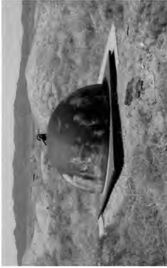
Shelter at ground zero, directly under 11 kt Fizeau nuclear explosion (500 ft tower)
