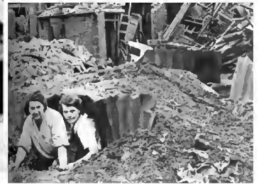
Proof that the Anderson garden shelter could withstand a house collapsing on it can be seen in this picture. Mr. and Mrs. Clague bless their insistence on 'going to ground' when their homes and those of their neighbours were reduced to rubble.
