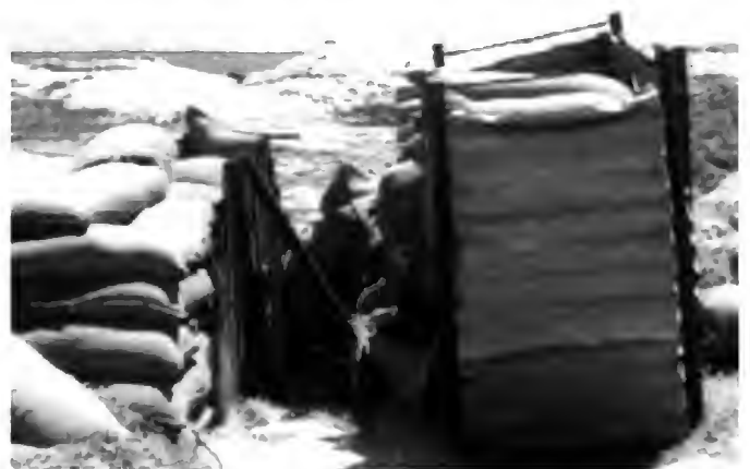
Left: Fig. 12.3, Andersons at 1800 ft after burst. Right: Fig. 12.4, Andersons protected by blast walls at 2760 ft.
