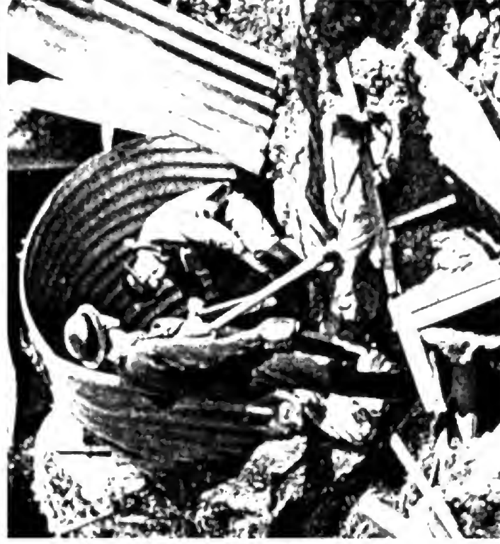
Anderson shelters absorbed the blast energy and were damaged, saving lives.
