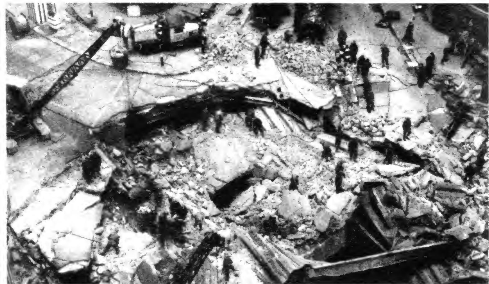
ENORMOUS CRATERS. At the Bank, where the road collapsed into the subway beneath. A temporary bridge was thrown right across it.
