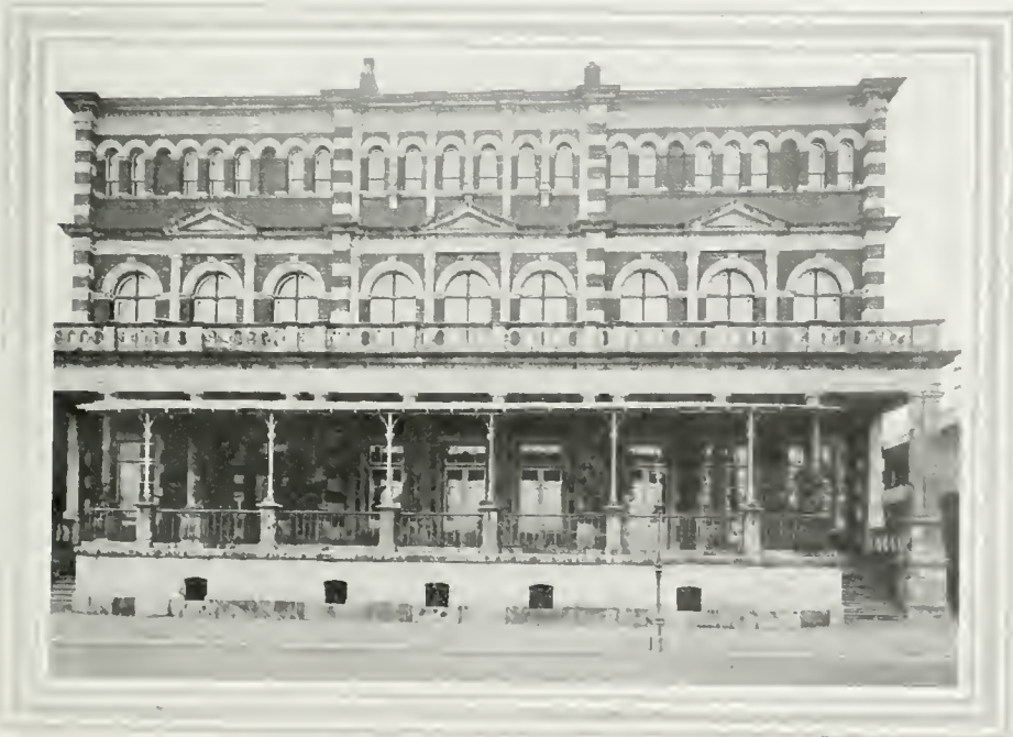
THE YOKOHAMA UNITED CLUB, ON THE BUND
