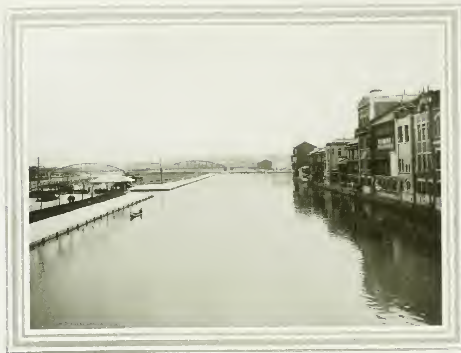
TENJINBASHI BRIDGE, FROM SHIN-NANIWA-BASHI BRIDGE, OSAKA
