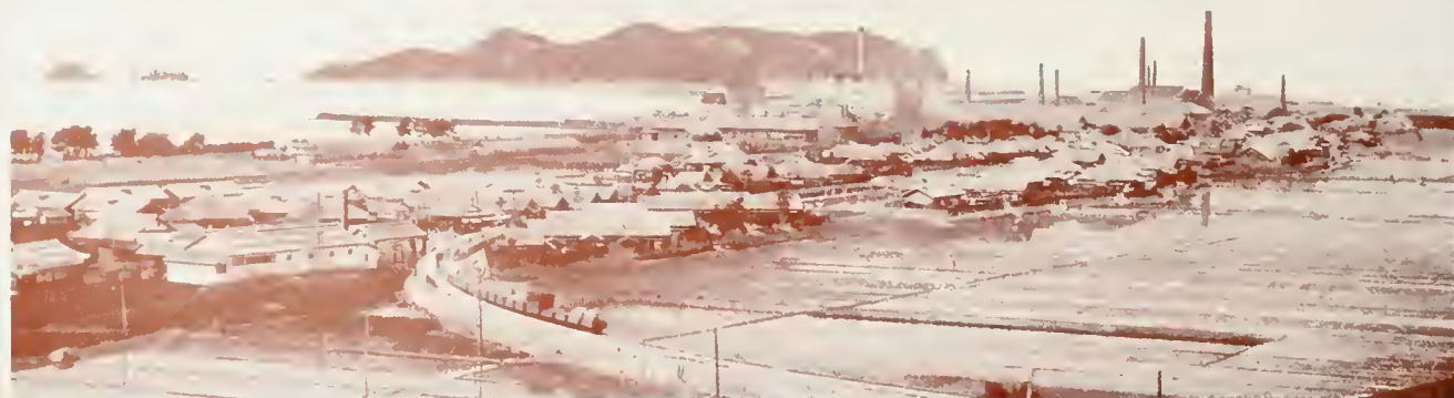
SUMITOMO COMPANY: VIEW OF THE TREATMENT WORKS IN CONNECTION WITH THE BESSHI COPPER MINE, AT NIHAMA
