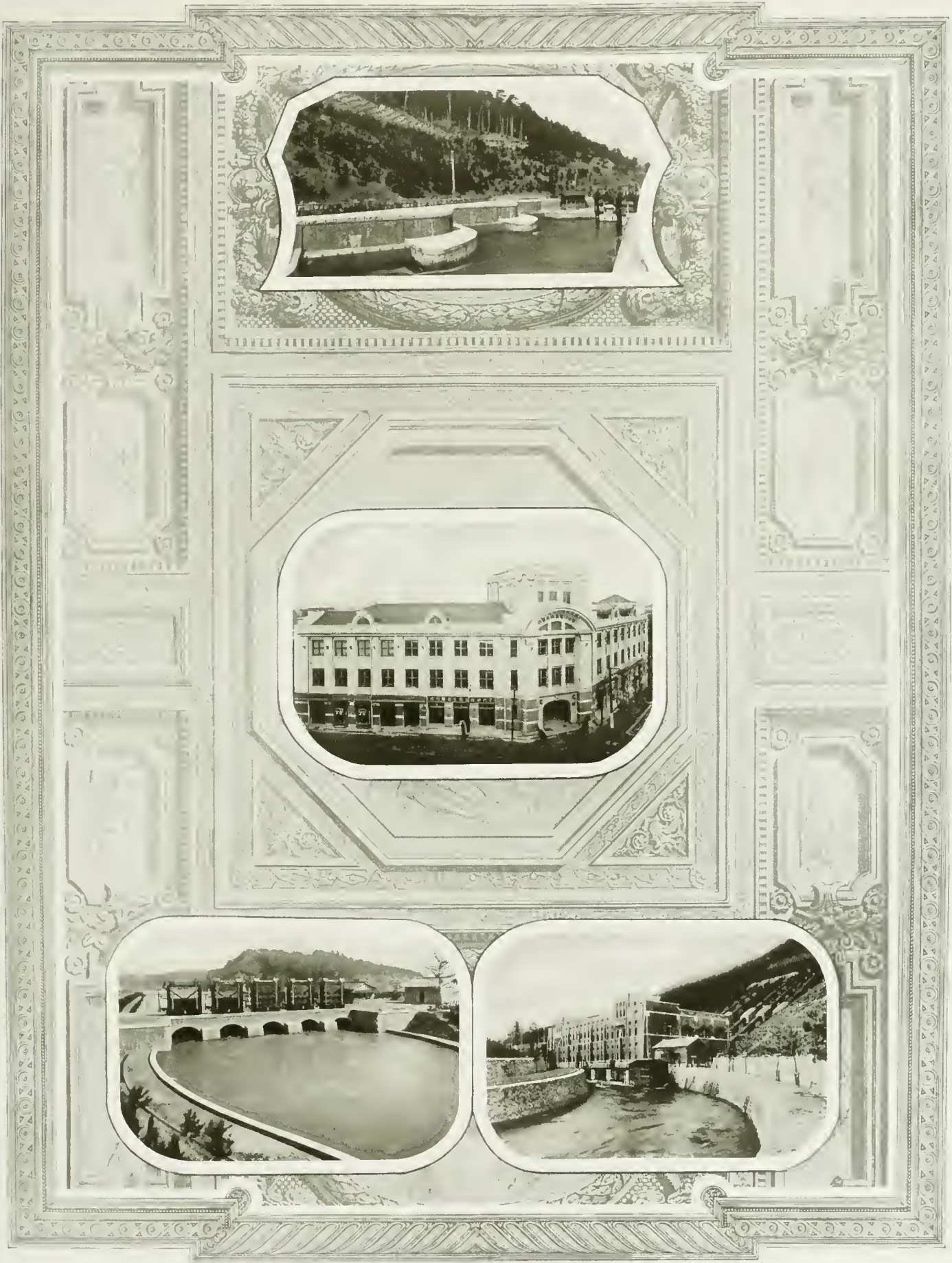
UJIGAWA ELECTRIC CO., LTD.: THE OVERFLOW — THE OSAKA OFFICES — THE REGULATOR GATES — UJI POWER HOUSE
