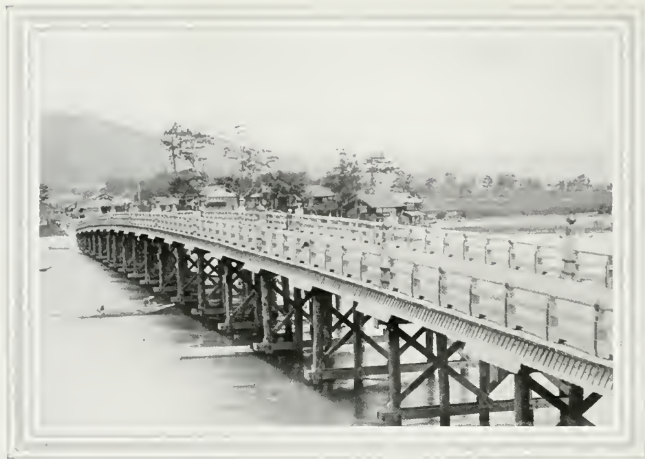
A JAPANESE BRIDGE OF THE OLD STYLE, AT SHIMOGAMO
