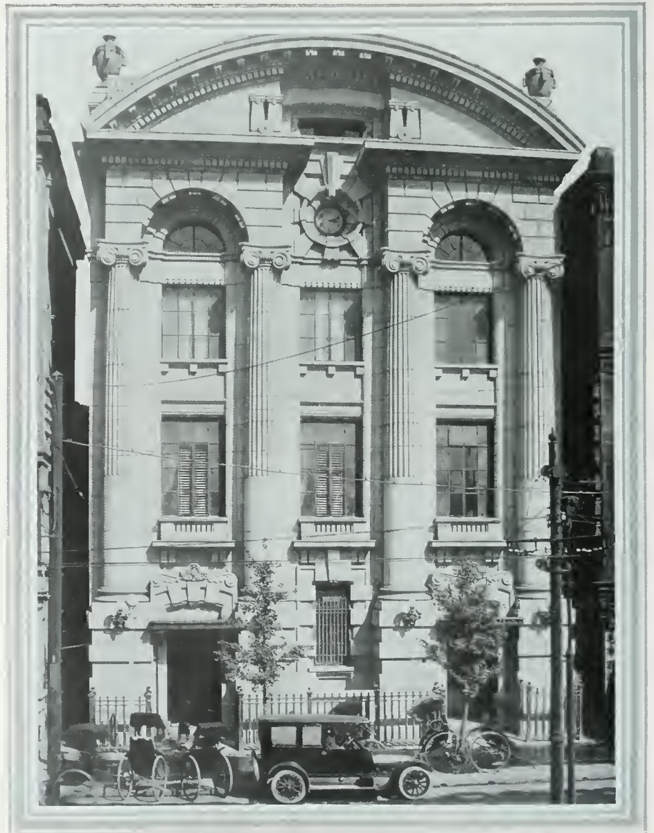
PREMISES OF MORIMURA BANK, TOKYO
