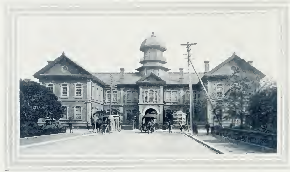
THE IMPERIAL CUSTOM HOUSE, YOKOHAMA
