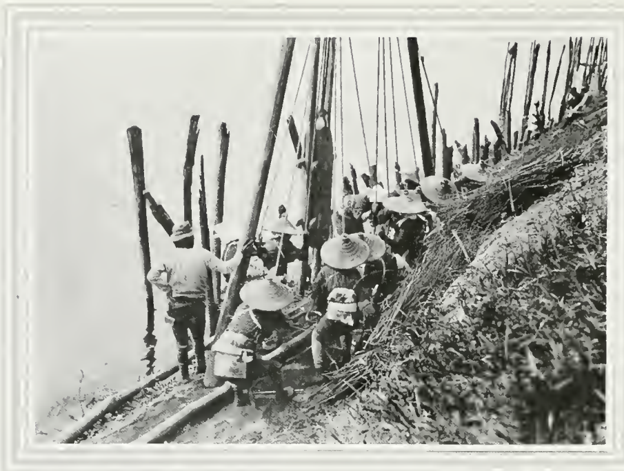
CONSTRUCTING A RIVER EMBANKMENT
