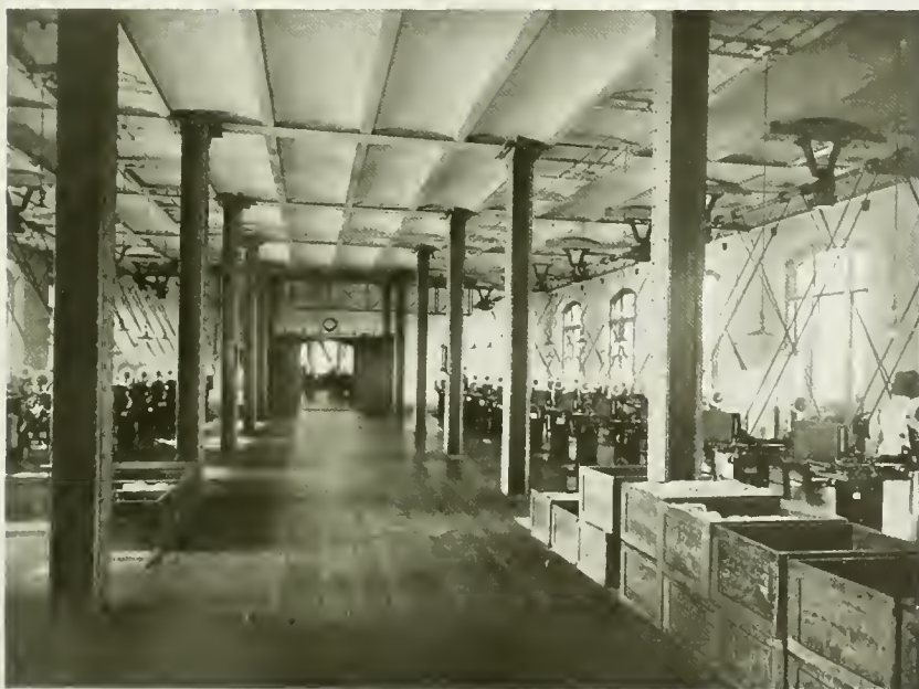
ONE OF THE MACHINE AND WORK ROOMS, IMPERIAL TOBACCO MONOPOLY
