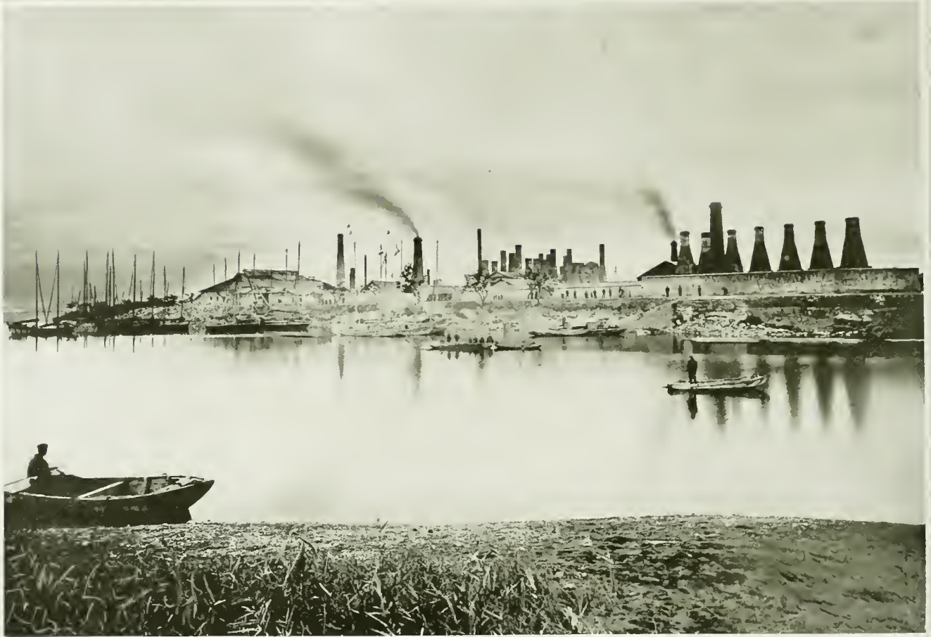
GENERAL VIEW OF FIRST FACTORY OF NIPPON CEMENT CO., LTD.
