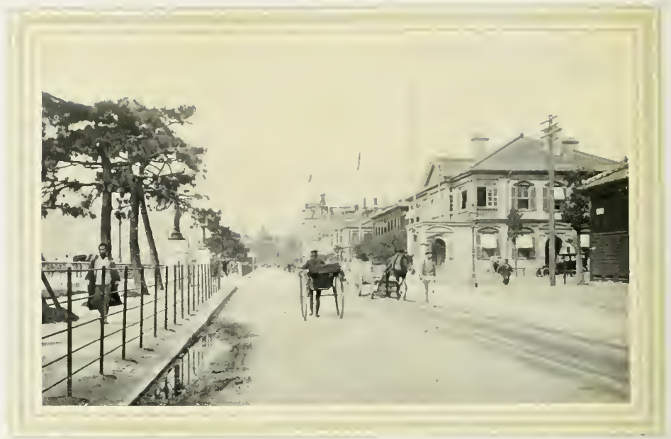
THE BUND, KOBÉ
