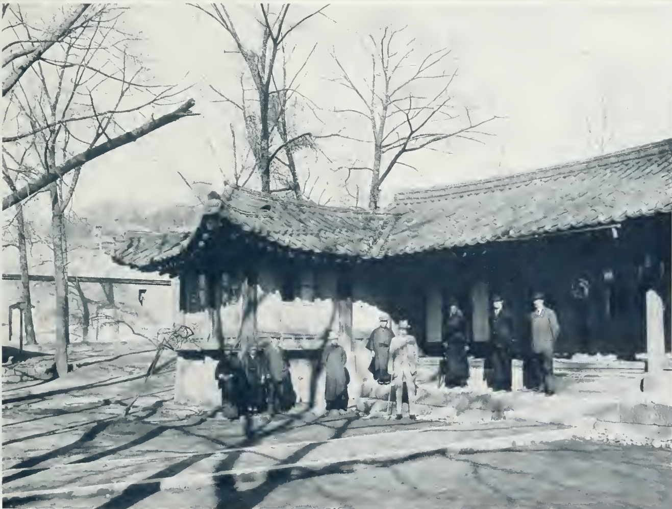
TOWNSEND & COMPANY: THE PICTURESQUE OLD KOREAN OFFICE BUILDING AND THE FIRM'S STAFF
