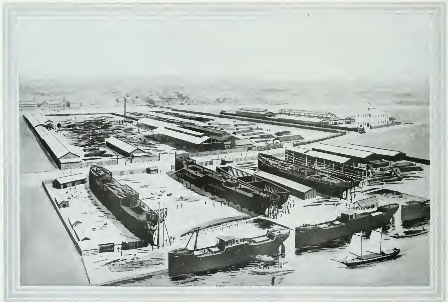
BIRD'S-EYE VIEW OF THE BUILDING YARDS OF THE OSAKA SHIPYARD COMPANY, LIMITED
