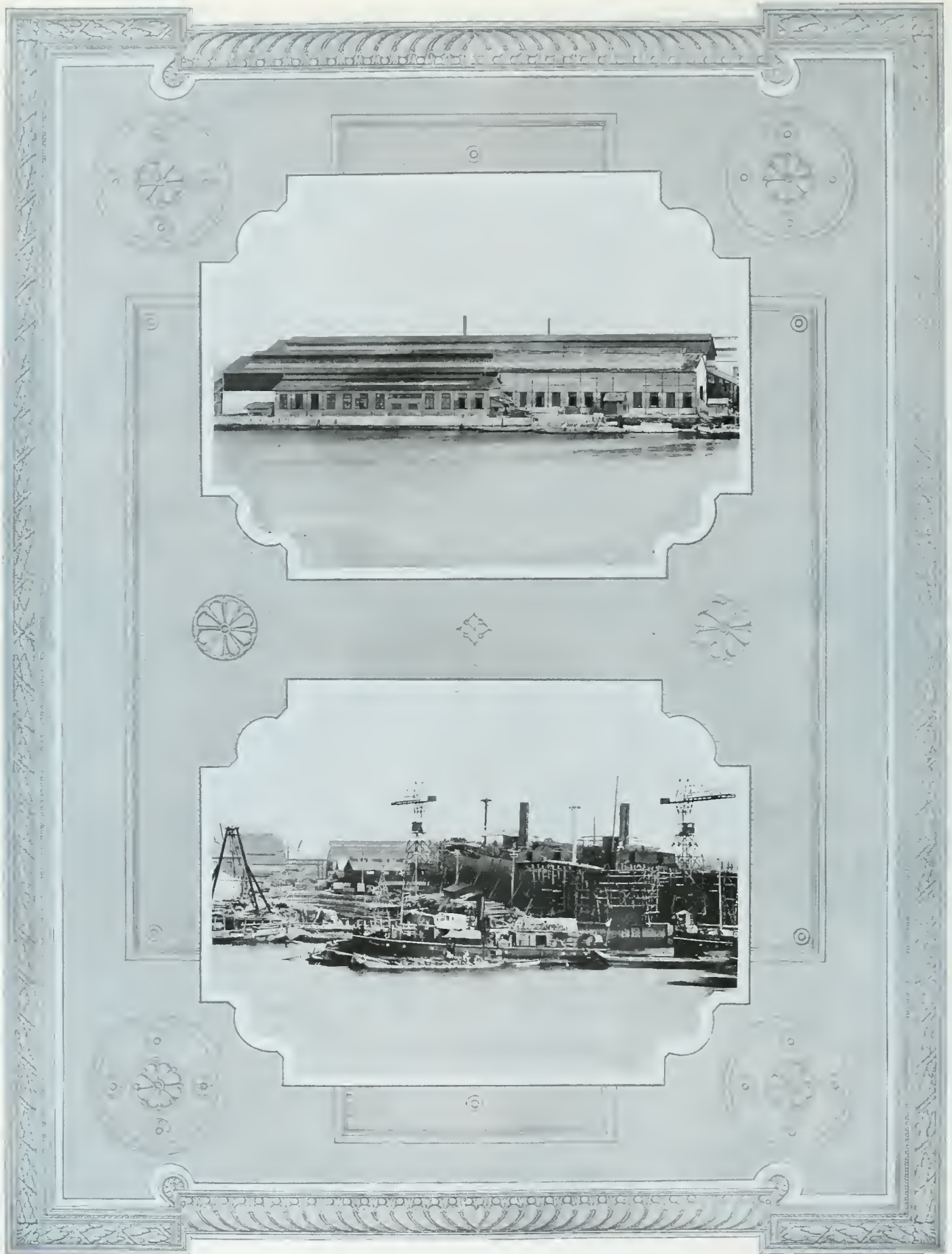
ISHIKAWAJIMA SHIPBUILDING AND ENGINEERING CO., LTD.: THE MACHINE SHOPS AND DOCKYARD
