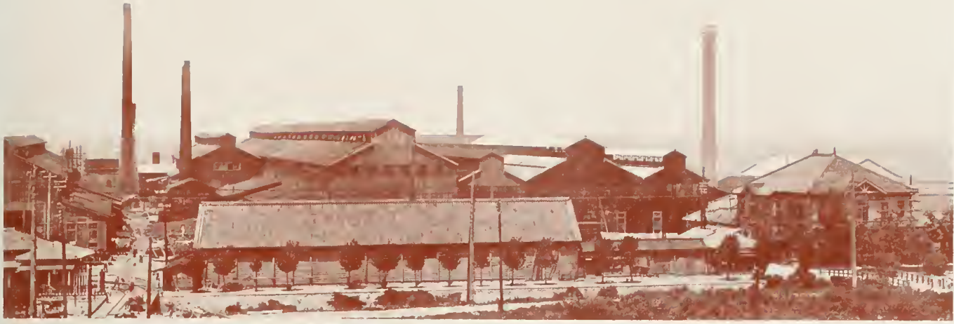
STEEL WORKS AT NISHI-KU, OSAKA
