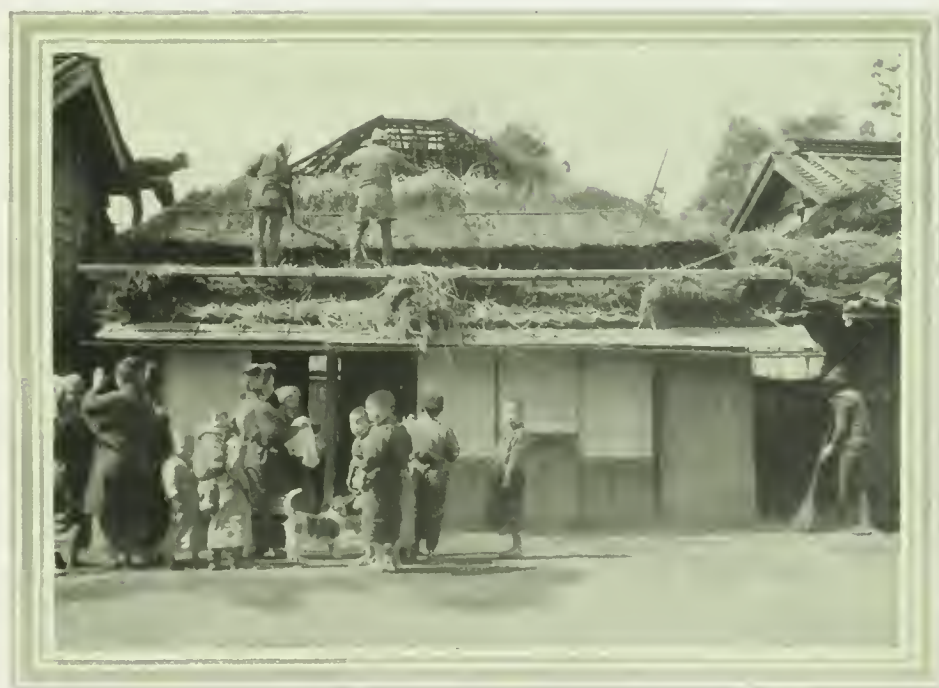
CHANGING THE ROOF, AN OPERATION NECESSARY BUT ONCE IN A GENERATION
