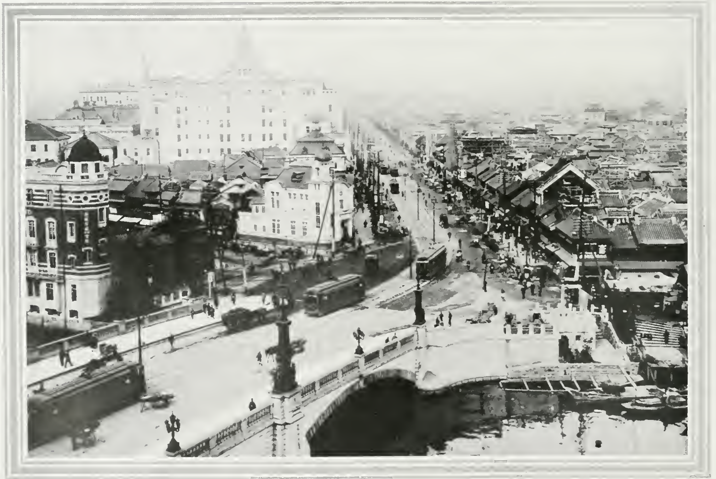
THE NIHONBASHI BRIDGE, TOKYO
