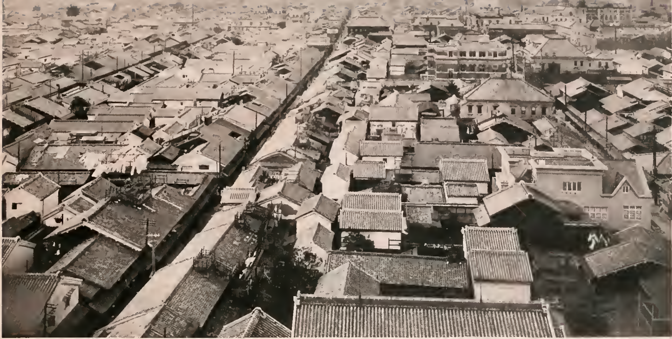
BIRD'S-EYE VIEW OF HIGASHI-KU AND NISHI-KU WARDS, OSAKA
