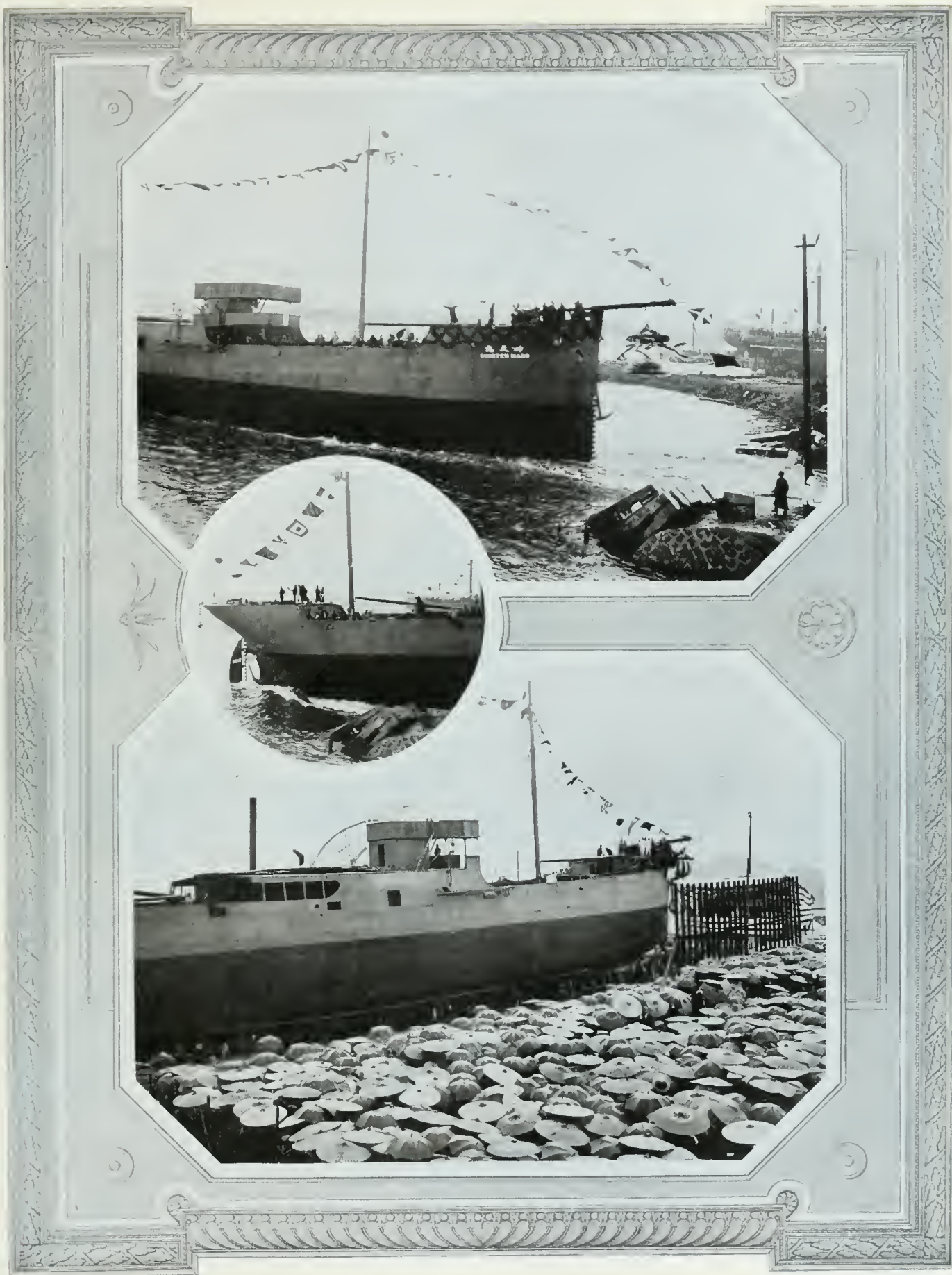
YOKOHAMA DOCK CO., LTD.: THREE VIEWS OF THE LAUNCHING OF THE "SHINTEN MARU"
