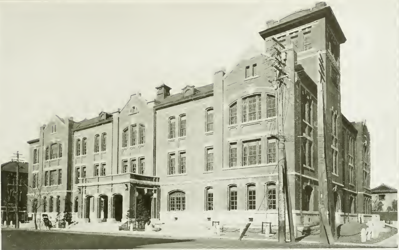
THE ADMINISTRATION OFFICES OF THE IMPERIAL GOVERNMENT MONOPOLIES BUREAU, TOKYO
