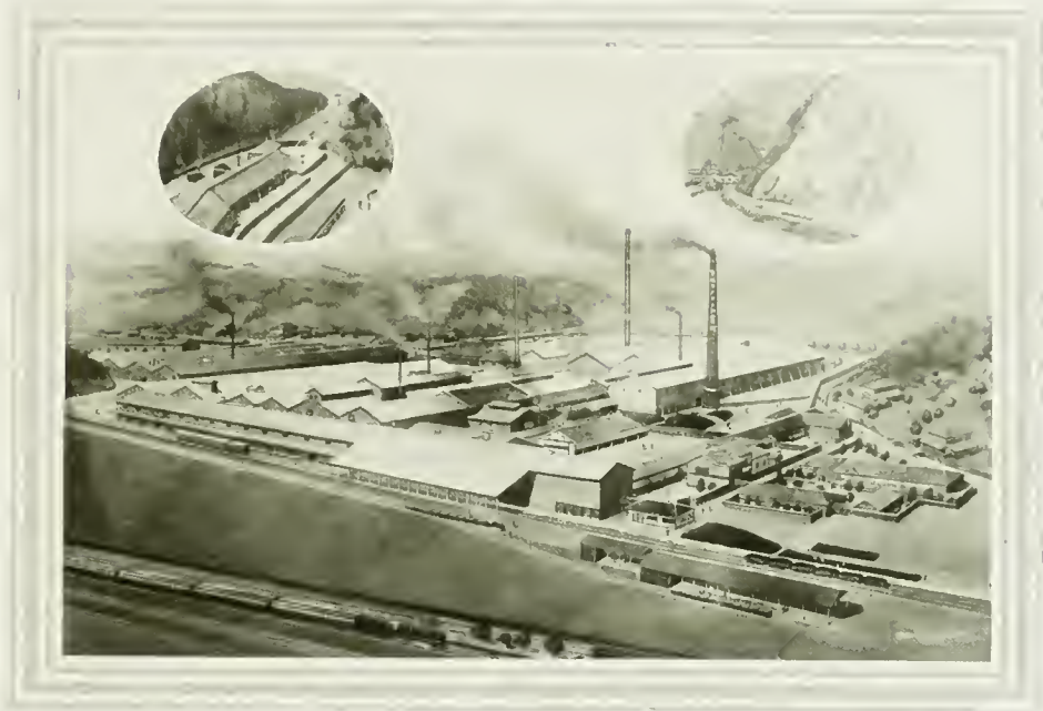
VIEWS OF THE FACTORY OF THE IWAKI CEMENT CO., LTD.
