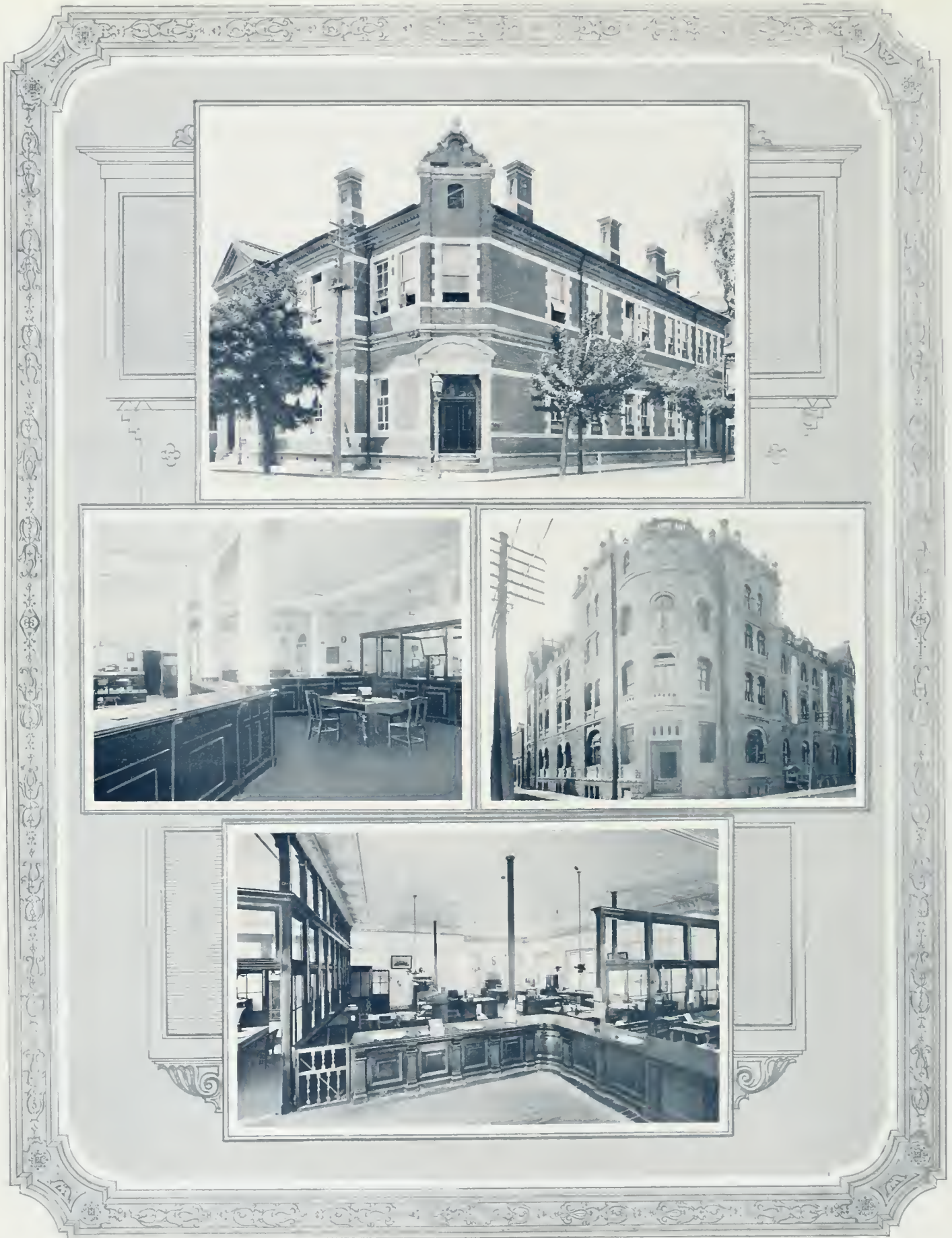
INTERNATIONAL BANKING CORPORATION: KOBÉ BRANCH—INTERIOR OF HEAD OFFICE FOR JAPAN AT YOKOHAMA—BUILDING OCCUPIED BY HEAD OFFICE FOR JAPAN, YOKOHAMA—INTERIOR OF KOBÉ BRANCH
