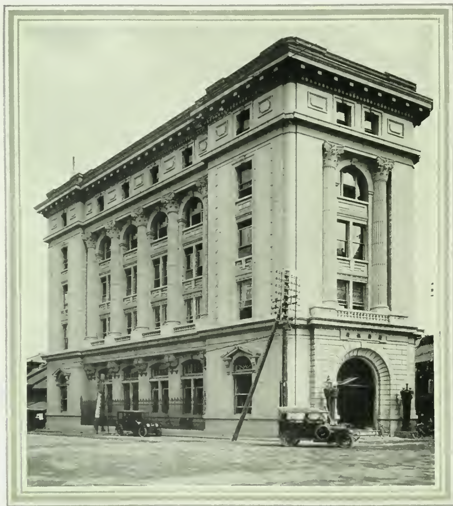
PREMISES OF MEIJI TRADING CO., LTD., LOCATED IN MURAI BUILDING
