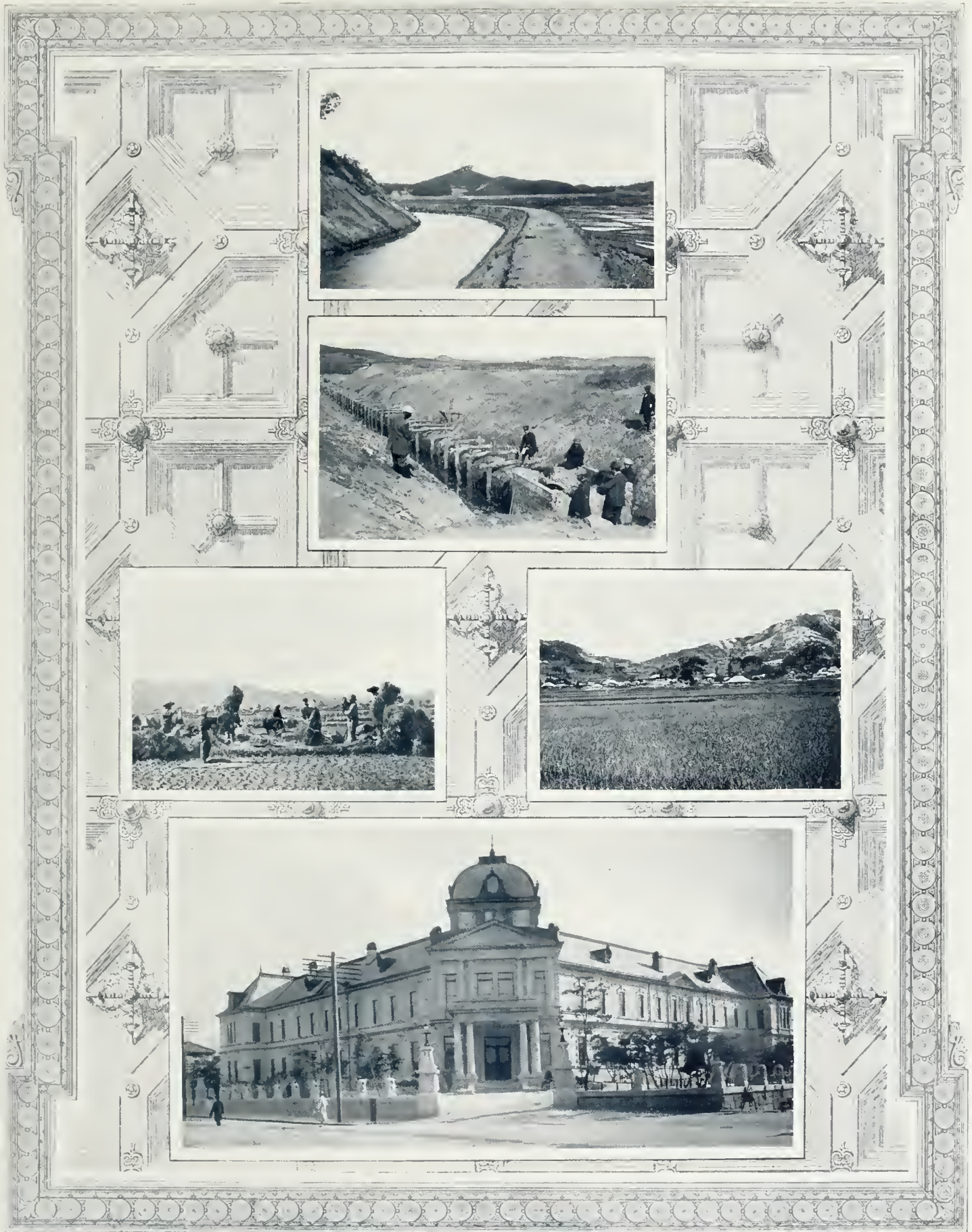
TOYO TAKUSHOKU KABUSHIKI KAISHA (THE ORIENTAL DEVELOPMENT CO., LTD.): VIEW OF FARM LAND AND RICE FIELDS—LAYING AN IRRIGATION PIPE LINE—TWO VIEWS SHOWING TANGIBLE PROOF OF THE COMPANY'S SUCCESS—THE HEAD OFFICE AT SEOUL
