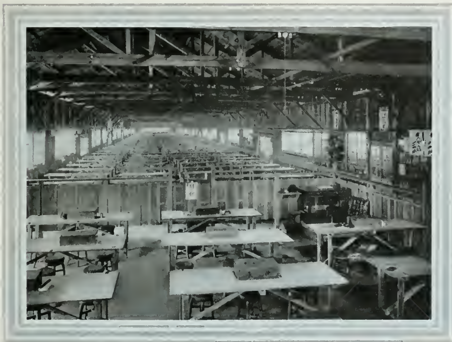
DINING ROOM MAINTAINED FOR THE EMPLOYEES OF THE NIPPON HEIKI SEIZO KABUSHIKI KAISHA (JAPAN ARMS AND MACHINERY MANUFACTURING CO., LTD.)
