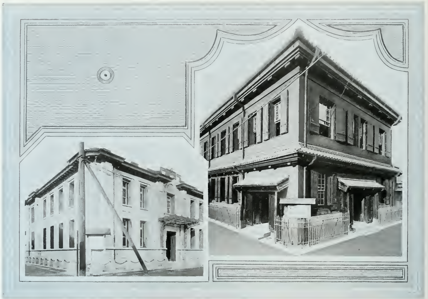
OSAKA CHOCHIKU GINKO (OSAKA SAVINGS BANK, LTD.): THE PREMISES OF THE KYOTO BRANCH — THE HEAD OFFICE AT OSAKA
