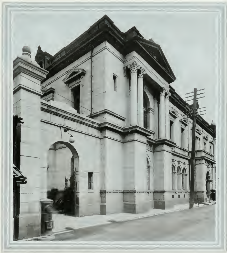
HEAD OFFICE OF THE THIRTY-FOURTH BANK, LIMITED, OSAKA
