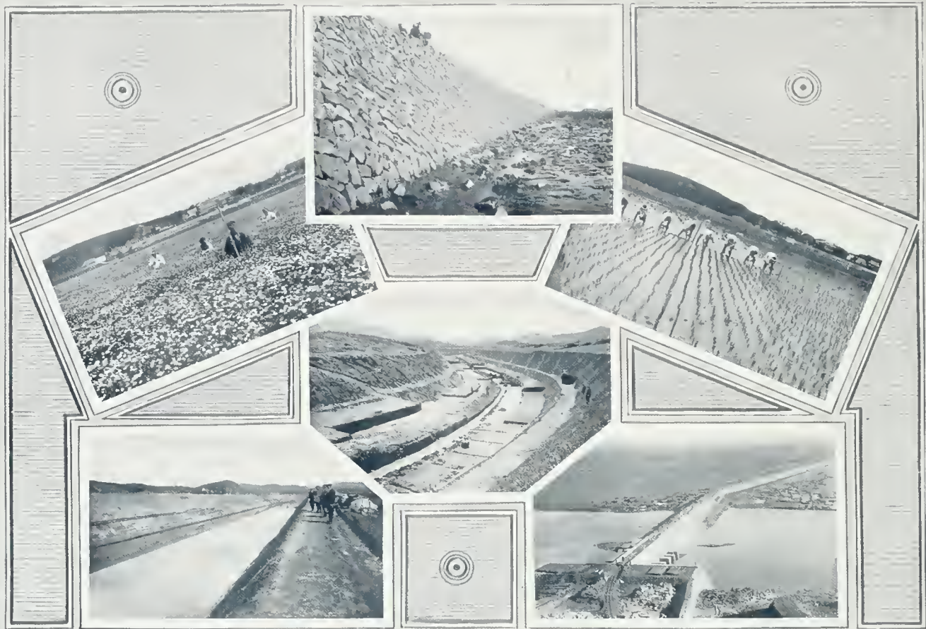
FUJII KOGYO KABUSHIKI KAISHA: (LEFT TO RIGHT) ONE OF THE FIRST CROPS—PORTION OF THE SEA WALL CONSTRUCTED BY THE COMPANY—PLANTING RICE ON REDEEMED LAND. (LOWER CENTRE) CONSTRUCTION WORK ON IRRIGATION CANAL—AN IRRIGATION CANAL—THE SEA WALL
