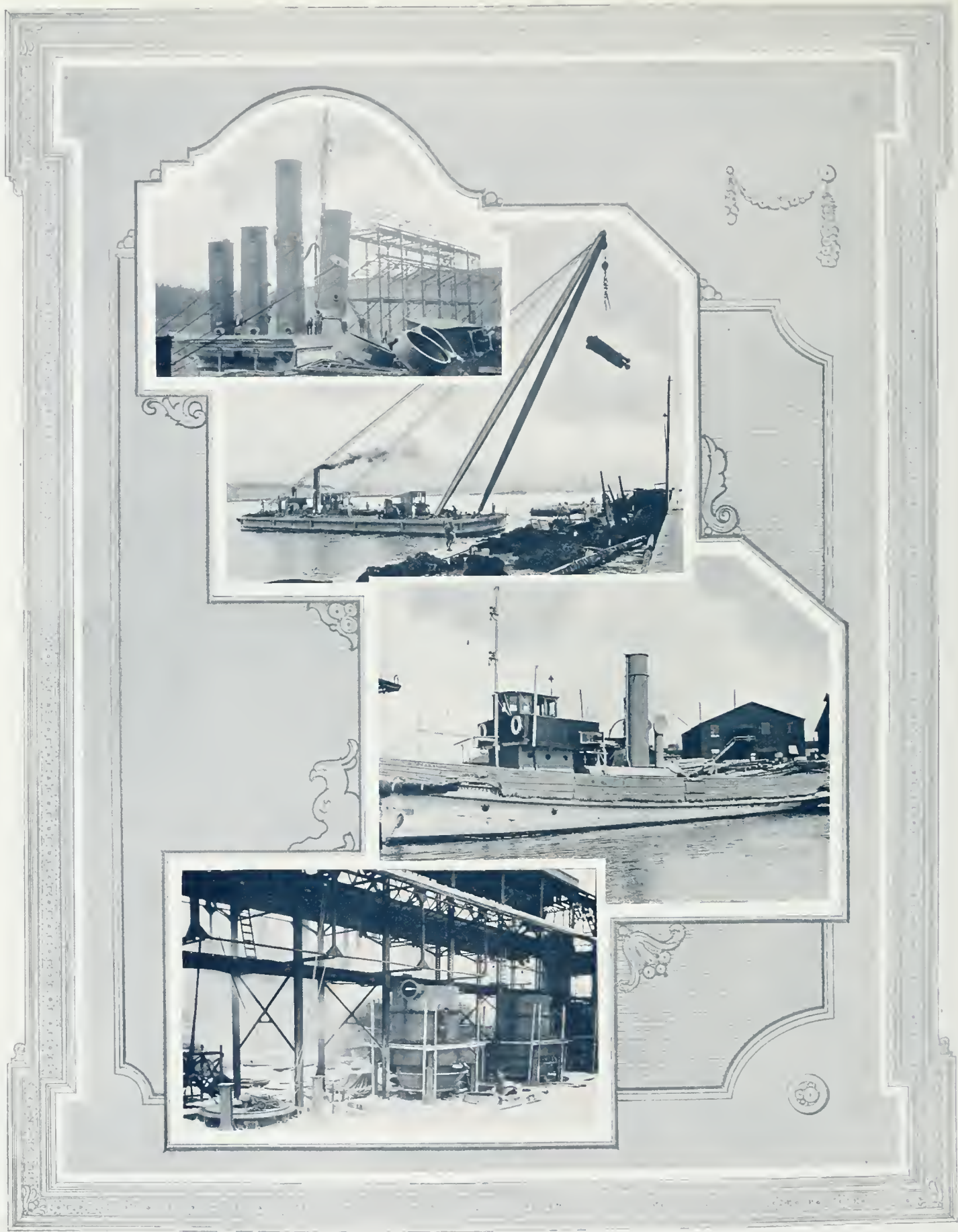
ARTHUR BUCKNEY, A. M. I. E. E. : ERECTION OF LYMN-RILEY GAS PRODUCERS — TYPE OF FLOATING CRANE SUPPLIED TO THE RUSSIAN GOVERNMENT —TYPE OF TUG BOAT SUPPLIED TO THE RUSSIAN GOVERNMENT—ANOTHER PROCESS IN THE ERECTION OF LYMN-RILEY GAS PRODUCERS
