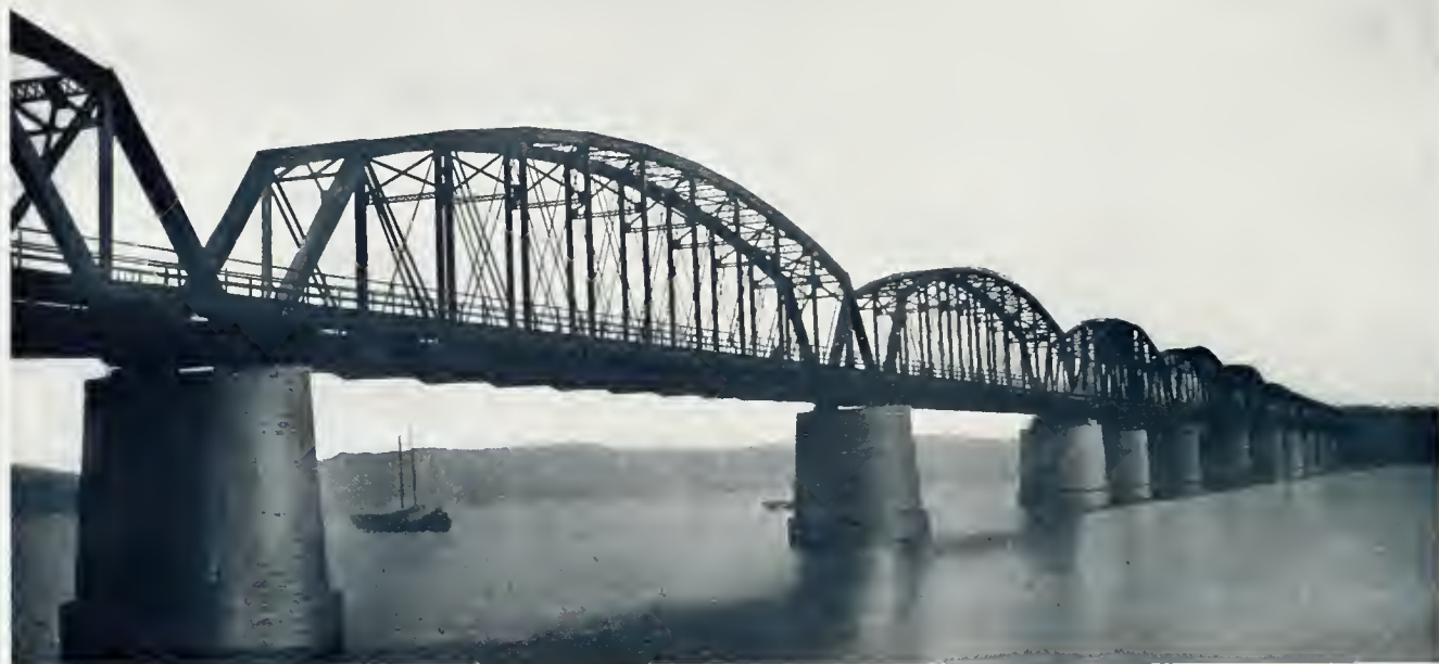
THE RAILWAY BRIDGE OVER THE YALU RIVER AT ANTUNG, 3,098 FEET IN LENGTH
