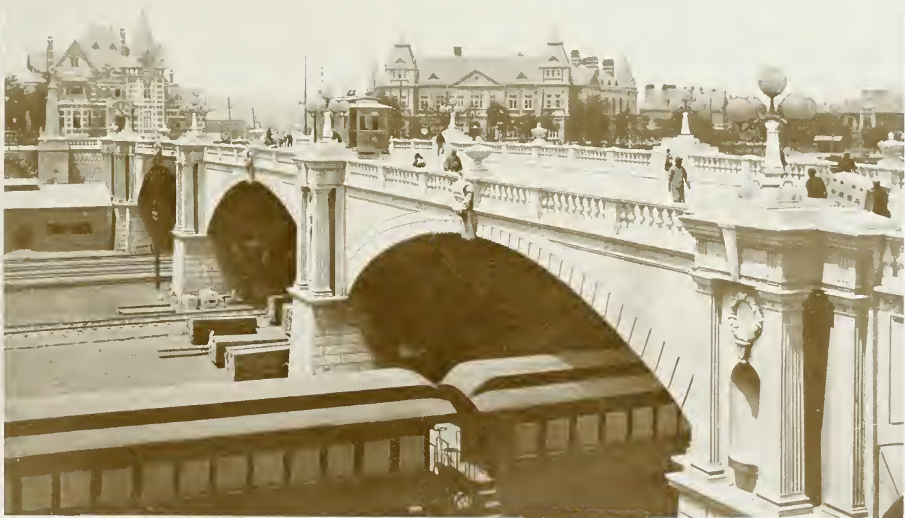
NIPPON BRIDGE OVER SOUTH MANCHURIA RAILWAY, DAIREN
