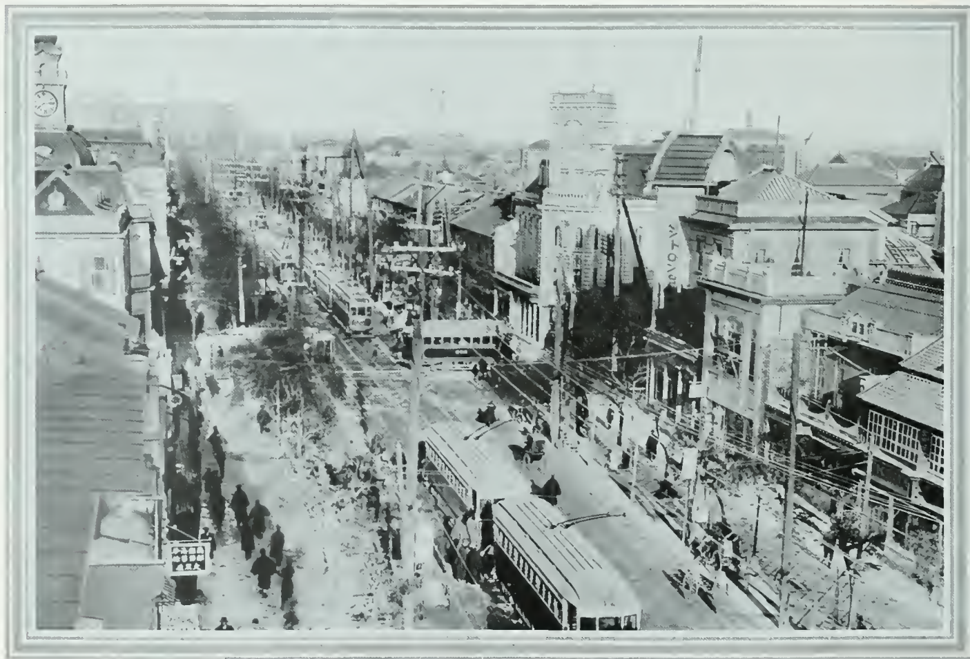
GENERAL VIEW OF BUSINESS STREET IN TOKYO
