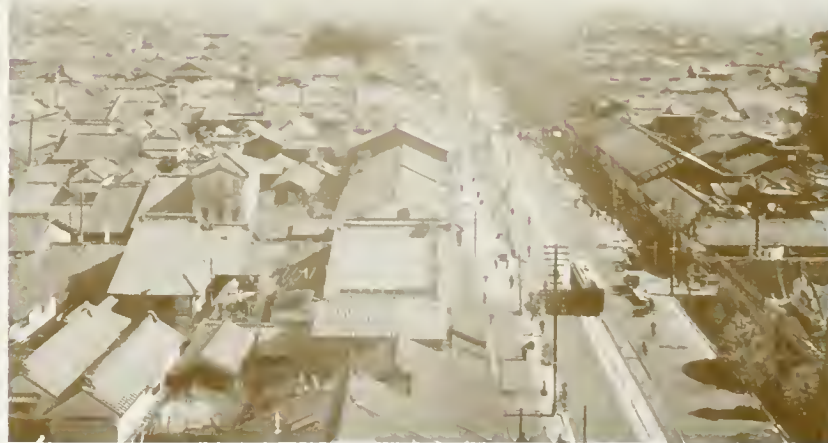
LOOKING TOWARD THE MONUMENT FROM THE ROOF OF FUJIMOTO BILLBROKER BANK, NAGOYA
