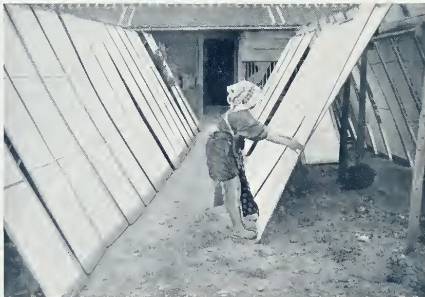
METHOD OF SUN-DRYING PAPER EMPLOYED IN A SMALL FACTORY
