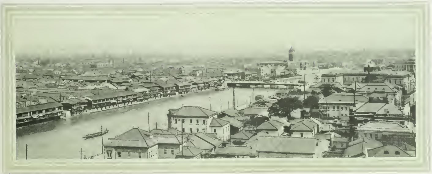
A VIEW OF KITA WARD, SHOWING WATANABE BRIDGE. PROMINENT IN THE PICTURE IS THE SUPREME COURT BUILDING
