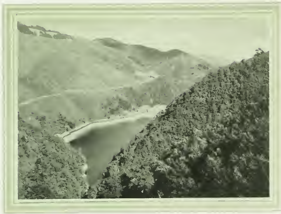
RESERVOIR AT KOBÉ
