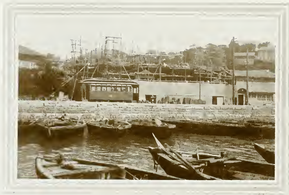
SAWAYAMA SHOKAI: NEW NAGASAKI PREMISES IN COURSE OF CONSTRUCTION
