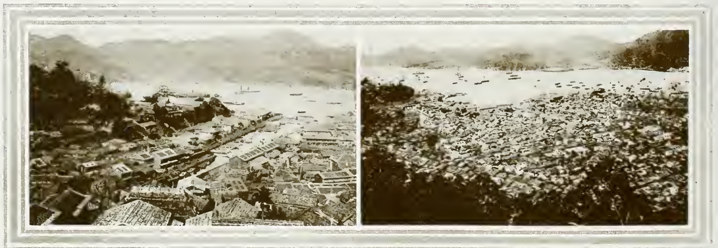
TWO ASPECTS OF THE PORT AND HARBOUR OF NAGASAKI
