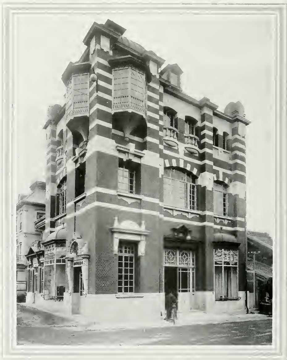
PREMISES OF TAKEUCHI SAFE COMPANY
