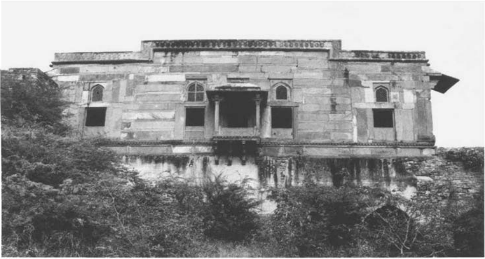
Plate 30. Akbar's jharoka , exterior facade, Daftar Khana, Fatehpur Sikri
