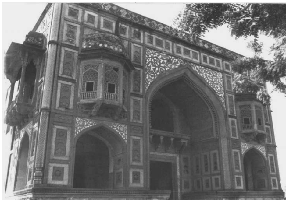
Plate 81. Partial facade, Kanch Mahal, Agra
