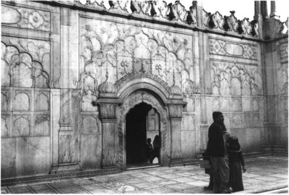
Plate 161. Courtyard walls, Moti mosque, Shahjahanabad, Delhi
