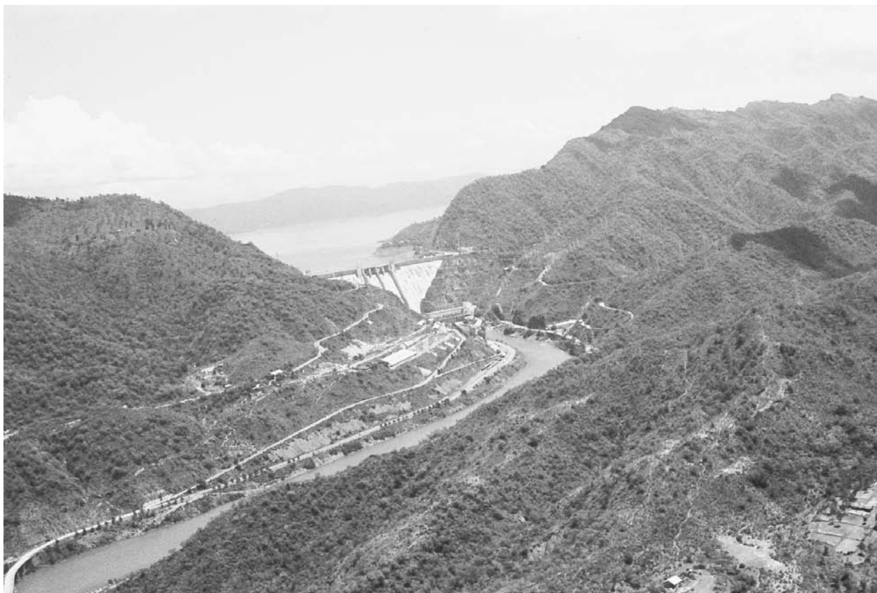
Bhakra Dam. When Nehru dedicated the Bhakra Dam (shown here) in 1963, he referred to it as a “temple of modern India,” a symbol of the aspirations of developing countries worldwide. In the early twenty-first century, similar large-scale dam projects in India (at last count more than 23) are the focal point of several well-funded campaigns to protect the millions of ordinary citizens displaced by them. SUJATA KULSHRESHTHA / FOTOMEDIA.
