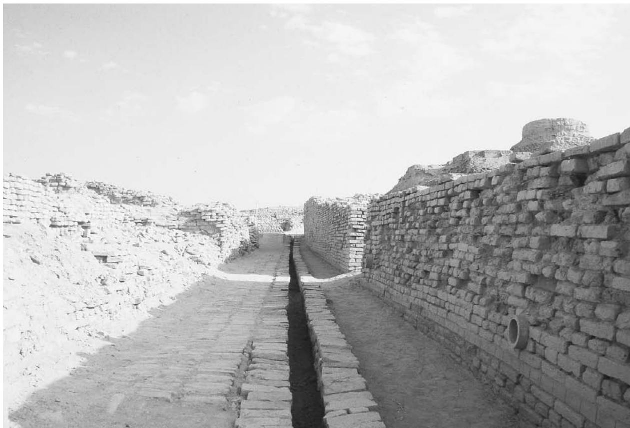
Brick Wall and Drain Excavated at Mohenjo-Daro. Due to the nature of the topography and the intensity of floods along the Indus and its tributaries, ancient settlements were not able to maintain major canals for irrigation, although they frequently constructed drains for redirecting floodwaters. FOTOMEDIA ARCHIVE.
