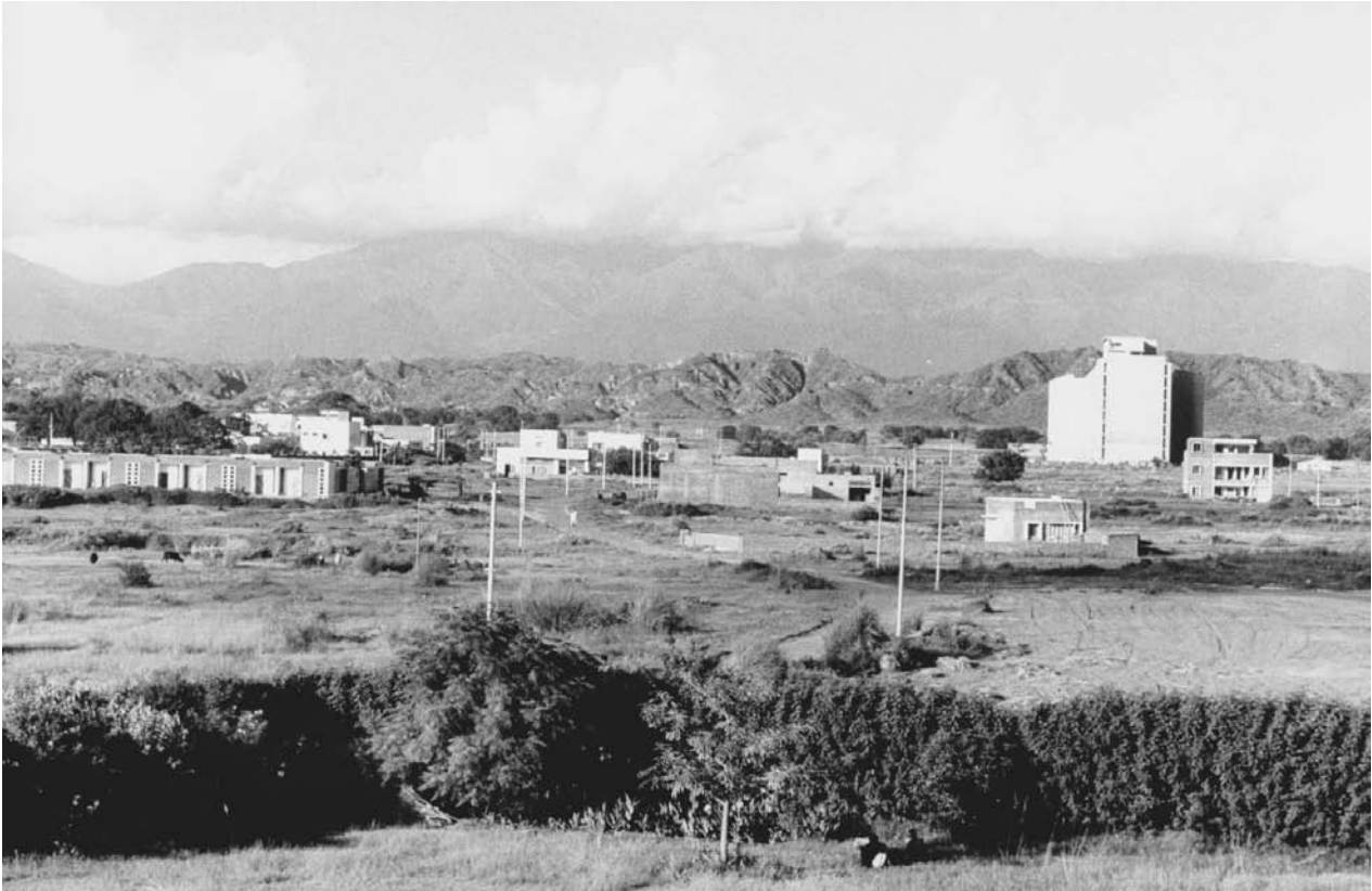
Secretariat Building in Chandigarh. To the right, the Secretariat, one of a series of government buildings on the northern fringe of Chandigarh designed by Le Corbusier, the French modernist architect, in the 1950s. The buildings' monumental size and scale were consonant with both the aspirations of Prime Minister Nehru who was eager for symbols of greatness for the new capital, and the splendid Himalayan landscape in which they are set. TIME LIFE PICTURES/GETTY IMAGES.
