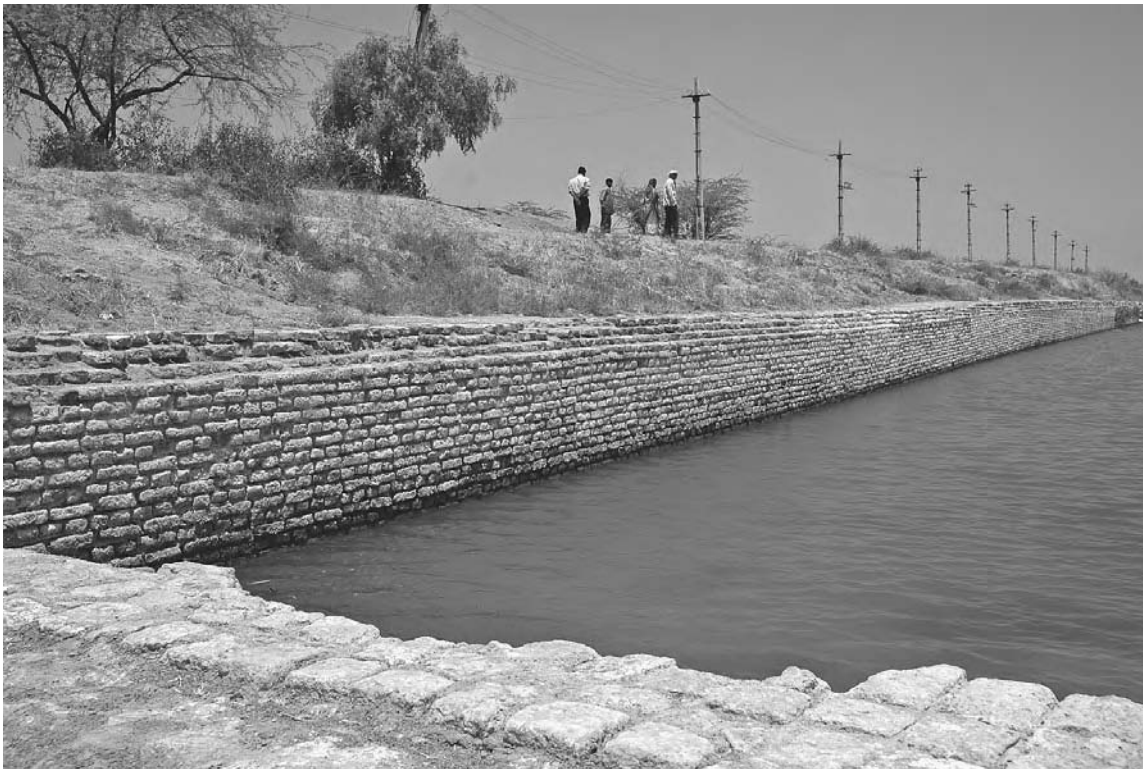
A view of the basin at Lothal, commonly known as the dock. It undoubtedly held water, probably seawater given that marine shells have been found in it; it had an inlet channel linking it with the river flowing past the settlement and an outlet channel with a sluice gate. Little else can be said about it with certainty and its purpose has yet to be convincingly established. (Namit Arora)
