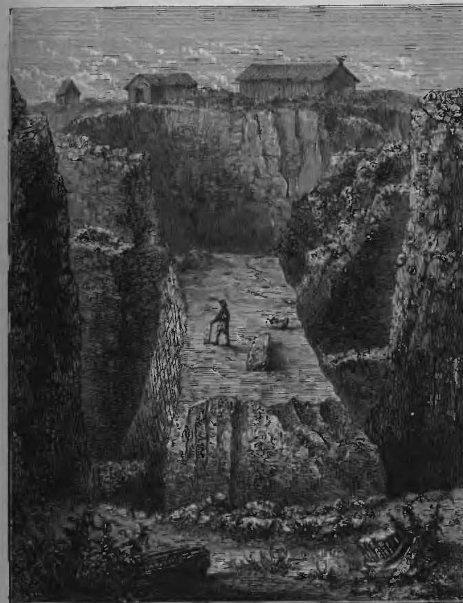
No. 3. The Great Tower of Ilum, seen from the S.E. The top is 8 m. (26 ft.) below the surface of the hill; the foundation is on the rock, 14 m. (46½ ft.) deep: the height of the Tower is 20 ft.
