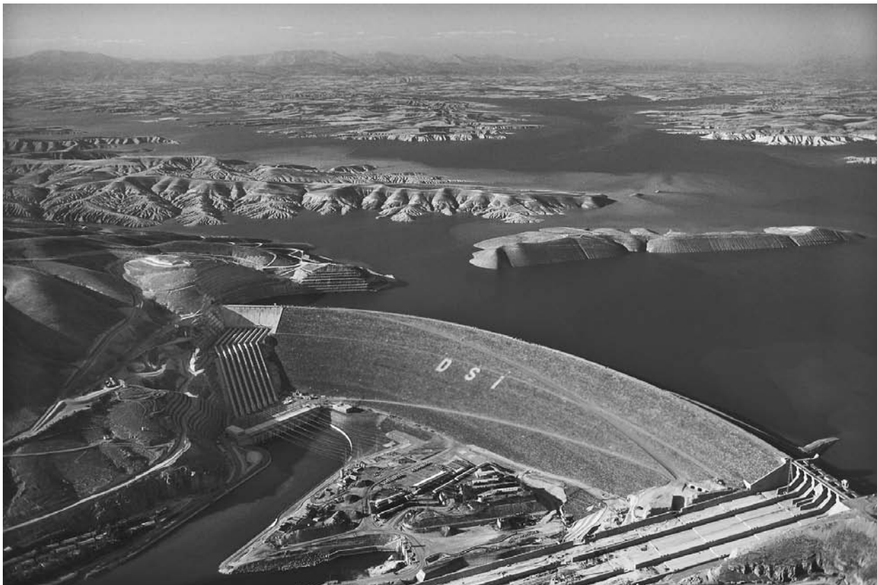
Atatürk Dam , built across the Euphrates River in southeastern Turkey and in use since 1990, is one of the largest dams of its kind (earth and rock fill) in the world. Dams such as these are not only expensive but are also costly in terms of reducing the flow of water to countries lying downstream, contributing to a growing shortage of fresh water in much of the region. © ED KASHI/CORBIS. REPRODUCED BY PERMISSION.
