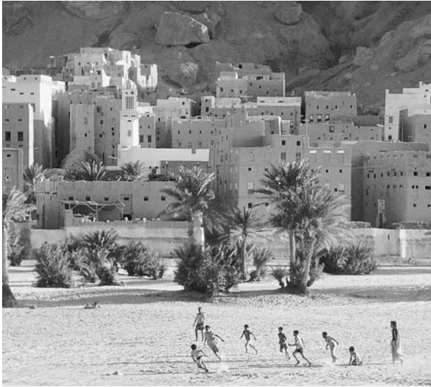
View of Shibam, Yemen, in the desert valley of Hadramawt. Hundreds of ancient, tower-like houses of up to nine stories high and built from clay can be seen from far away. UNESCO has declared it a protected world monument. © EARL & NAZIMA KOWALL/CORBIS. REPRODUCED BY PERMISSION.
