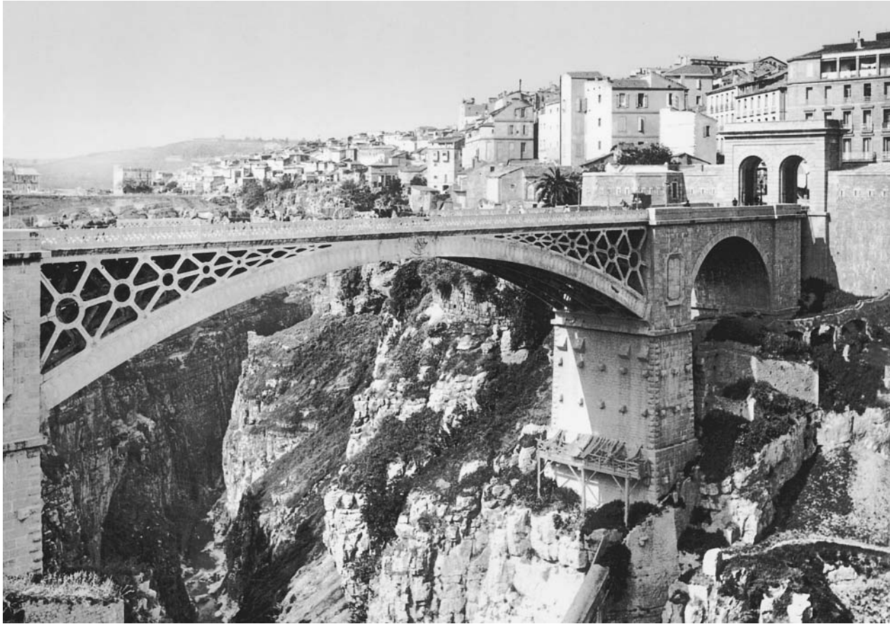
A leading producer of leather, woolen, and linen goods, Constantine is the largest city in eastern Algeria and the oldest continually inhabited city in the country. Constantine is almost completely surrounded by the Rhumel Gorges, and access to the city is provided by several spectacular bridges. LIBRARY OF CONGRESS PRINTS AND PHOTOGRAPHS DIVISION WASHINGTON, D.C.
