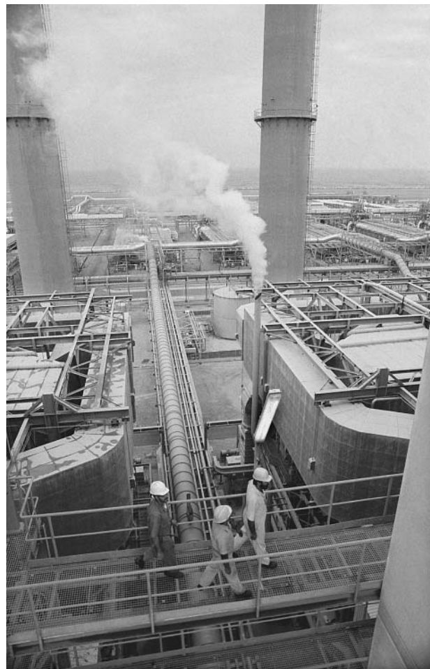
The desalinization plant at Jubail, Saudi Arabia, was the largest such facility in the world when it was photographed for the first time by foreign news media, in 1991. One of several plants along the Persian (Arabian) Gulf, between Kuwait and Qatar, it was then capable of processing 230 million imperial gallons of seawater into drinking water per day. © BETTMANN/CORBIS. REPRODUCED BY PERMISSION.
