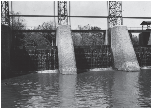
Solving the problems of getting water to the growing cane: Elaborate irrigation works in the sugar belt along the north coast of Central Java, 1920s (KITLV 18384, 18376, 18385)
