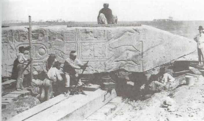
Photograph showing 'Cleopatra's needle' in the process of being prepared for transportation by the British engineer James Dixon. The obelisk was placed in a specially-made metal cylinder, towed by boat to England, and eventually erected on the Thames Embankment in 1878, only a year after Dixon had been contracted to bring it from Egypt. (REPRODUCED COURTESY OF THE GRIFFITH INSTITUTE)
