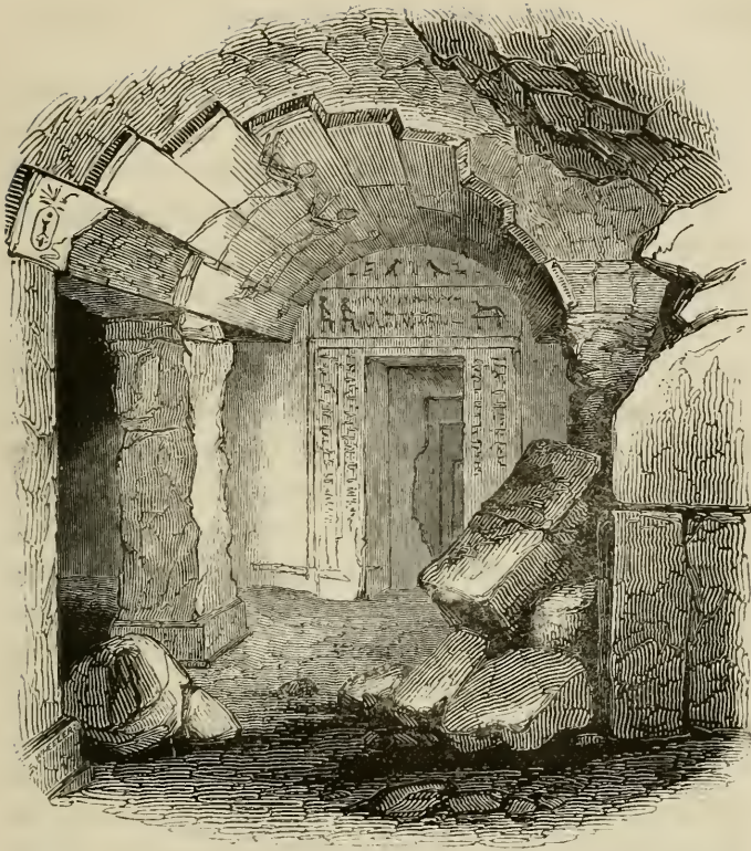
Vignette I. — Tomb at Saqqara, arched with stone, of the time of Psamaticus II. whose name occurs on the roof to the left, and other places.
